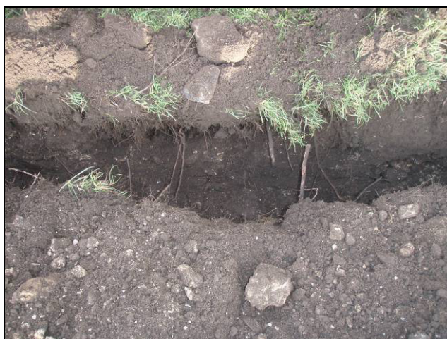
Fig. 4 South facing section of Green Lane duct trench
