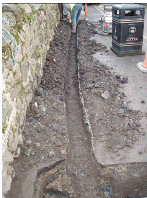
Fig. 8 Service box and ducting trench on Chare End
