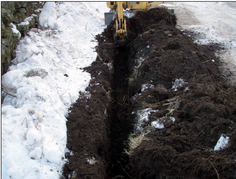
Fig. 3 Trench cut for ducting
