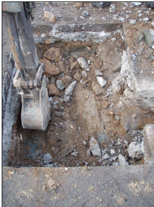
Fig. 4 Service box trench
