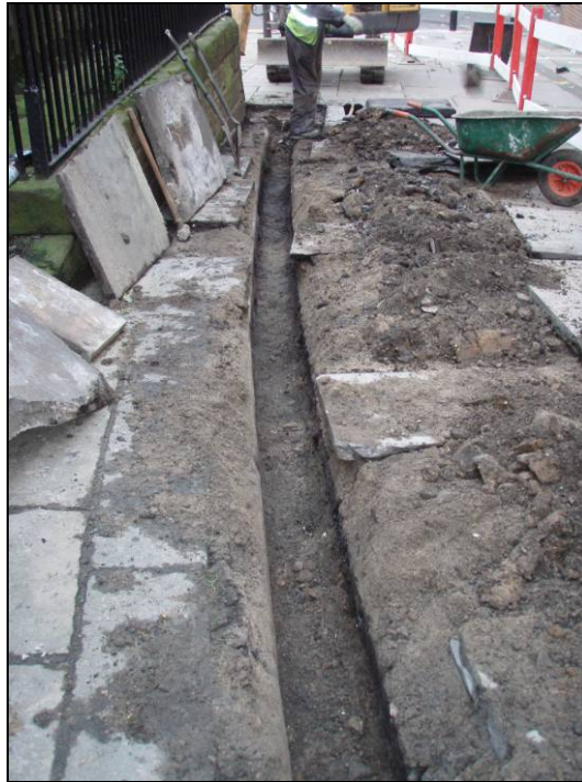
Fig. 3 Ducting trench on Croft Street looking south
