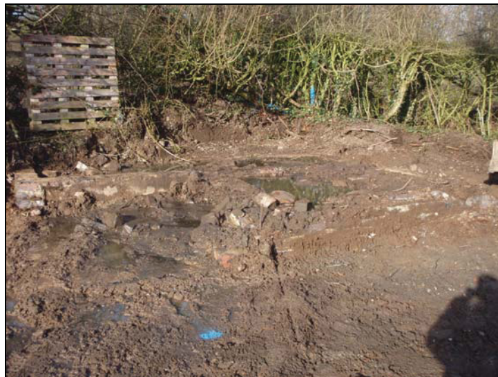
Fig. 6 View of the demolished brick built building.
