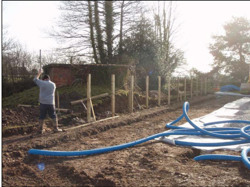
Fig. 7 Excavation of fence posts.
