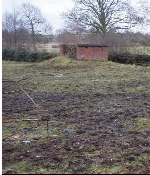
Fig. 5 View of the brick built building.
