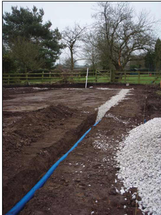
Fig. 4 View of a drainage trench being backfilled.
