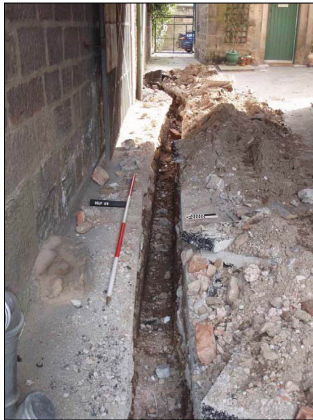
Fig. 3 Trench shown running below the archway, looking east. (Scale: 2m)
