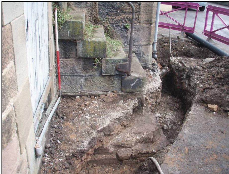
Fig. 7 View of sandstone foundation corner (106) showing the proximity to the steps and building above (Scale: 2m)
