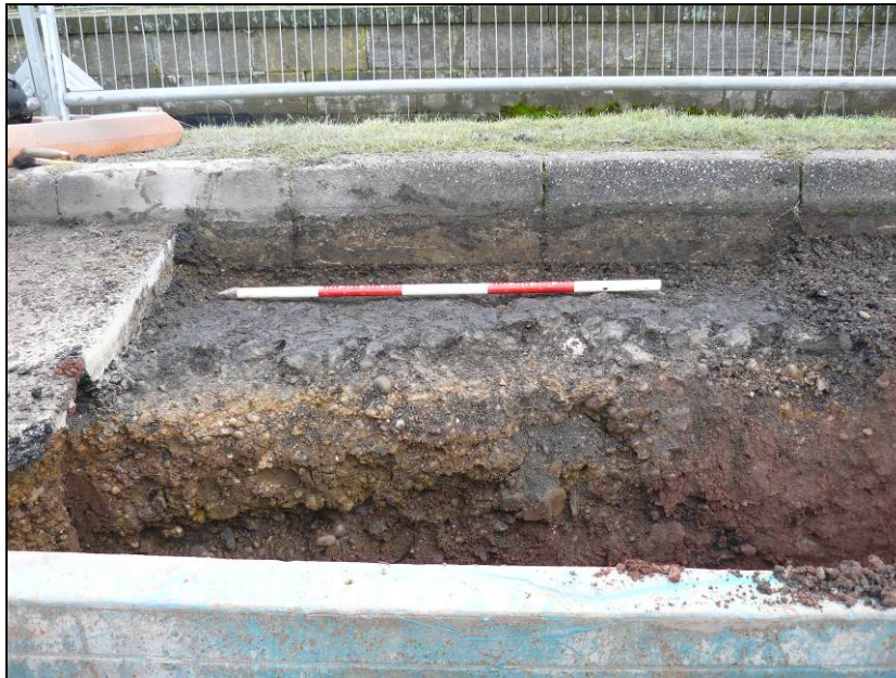
Fig. 11: View of gravel surface (507) below tarmac in Trench 3, Scale: 2m (looking east).
