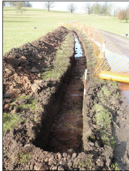
Fig. 18: Trench 4, looking west. (Scale: 0.2m graduations)
