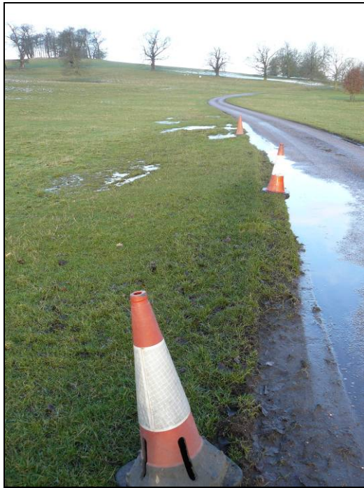
Fig. 17: View of flooded access road.
