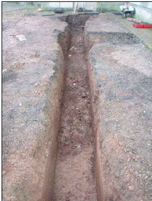
Fig. 13: Trench 3: View of trench, (looking south).
