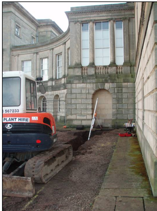
Fig. 12: Location of Trench 3 (looking south).
