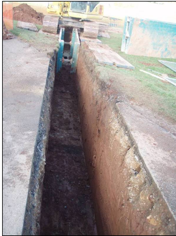
Fig. 7: View of Trench two coming across the road.
