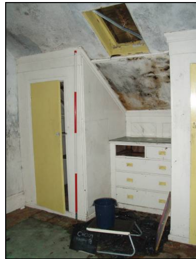
Fig. 42 Modern cupboards in Room 9.
