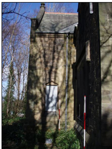
Fig. 21 External south elevation, west section.
