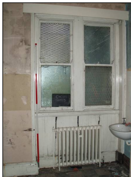
Fig. 36 Sash windows of Room 5
