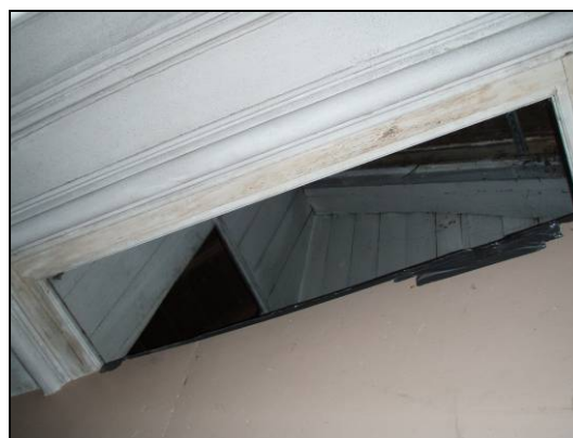
Fig. 48 Partition wall blocking Light in Room 14.
