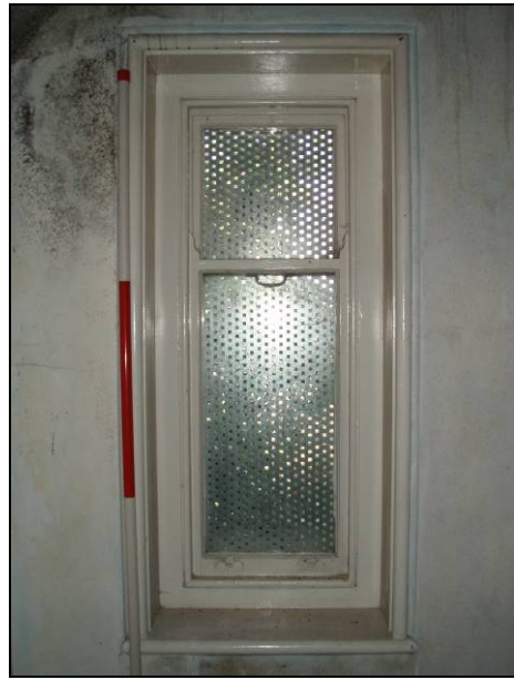
Fig. 40 Small sash window in Room 8.
