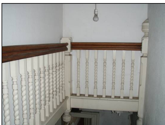
Fig. 49 Partition wall behind balustrade in Room 14.
