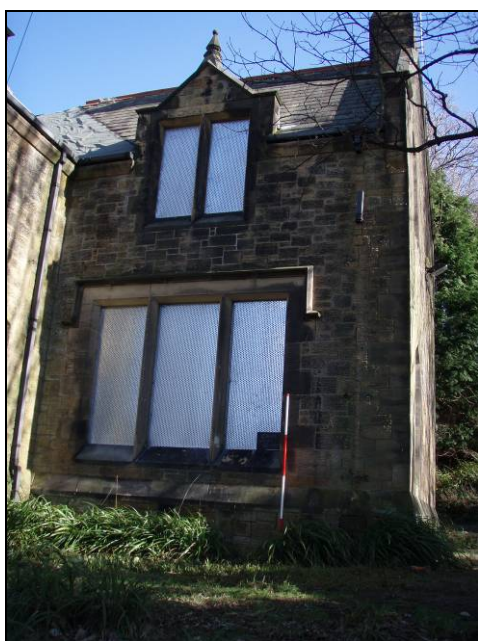
Fig. 16 Exterior west elevation, south section.
