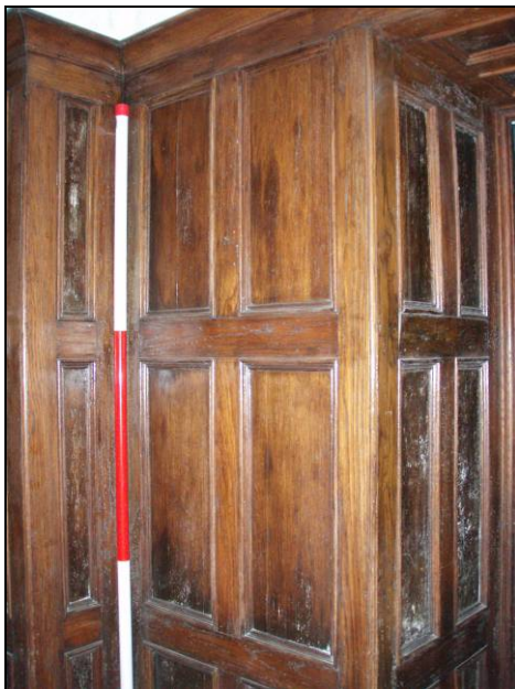
Fig. 27 Wood panelling in porch.
