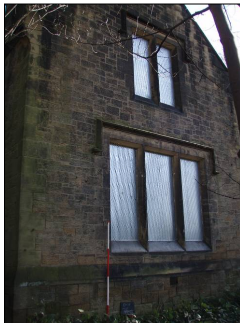
Fig. 17 Exterior west elevation central.
