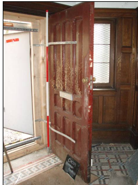
Fig. 26 Internal porch doorway.
