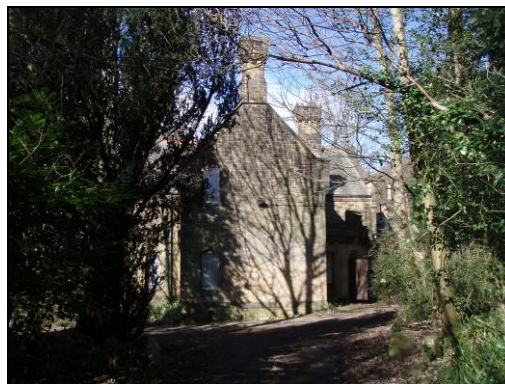
Fig. 20 Exterior south elevation, central section
