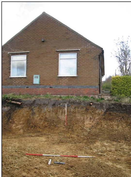
Photo showing made-ground deposit located to the north & underlying the property.
