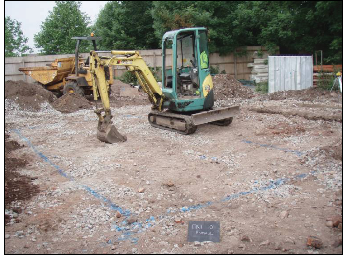
View of phase two excavation area. Facing south.
