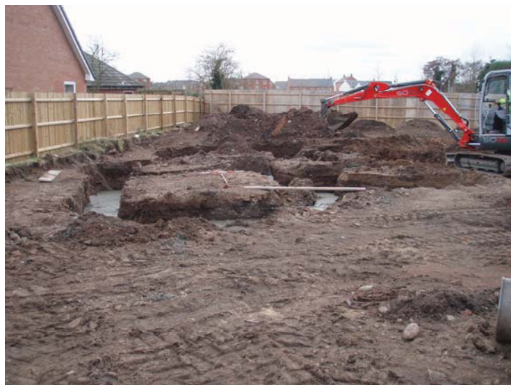
View of the foundation trenches after excavation facing south
