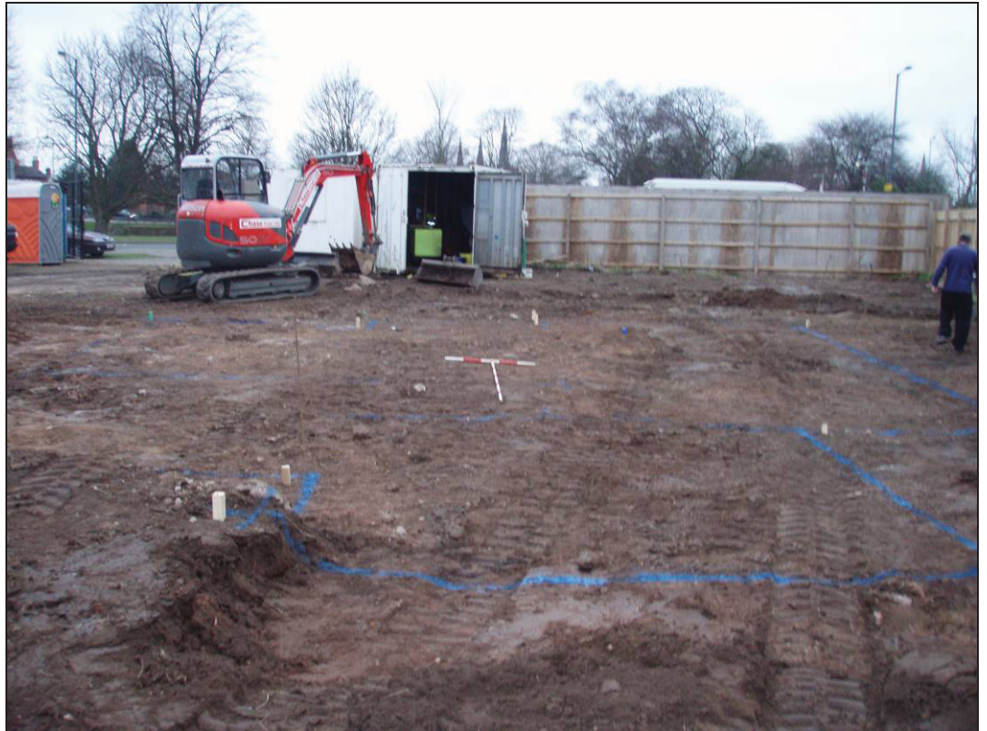
Figure 3. Stripped area prior to excavation of foundation footings
