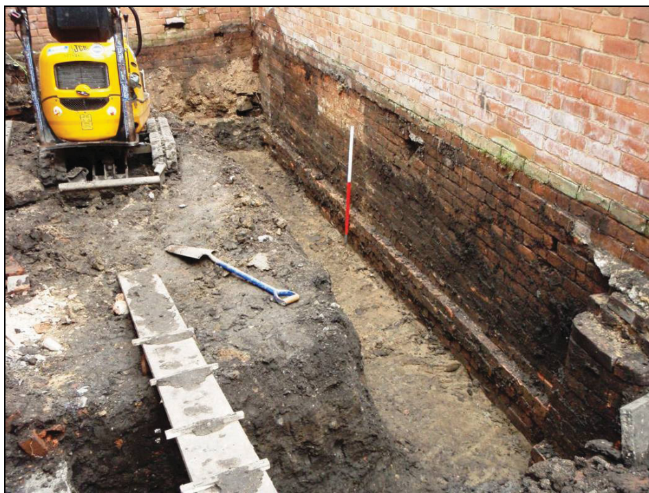
Figure 10: Foundation trench fully excavated down to the natural sub-stratum (117)
