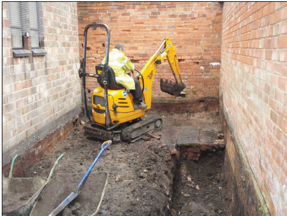
Figure 8: Foundation trench along garden wall, looking north
