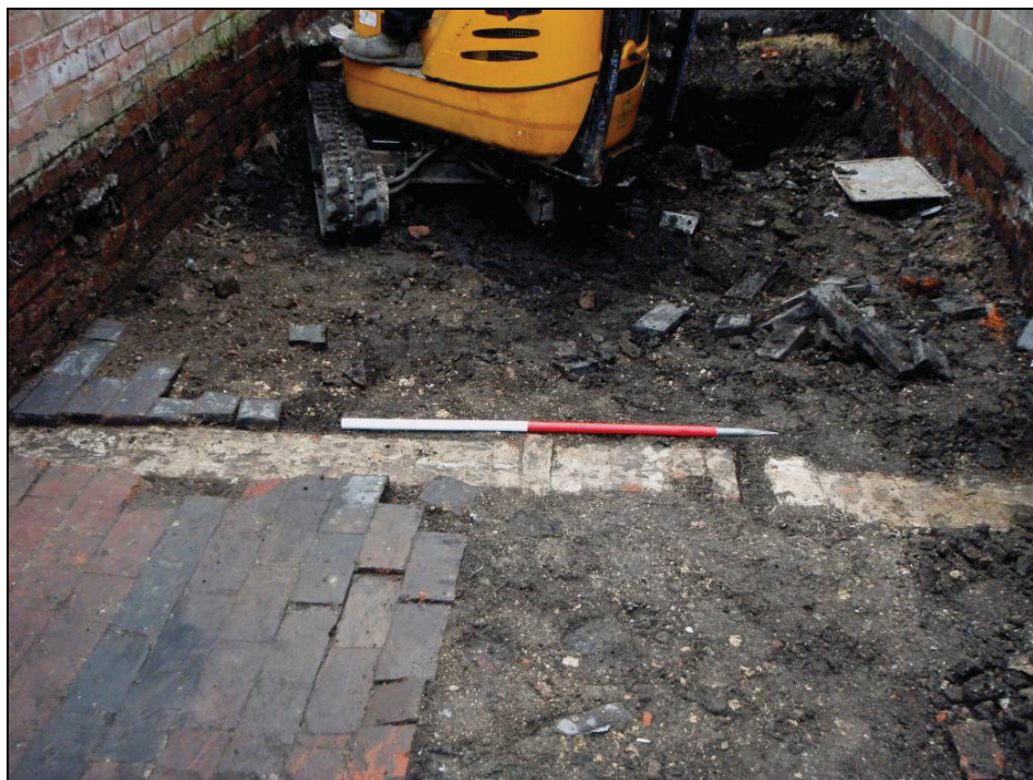
Figure 6: E/W brick wall (110), looking south
