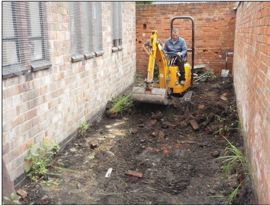
Figure 3: Excavation of drain trench, looking east
