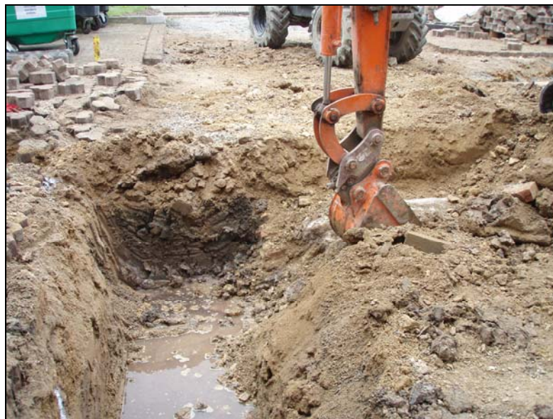
Fig. 4 Area 2 excavation showing course of brick lined drain.
