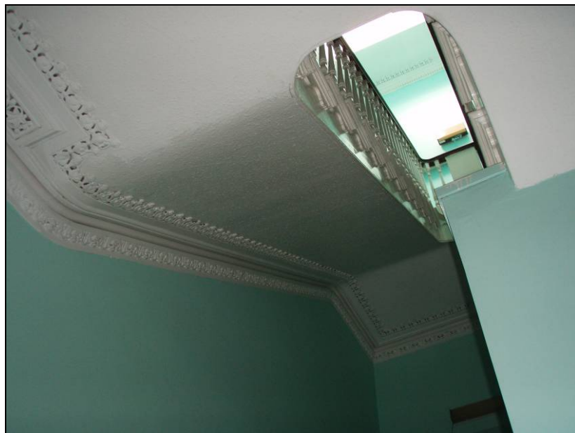
Fig. 21 Ceiling coving above staircase
