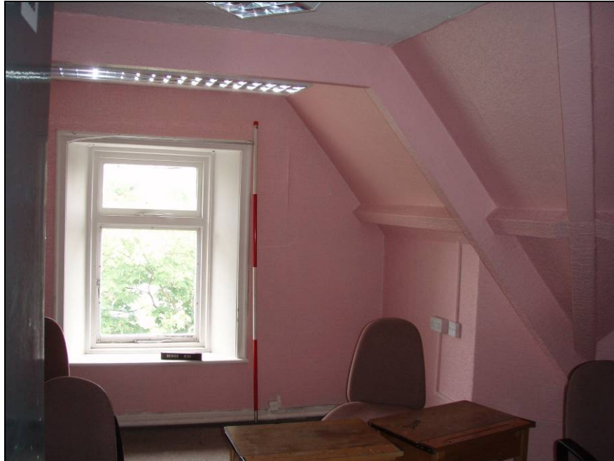
Fig. 22 Roof beams in room 30
