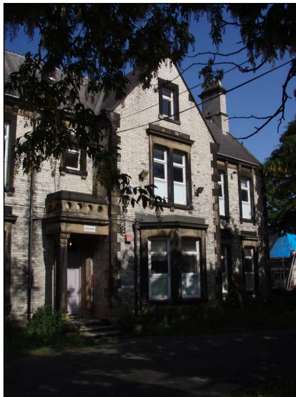
Fig. 11 East facing elevation
