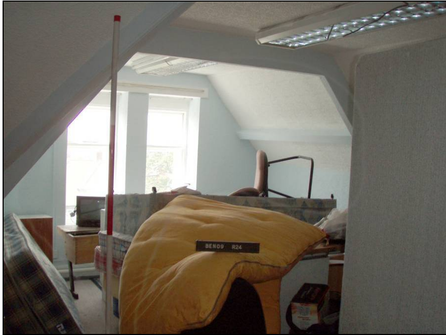
Fig. 21 Roof beams in room 24
