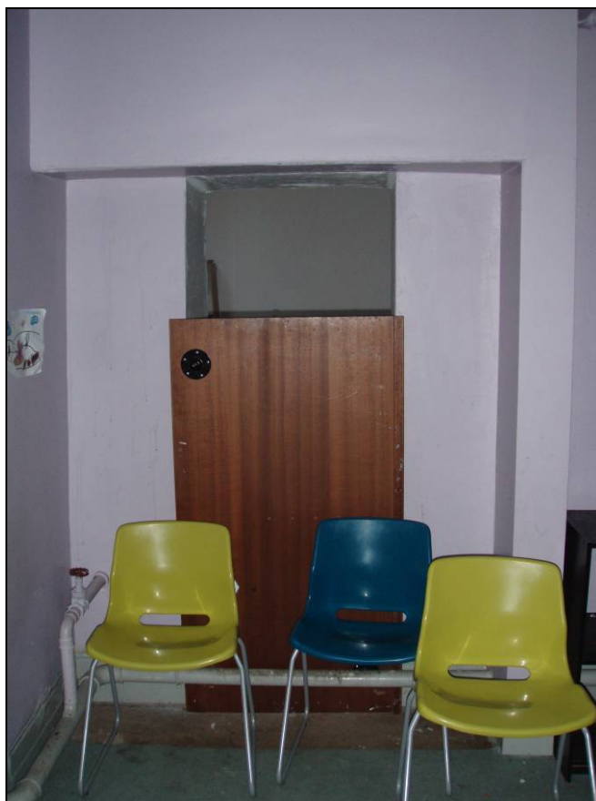
Fig. 17 Internal partition opening room 4
