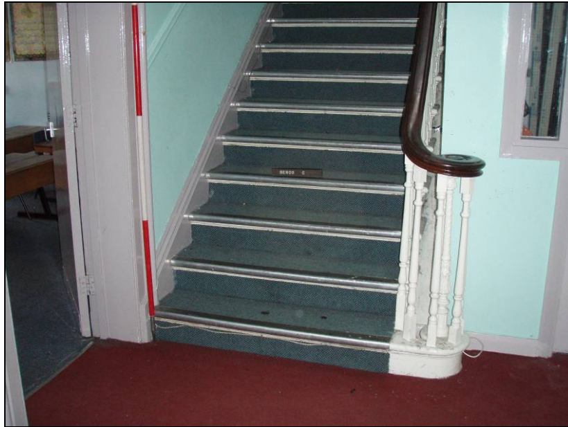
Fig. 20 Staircase to first floor with balustrade
