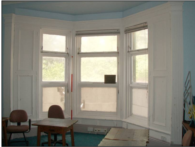
Fig. 14 Internal bay window room 1
