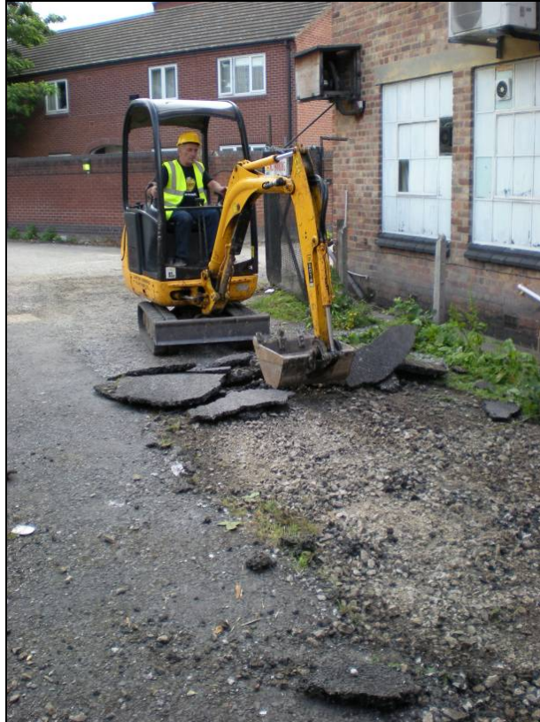
Fig 3. Initial removal of concrete from area to be excavated.
