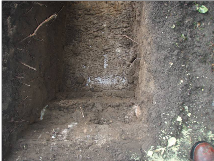
Fig 5. Foundation trench
