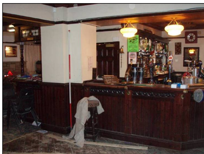
Fig19. Room2 Bar area, looking east (scale=2m)
