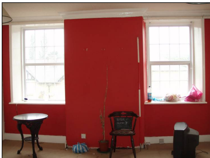
Fig29. Room 7, looking north (scale=2m)
