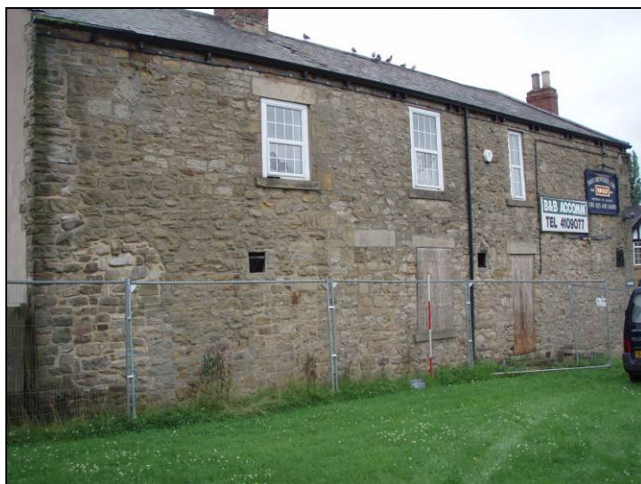
Fig41. Exterior east facing elevation, looking north-west (scale=2m)
