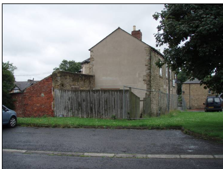
Fig40. Exterior south facing elevation, looking north (scale=2m)
