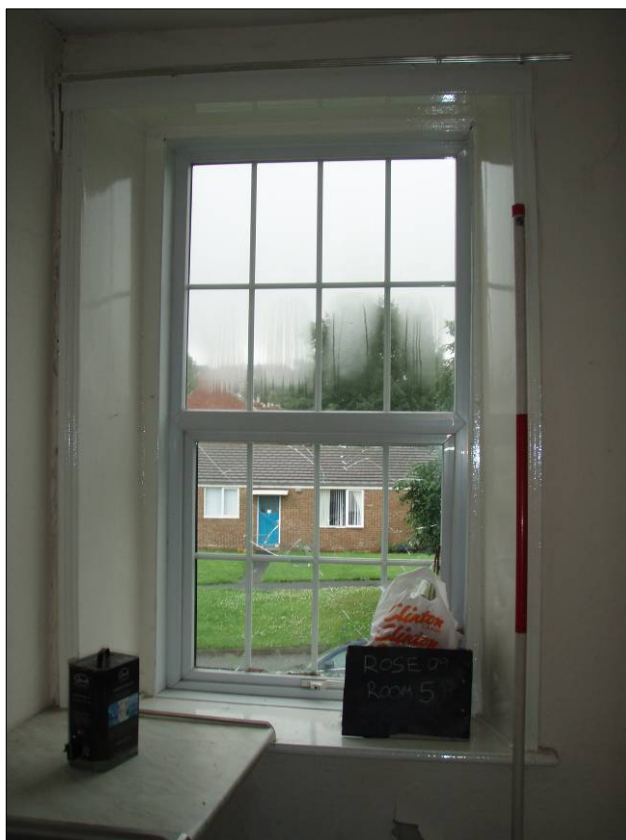
Fig27. Room 5, looking east (scale=2m)
