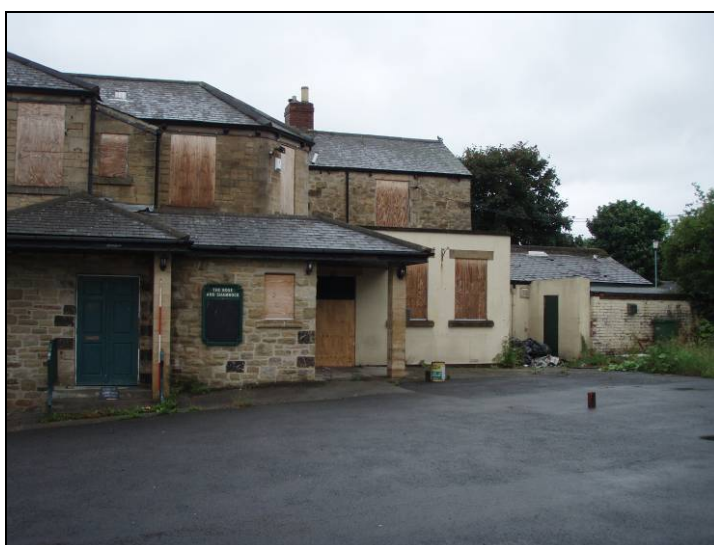
Fig36. Exterior west facing elevation, looking south east (scale=2m)
