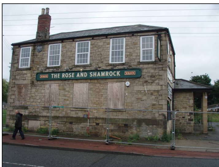
Fig39. Exterior north facing elevation, looking south (scale=2m)
