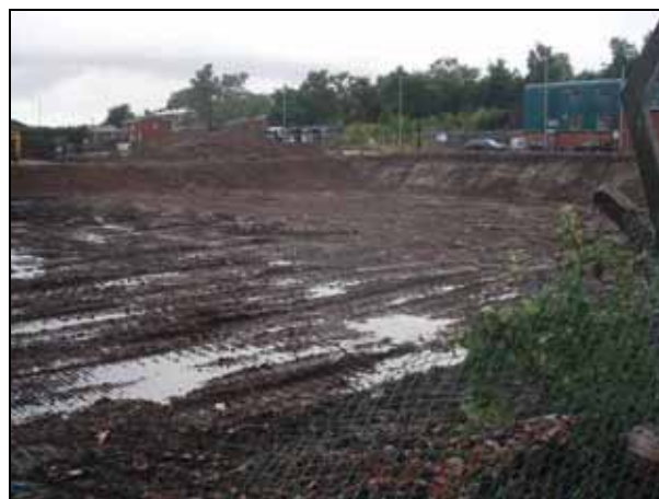
Fig. 12 Area 1 showing demolition.
