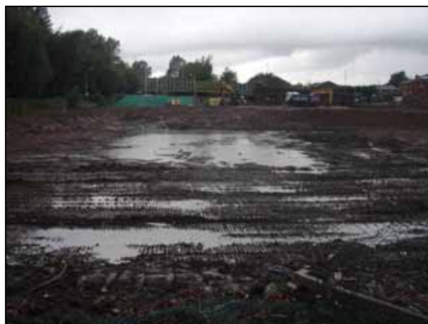
Fig. 11 Area 1 showing demolition.
