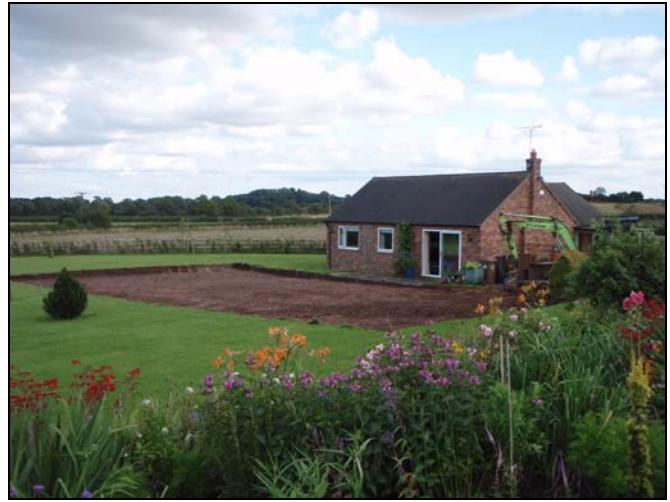
View of the existing bungalow and the stripped trench
