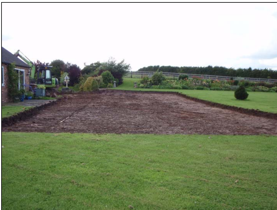
Fig. 5 View of the completed trench.
