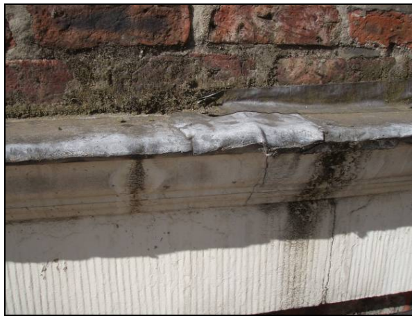
Fig. 24 Lead plated cill
