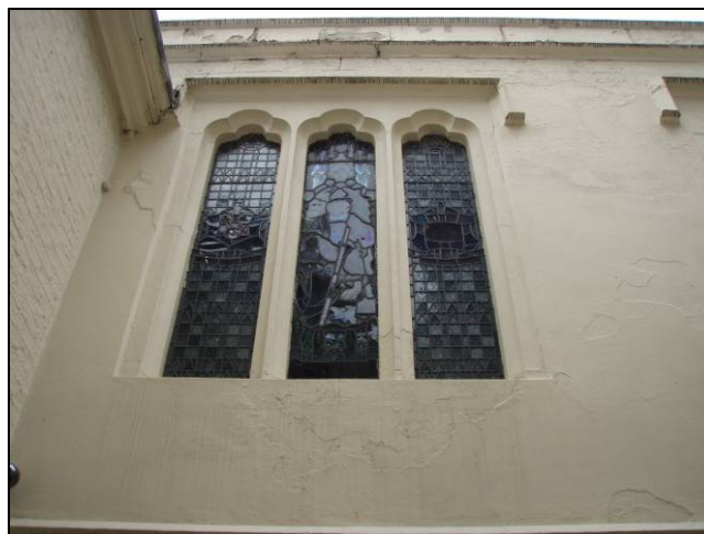
Fig. 8 First floor stained glass windows of entrance passage.
