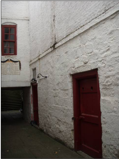
Fig. 18 South East facing elevation of rear access passage
