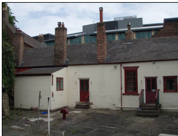
Fig. 16 South West facing elevation of Trinity Chare
