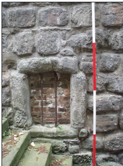
Fig. 17 South East facing elevation of stair case
