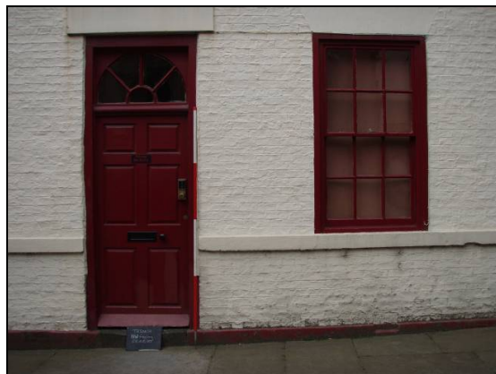
Fig. 14 North East facing elevation ground floor door of Trinity Chare
