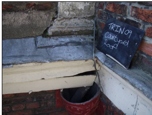
Fig. 25 Lead plated cill above drain
