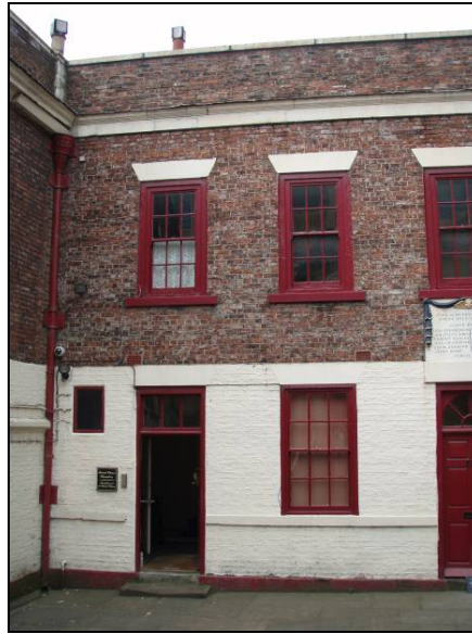
Fig. 12 North East facing elevation of Trinity Chare
