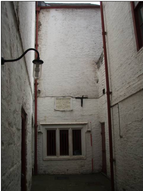
Fig. 20 South West facing elevation of access passage
