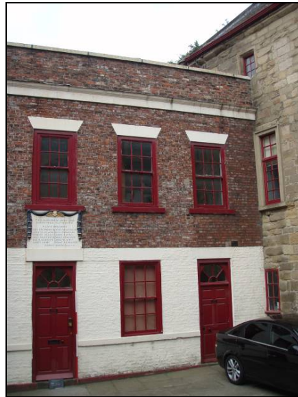
Fig. 13 North East facing elevation of Trinity Chare
