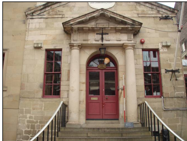
Fig. 4 South West facing elevation showing main entrance
