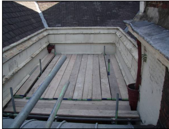
Fig. 26 guttering and cills
