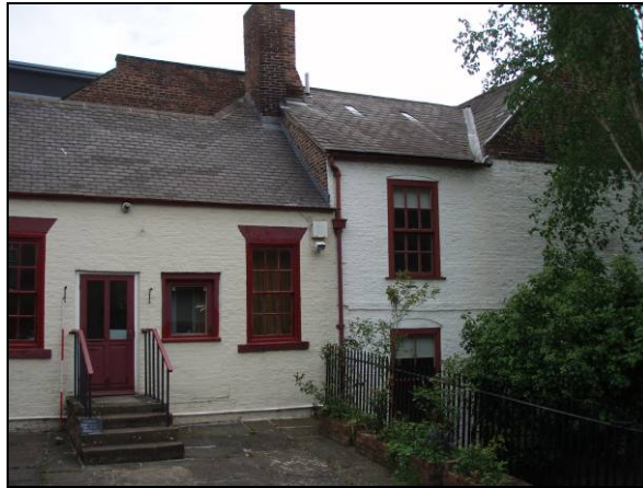
Fig. 15 South West facing elevation of Trinity Chare
