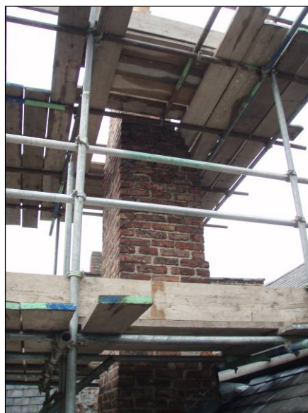
Fig. 29 Chimney of access passage roof
