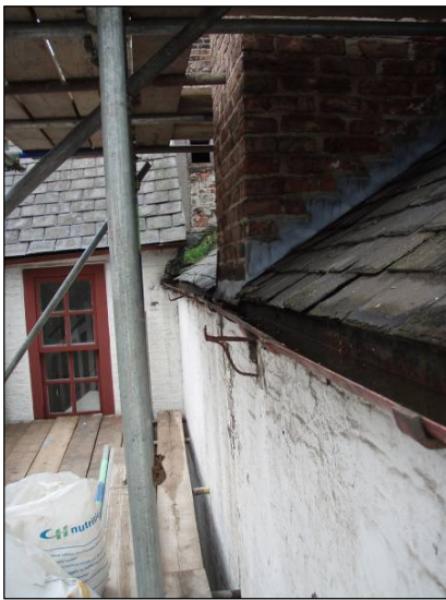
Fig. 27 Guttering of access passage
