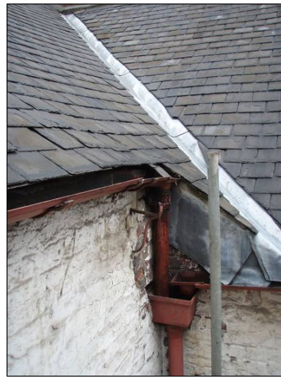
Fig. 28 Guttering of access passage
