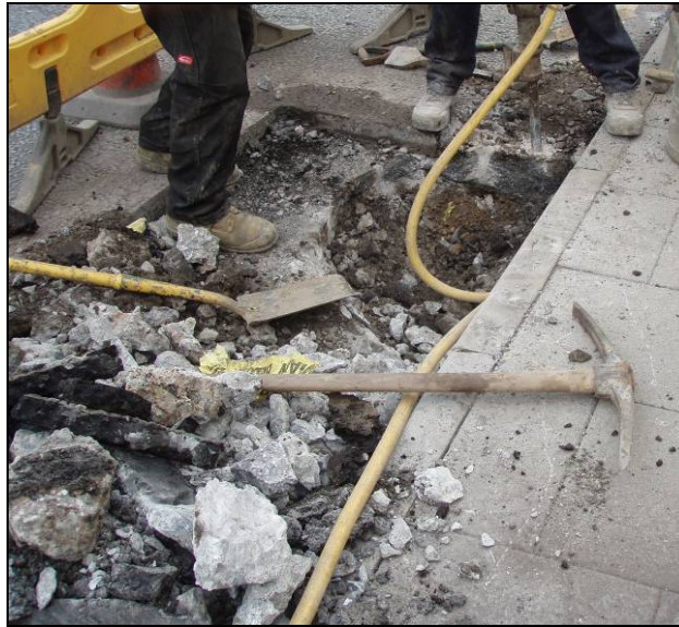
Fig. 3 Open trench showing tarmac, concrete and made ground.
