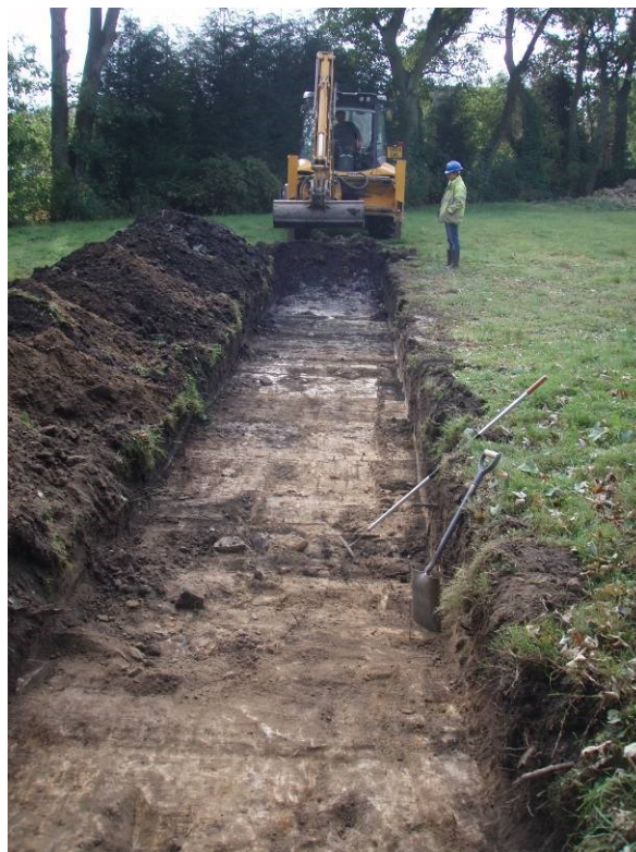
Excavation of the trench, looking south-east
