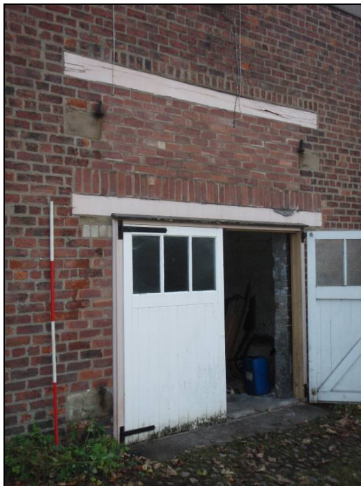
Figure 4: Detail of the Garage door
