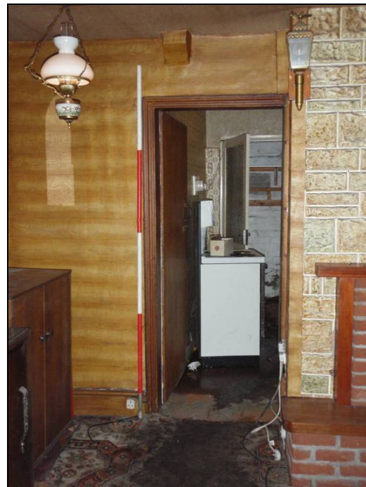
Figure 15: Doorway with a corbel over the lintel
