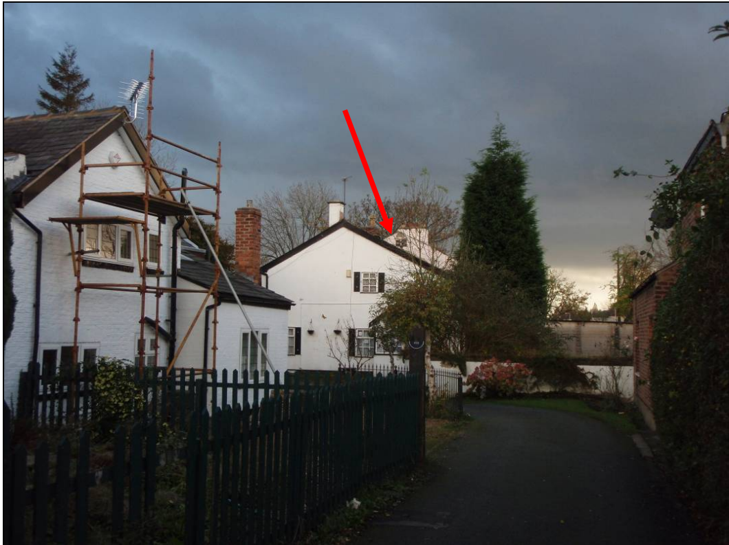
Figure 11: Top of gable of the north elevation indicated by a red arrow
