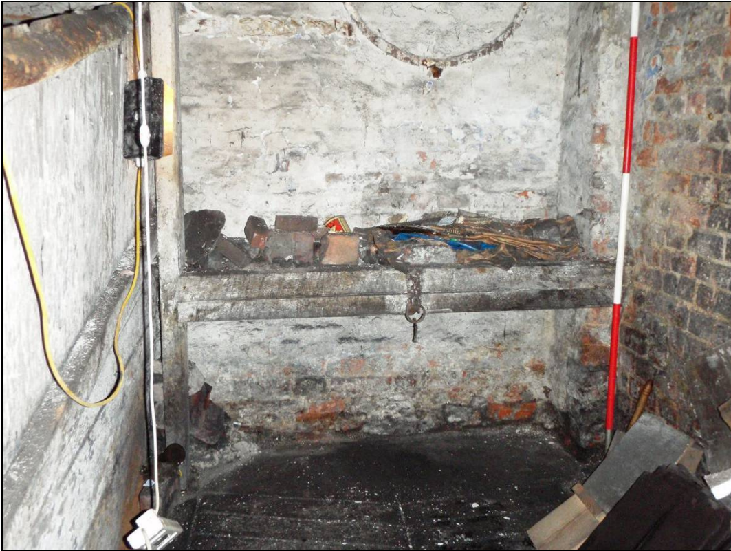
Figure 30: North wall of the Barn showing a neglected trough and signs of a former manger above it
