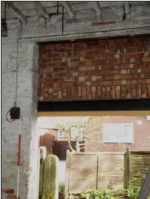
Figure 25: Inserted RSJ lintel of current doorway
