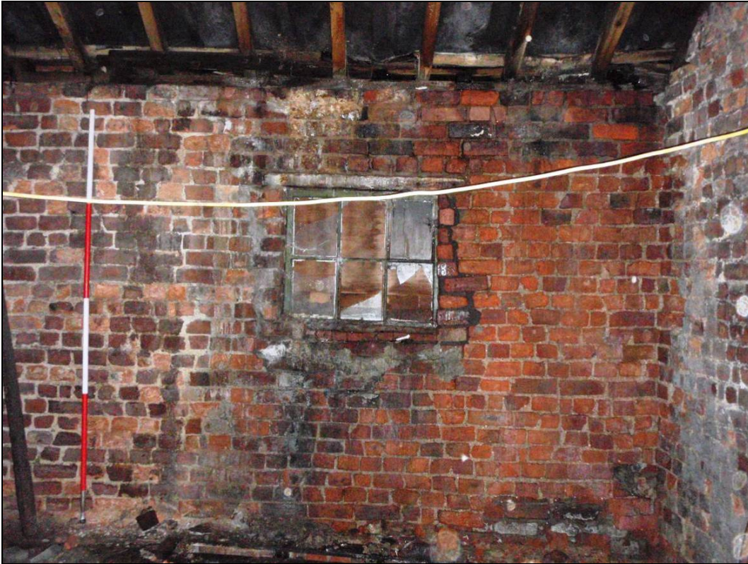
Figure 46: East wall of the Barn with inserted window
