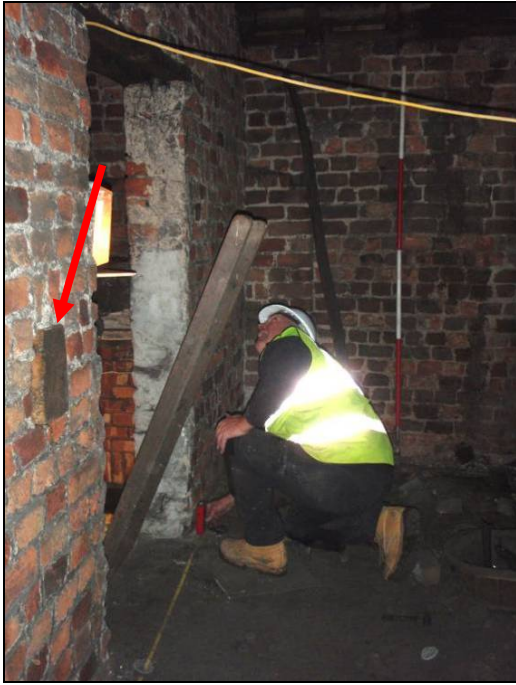
Figure 43: Garage beam indicated with red arrow
