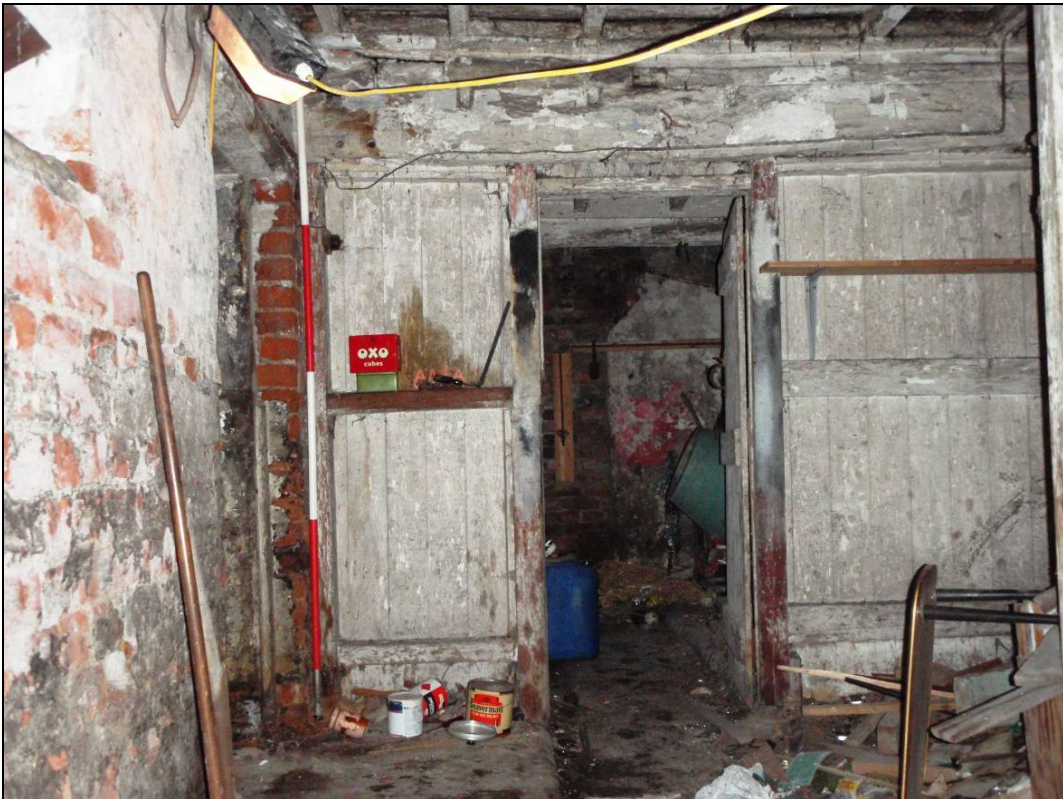
Figure 31: Timber partition to western side
