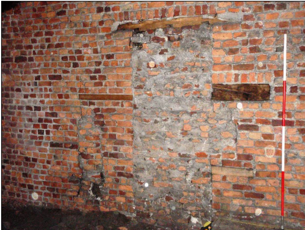
Figure 42: North wall of the Barn with blocked-up doorway
