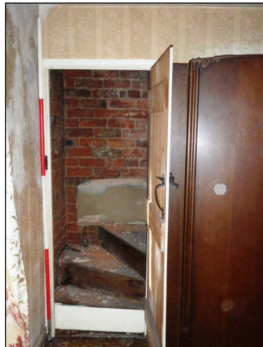
Figure 38: Staircase to the Loft Room
