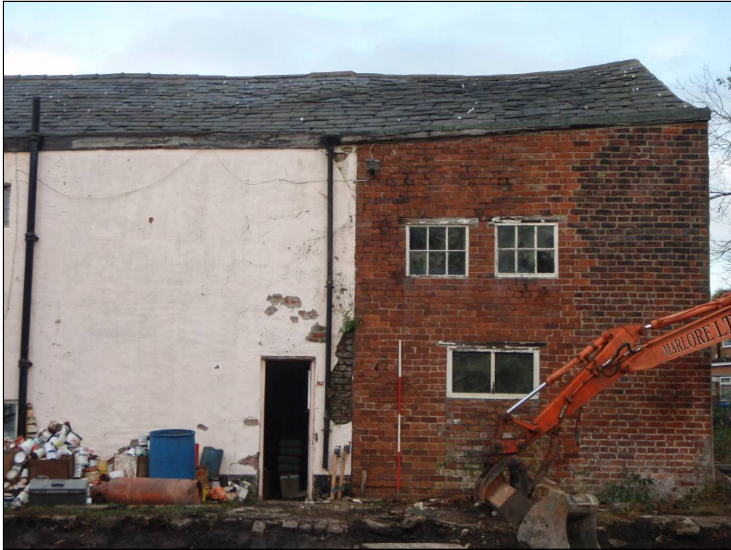
Figure 8: The southern end of the west elevation
