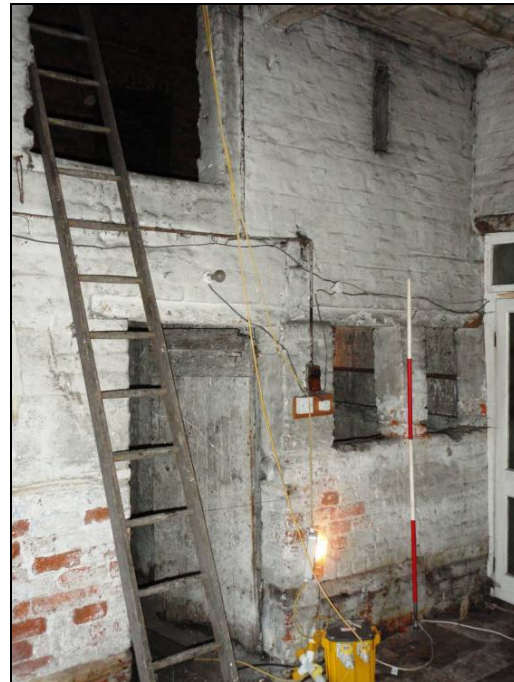
Figure 26: South wall of the Garage
