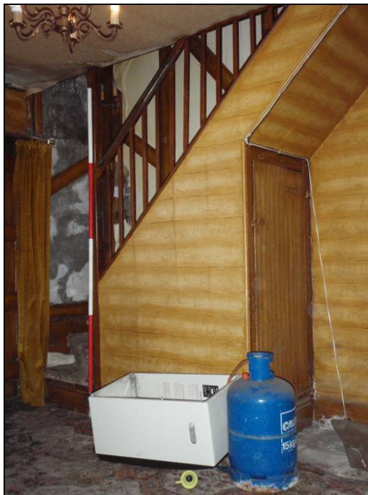
Figure 14: Staircase to the first floor
