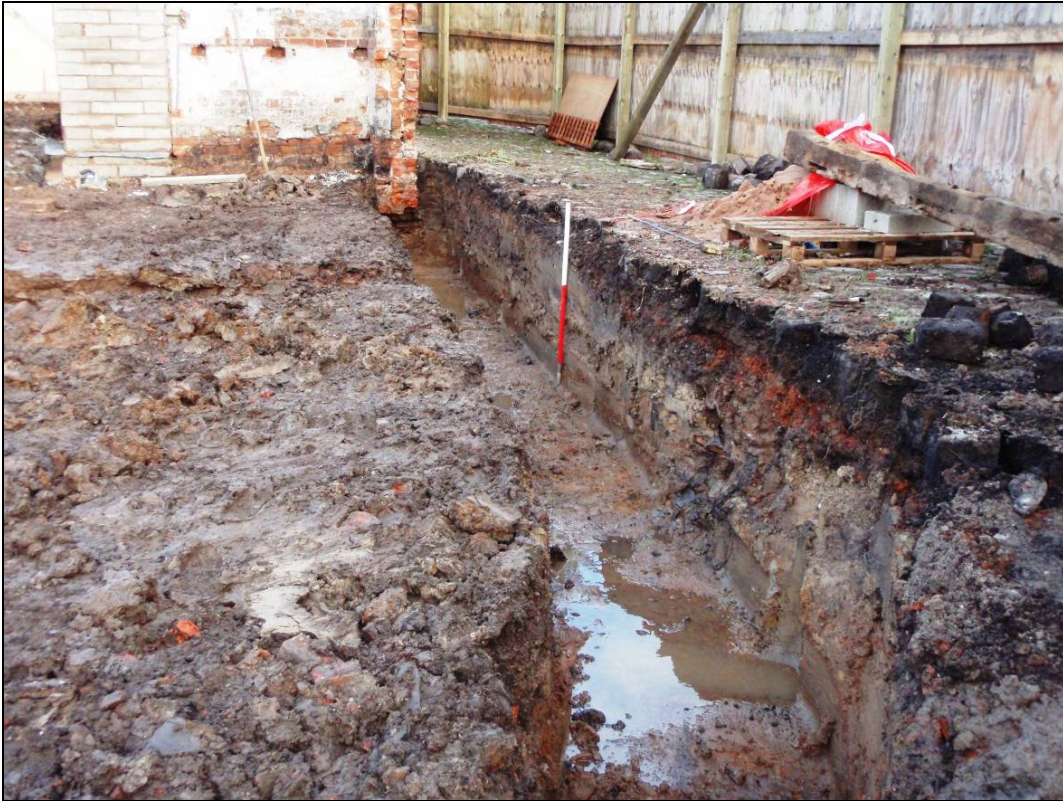
Figure 51: N/S foundation trench along the eastern side
