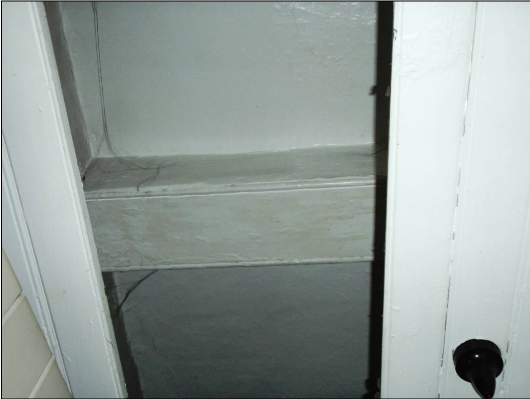
Figure 22: View of a ceiling beam revealed above the current false ceiling
