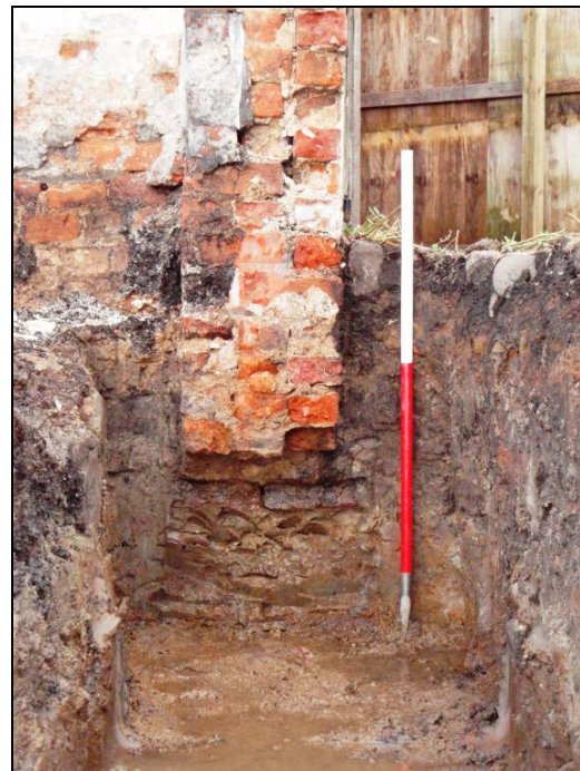
Figure 53: Foundation wall on the eastern side
