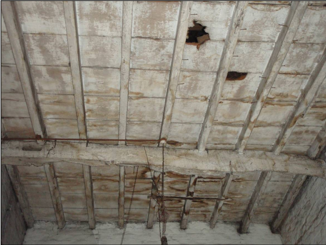
Figure 29: Ceiling structure of the Garage
