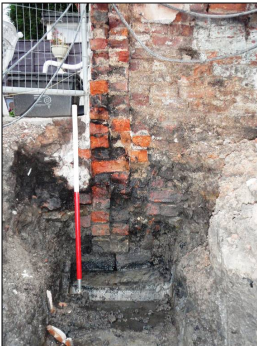
Figure 52: Foundation wall on the western side
