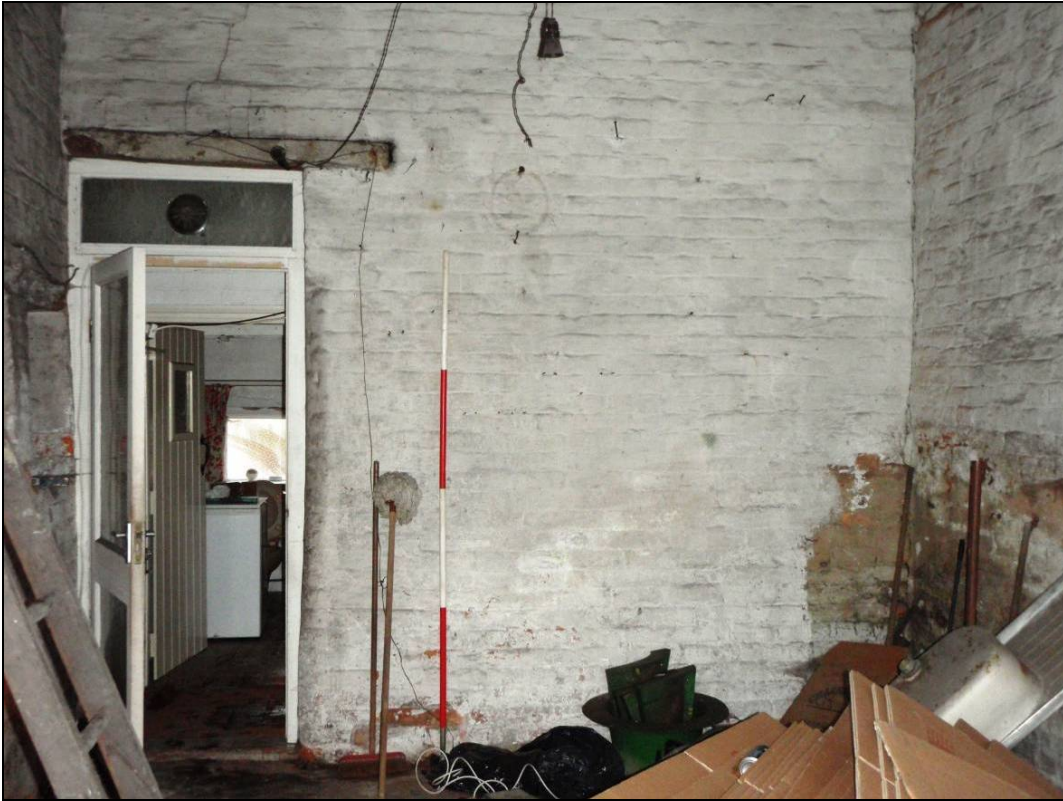
Figure 27: Inserted partition wall between the Kitchen and the Garage, looking west
