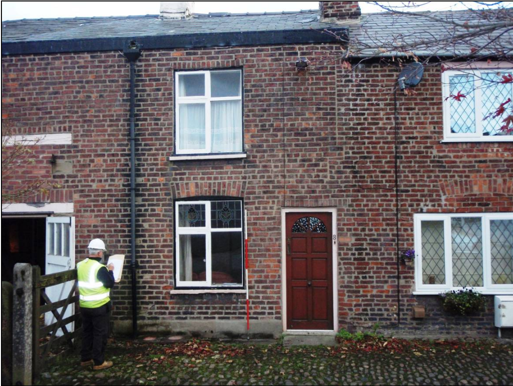
Figure 3: Detail of the doorway of the building with adjacent house no. 6 on the right
