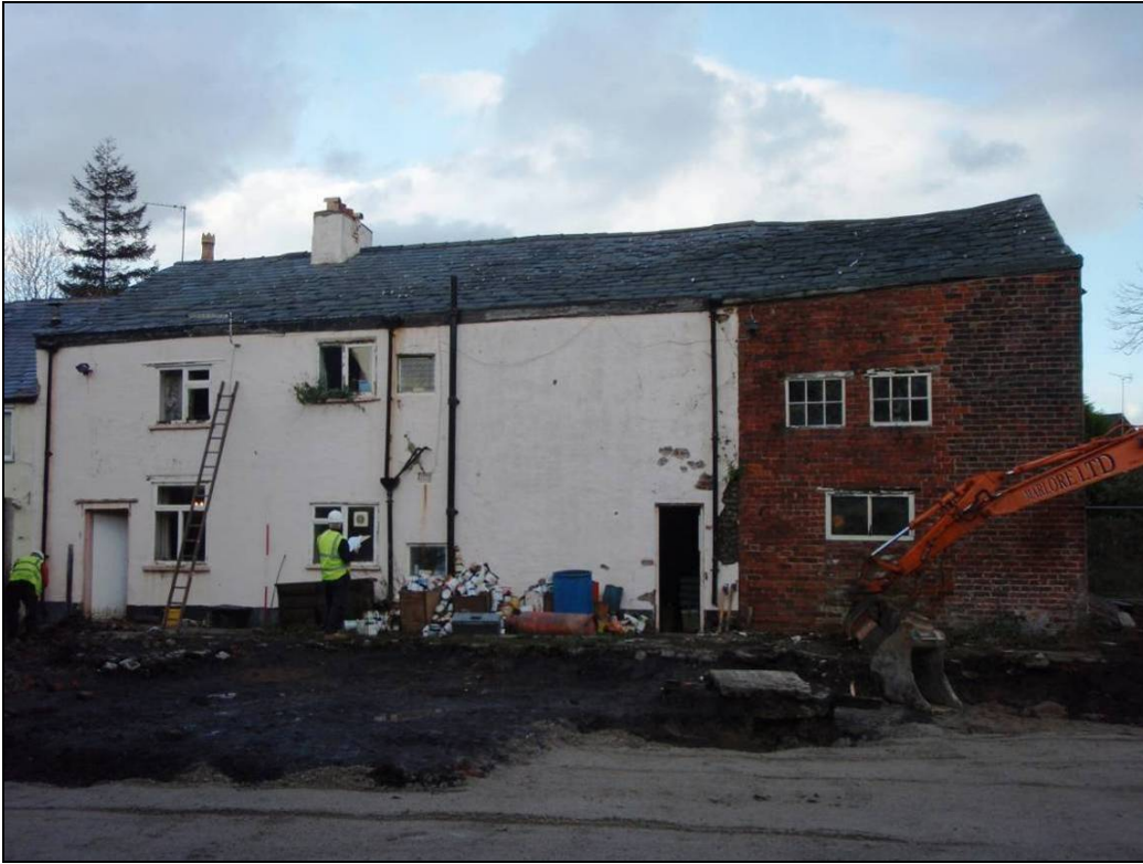
Figure 6: General view of west elevation
