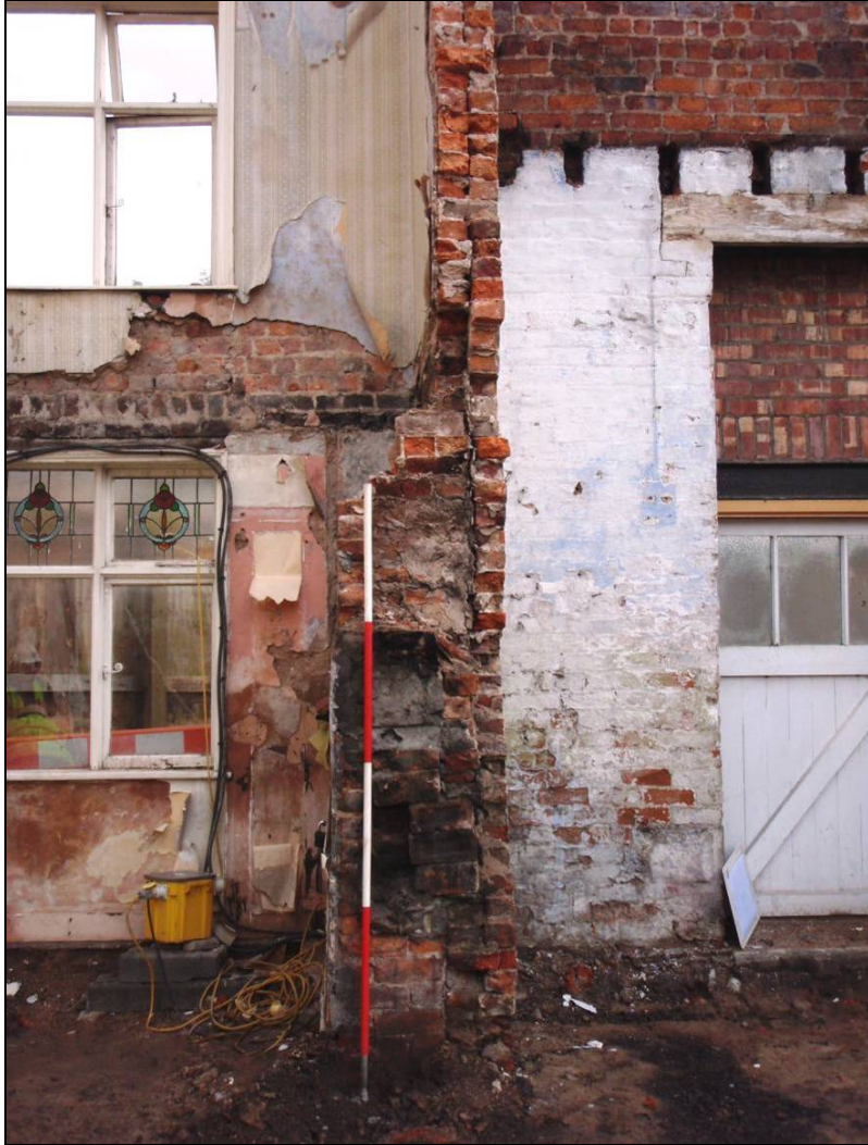
Figure 50 Section through the fireplace after partial demolition
