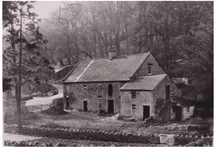
1967 photograph of Lode Mill looking northwest (Staffordshire County Council)
