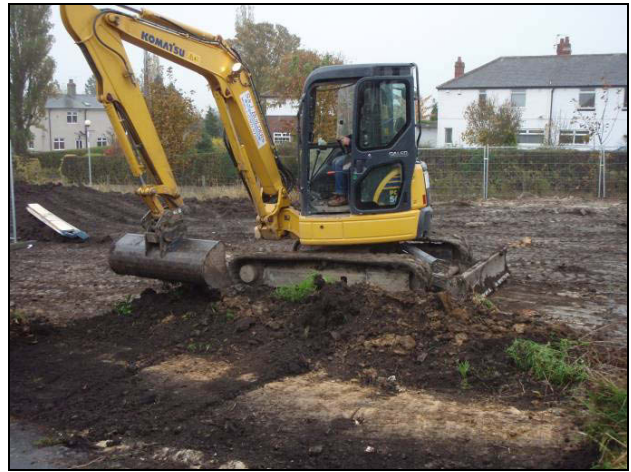
Undertaking of Ground Reduction
