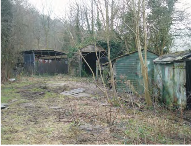
Figure 16: Derelect sheds/former workshops at the entrance of the former quarry
