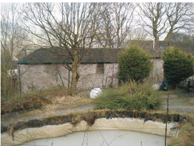
Figure 23: From the front of Peveril Croft, looking north towards the listed Former Stables of Castleton Hall
