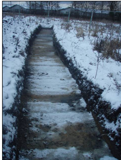
Trench 3 beginning to fill with snow
