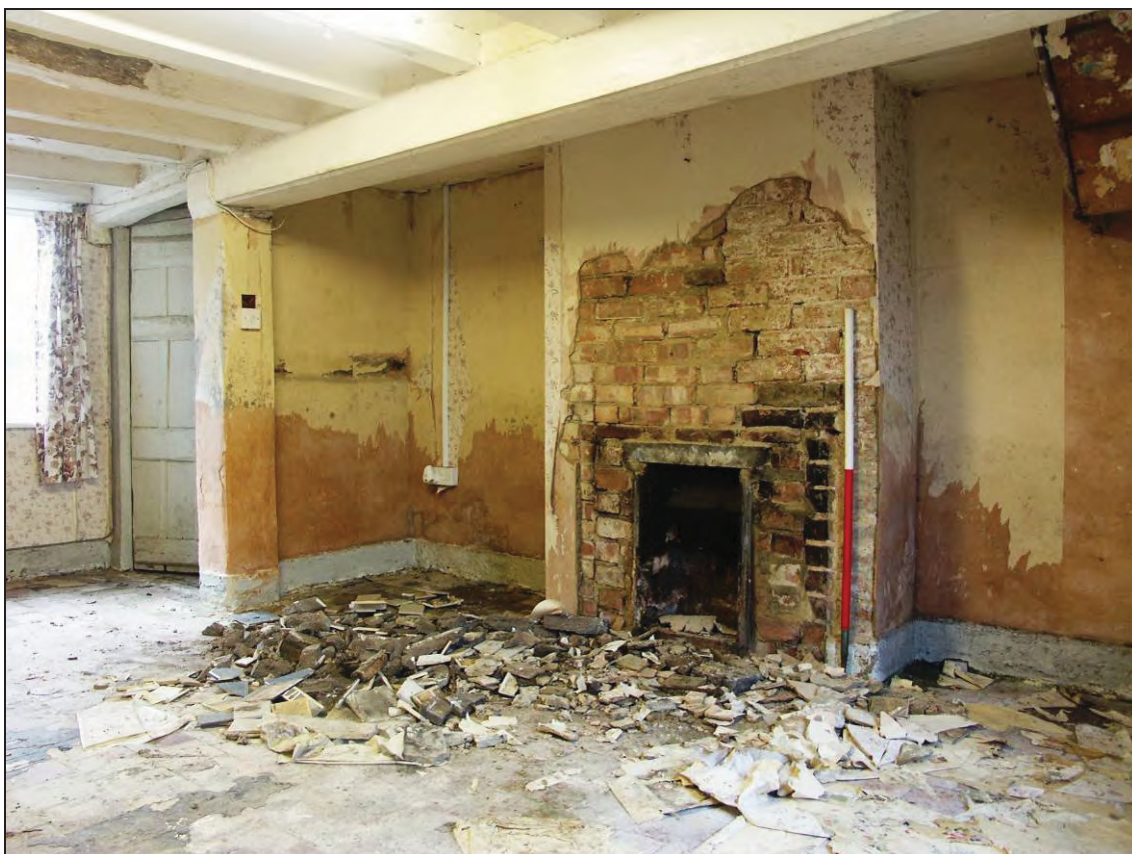
Figure 44: Fire place on the northern wall of room G-4 (scale 1m)
