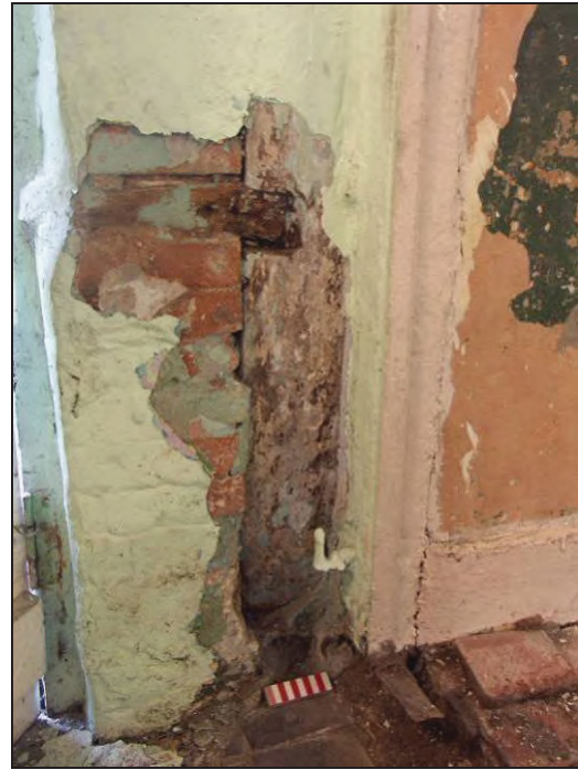
Figure 28: Inclined S-E post in room G-2
