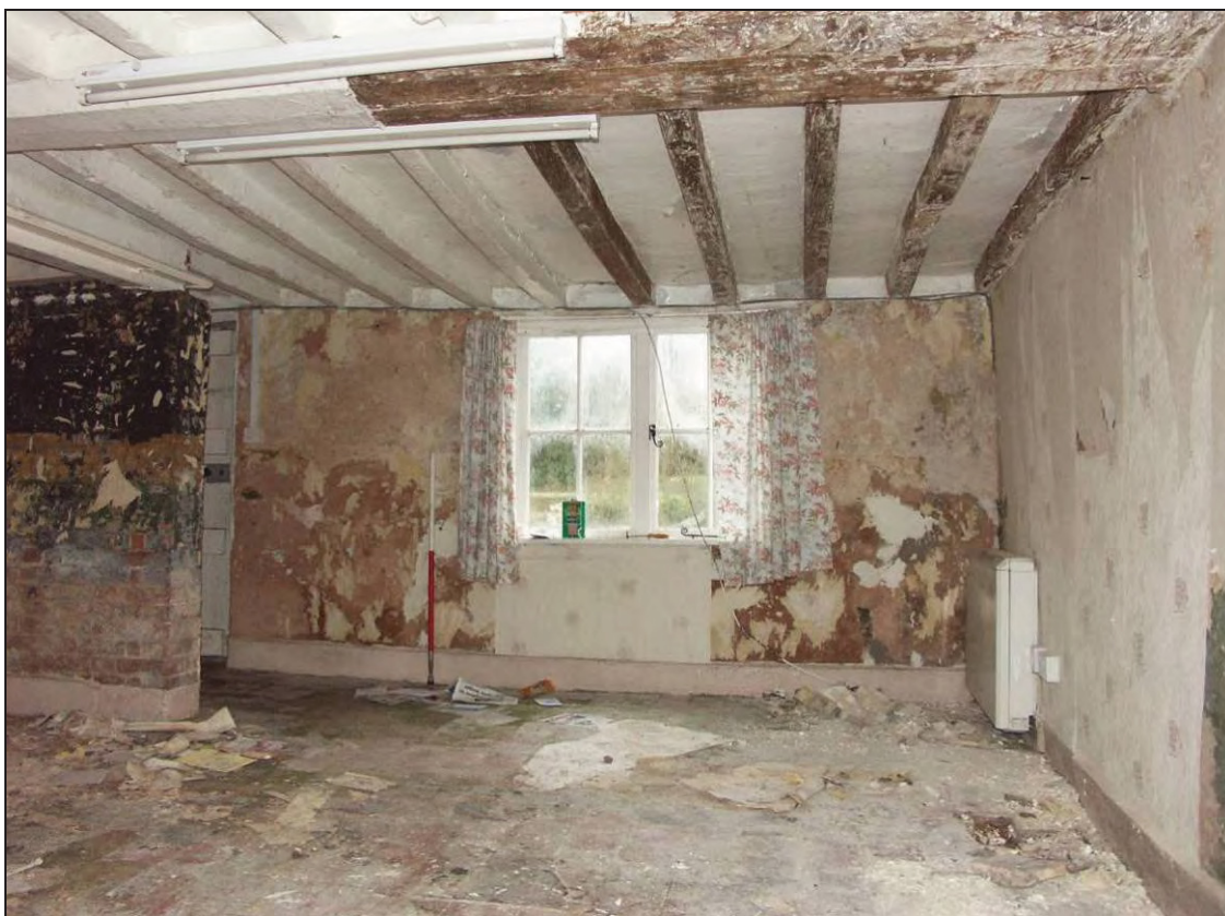
Figure 35: Room G-3, looking west (scale 1m)
