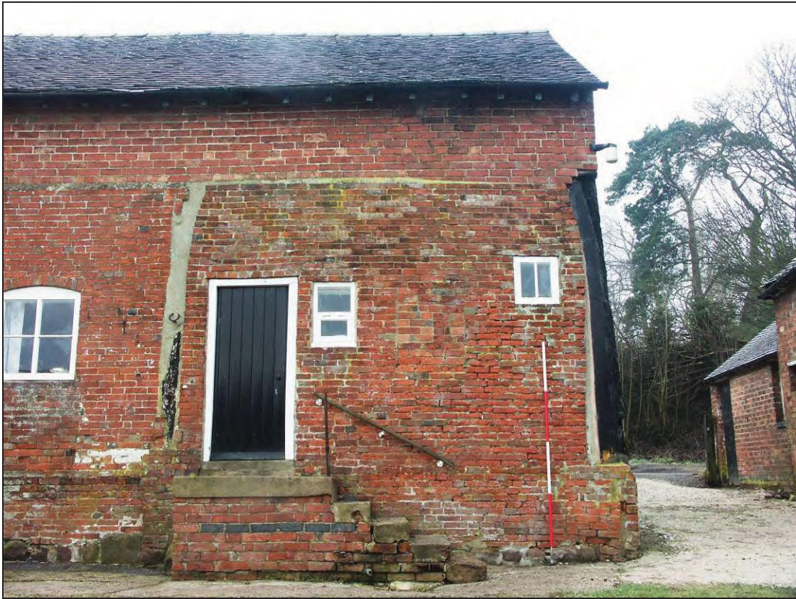
Figure 18: Northern bay with remains of timber-framed building (scale 2m)
