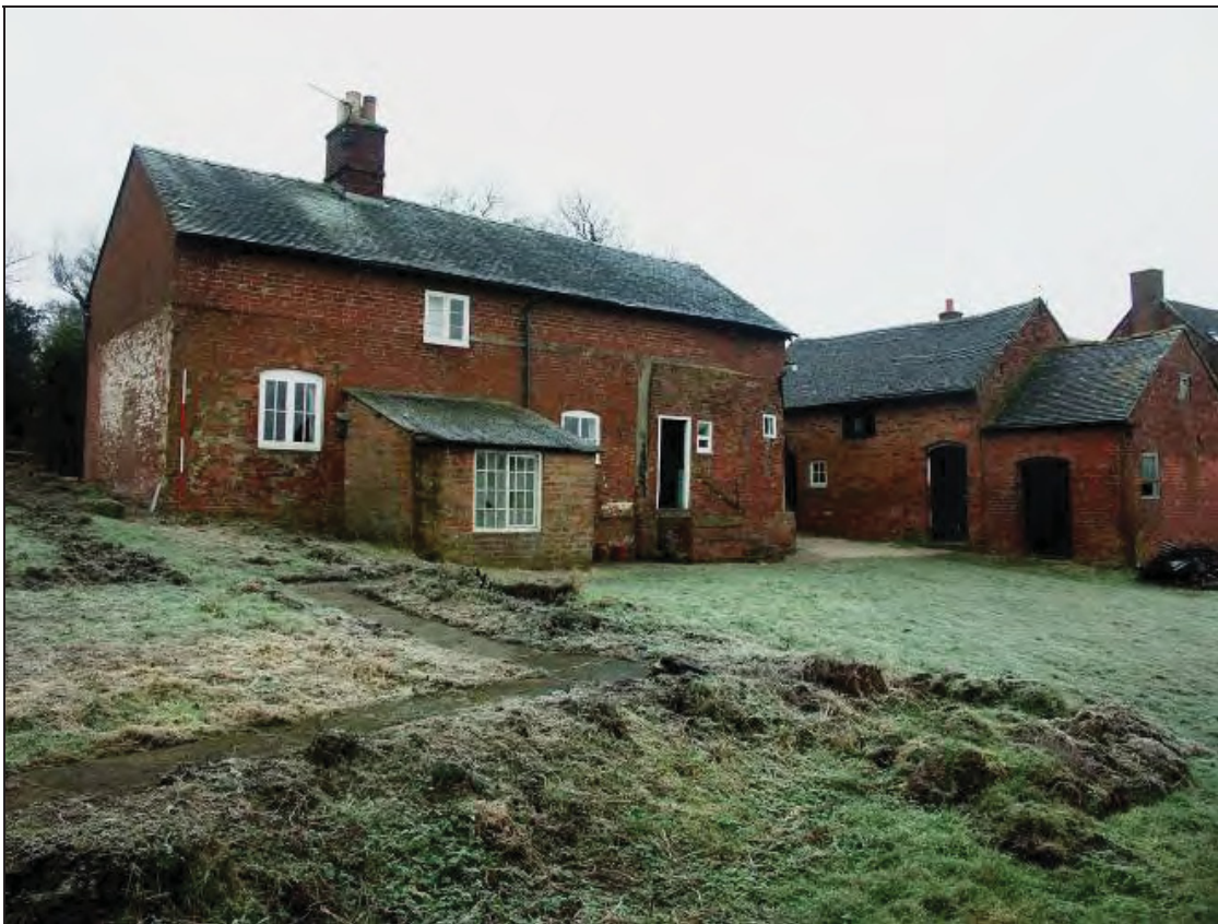
Figure 12: General view of the east elevation (scale 2m)
