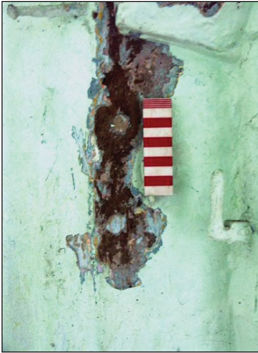
Figure 27: Surviving brace pegs on the S-E post
