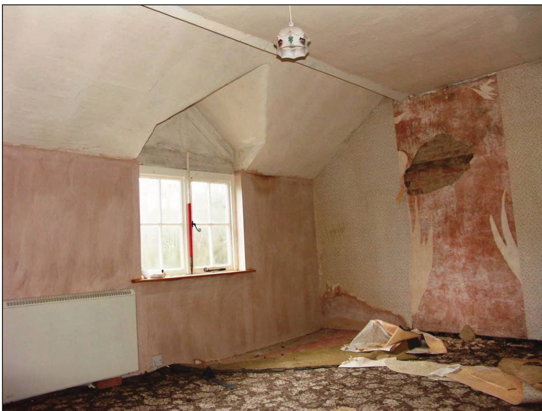
Figure 57: Western wall with repaired plaster work (scale 1m)
