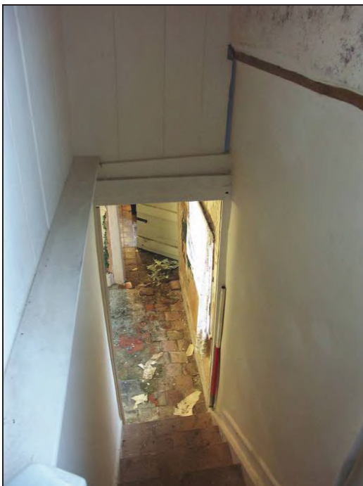
Figure 46: Staircase with timber wall plate (scale 1m)
