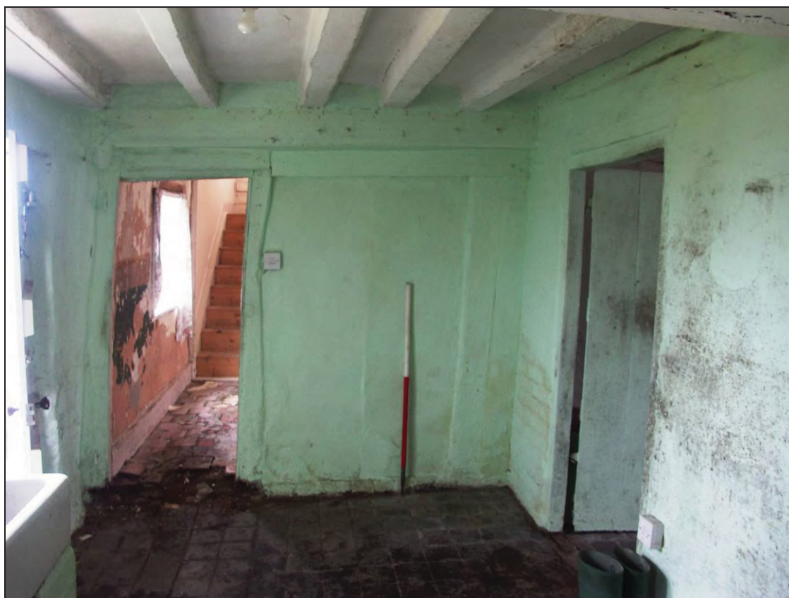
Figure 26: Eastern wall of room G-1 with surviving timber stud and rail (scale 1m)
