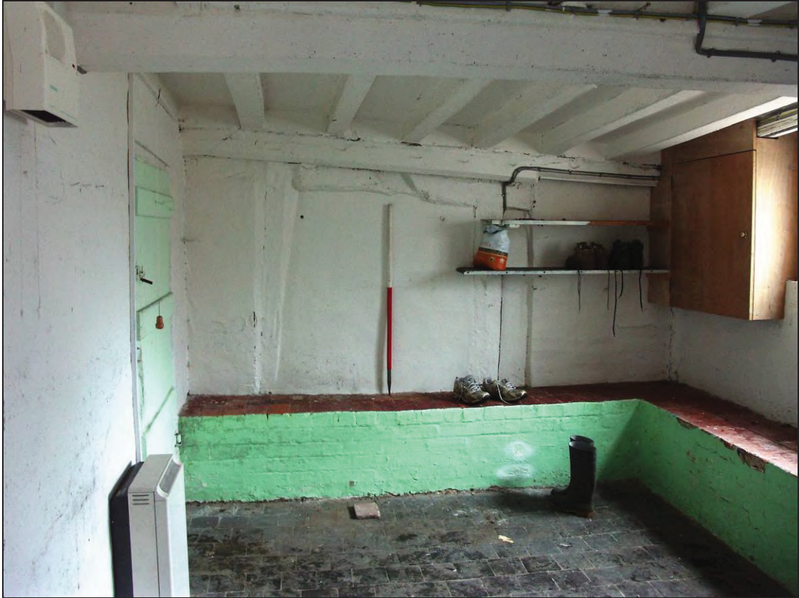
Figure 29: Surviving timber frame on the south wall of room G-2 (scale 1m)
