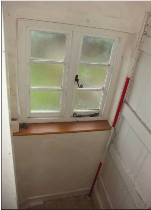
Figure 48: Window on the landing (scale 2m)
