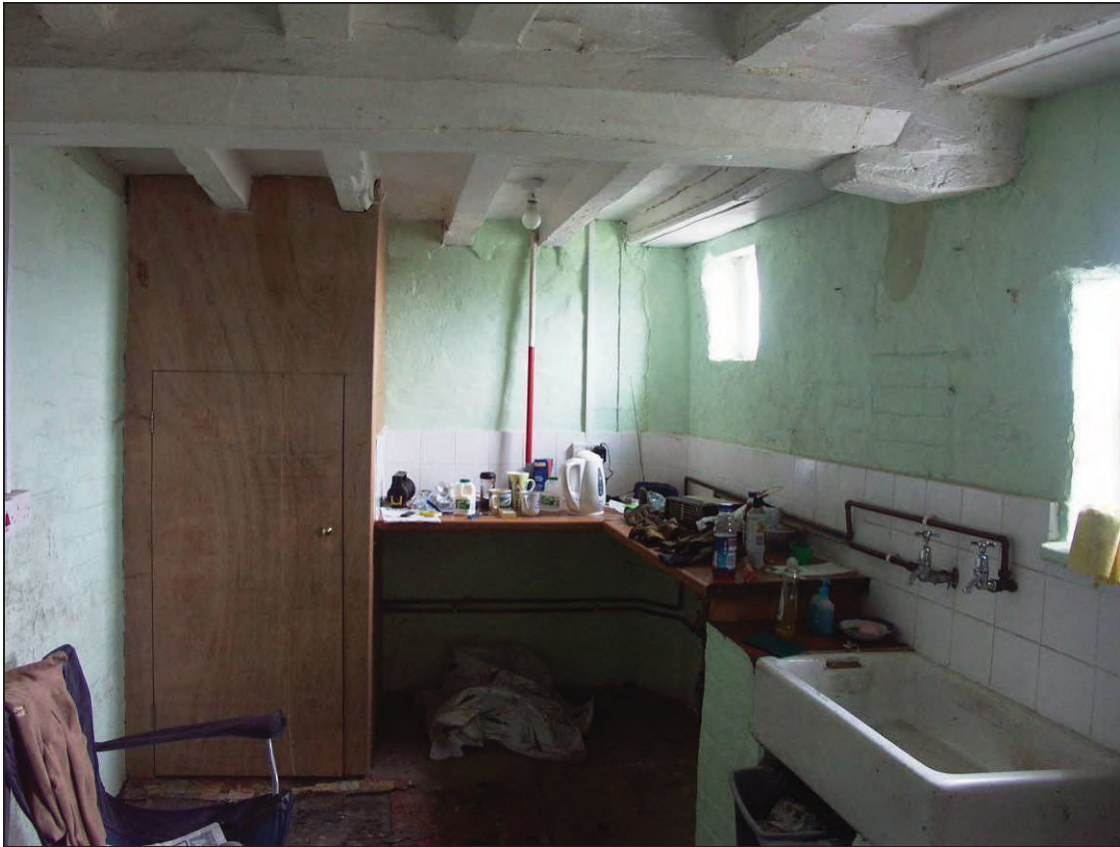
Figure 24: Southern wall of room G-1 (scale 1m)
