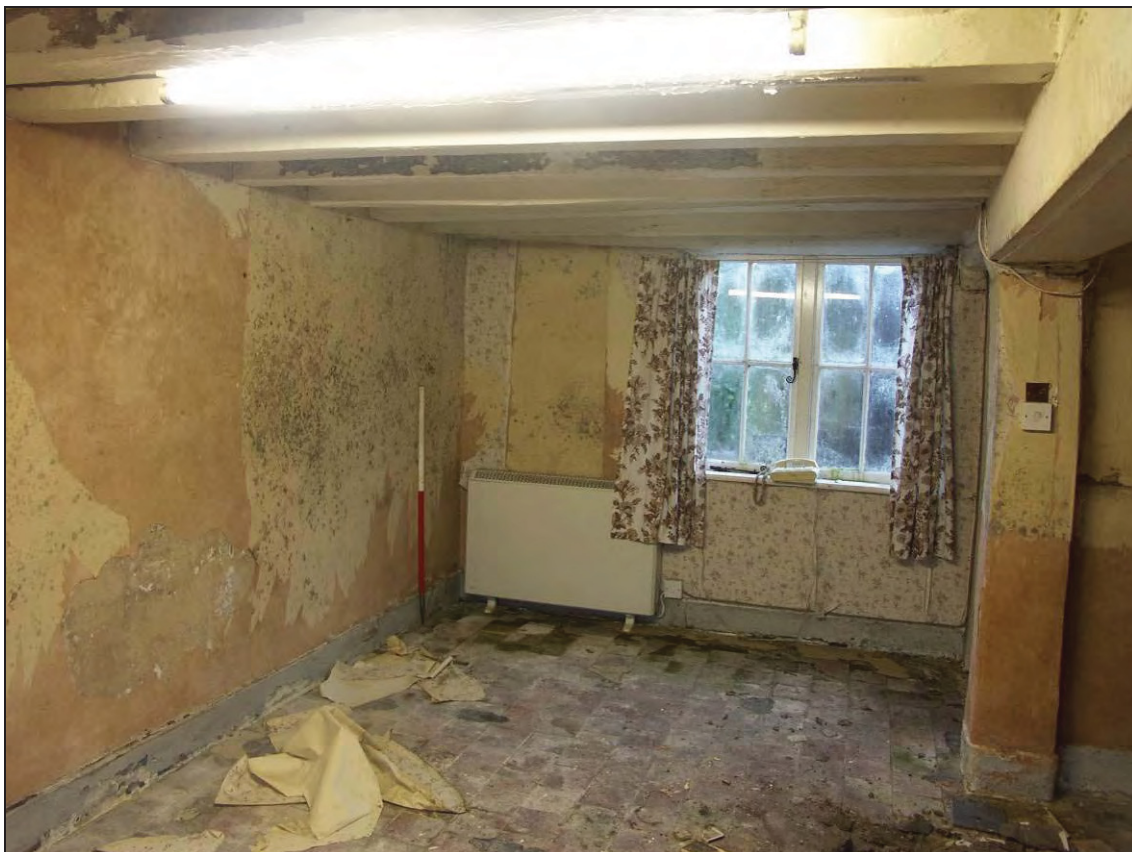
Figure 43: Room G-4, looking west (scale 1m)
