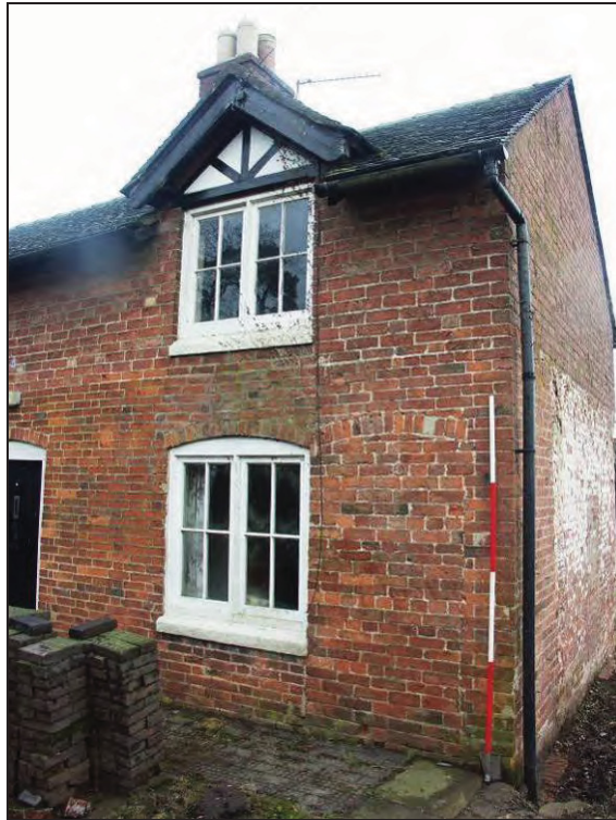
Figure 10: Former doorway blocked-up (scale 2m)
