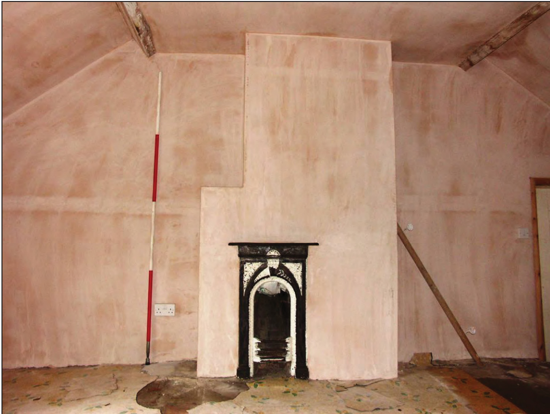
Figure 62: Central cast-iron fire place, looking north (scale 2m)
