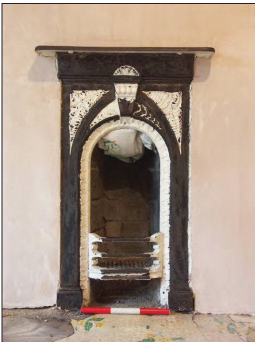
Figure 63: Detail of cast-iron fire grate (scale 300mm)
