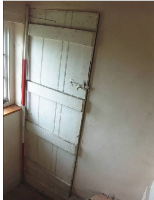
Figure 49: Doorway to room F-3 (scale 2m)
