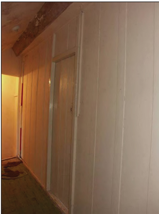
Figure 50: Panelling along the passageway (scale 2m)
