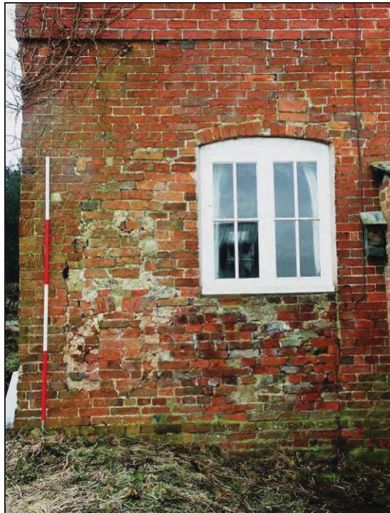
Figure 14: Southern bay with bricked-up oven
