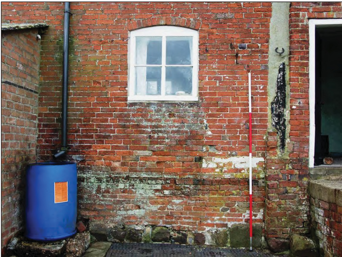
Figure 17: Exposed rubble stone foundation supporting a brick plinth (scale 2m)
