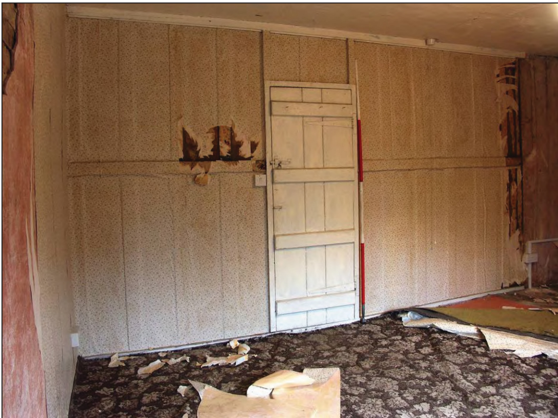
Figure 55: Wood panelling with doorway to the passageway, looking east (scale 2m)
