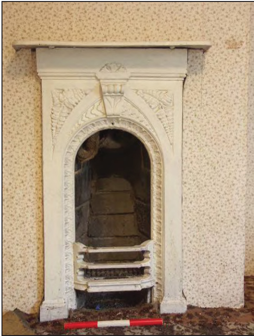
Figure 58: Detail of cast-iron fire grate (scale 300mm)
