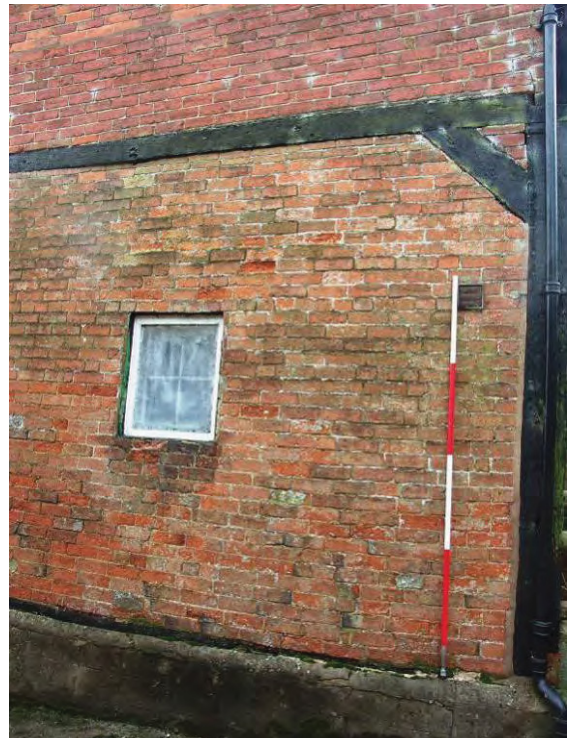
Figure 22: Detail of timber post, brace and wall plate
