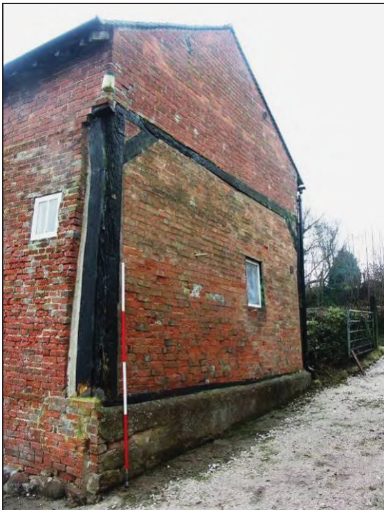
Figure 21: North elevation with timber frame
