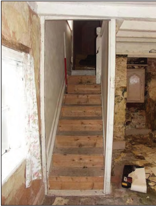
Figure 41: Staircase to the upper floor (scale 1m)
