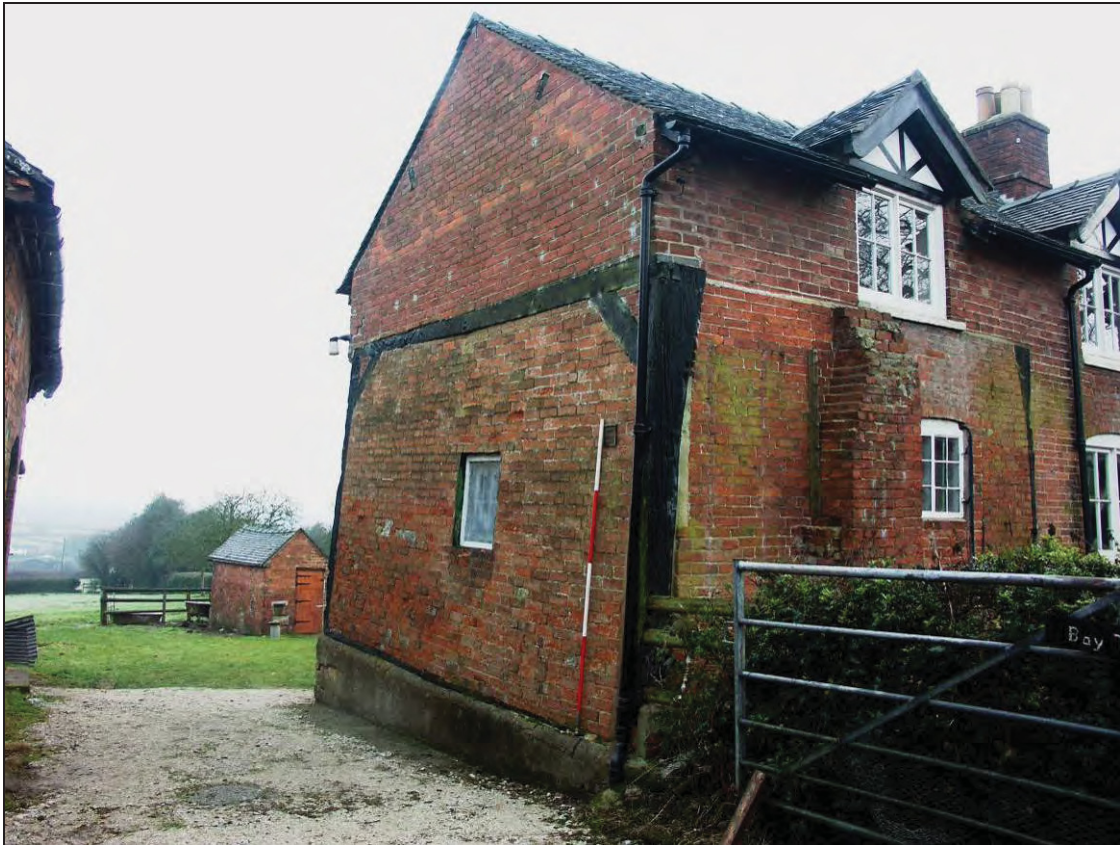
Figure 23: Former timber frame building incorporated into the main house (scale 2m)
