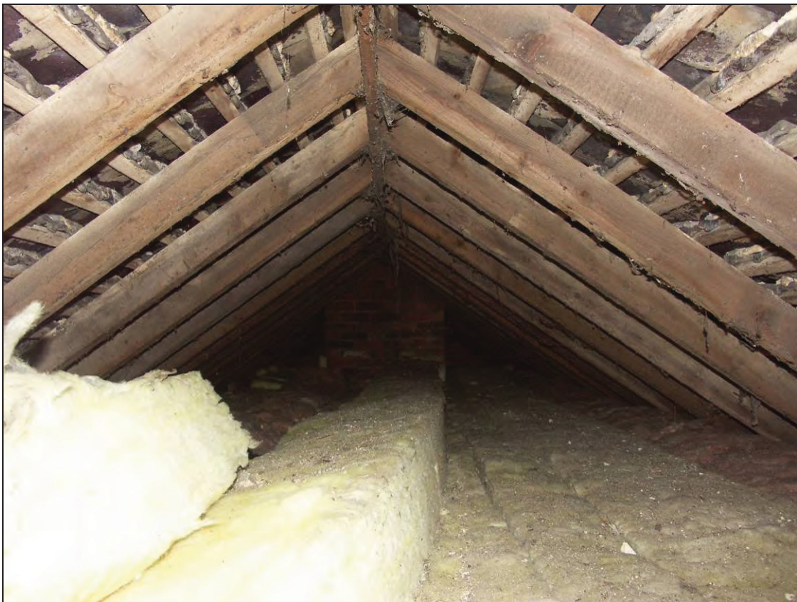
Figure 54: Inside the roof structure, looking south
