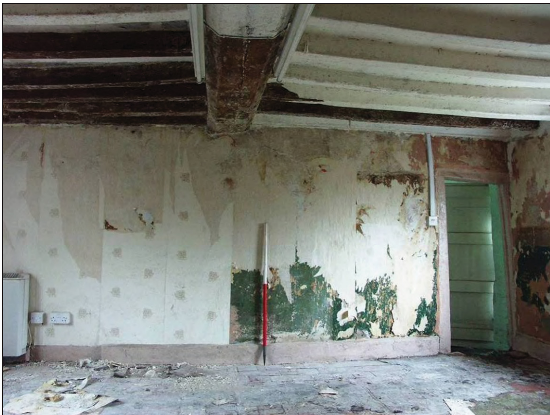
Figure 34: General view of room G-3, looking north (scale 1m)
