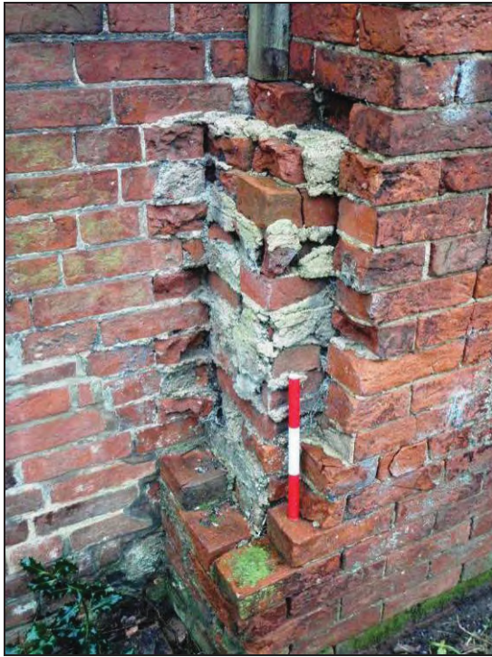
Figure 7: Brick infill inside the former fire place (scale 300mm)
