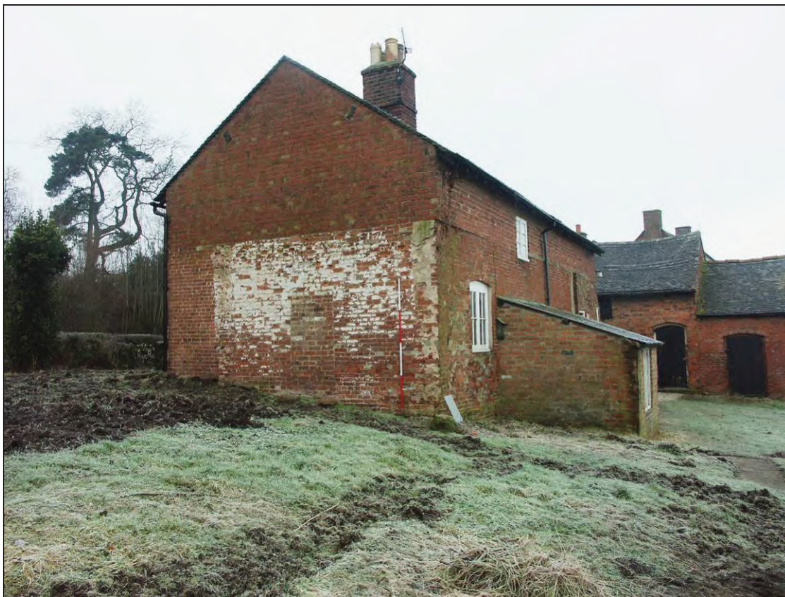
Figure 19: General view of the south elevation (scale 2m)
