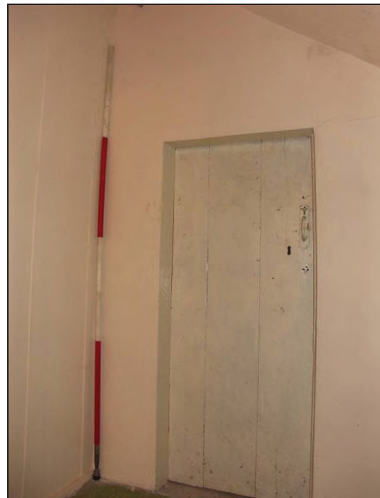
Figure 51: Doorway to room F-1 (scale 2m)
