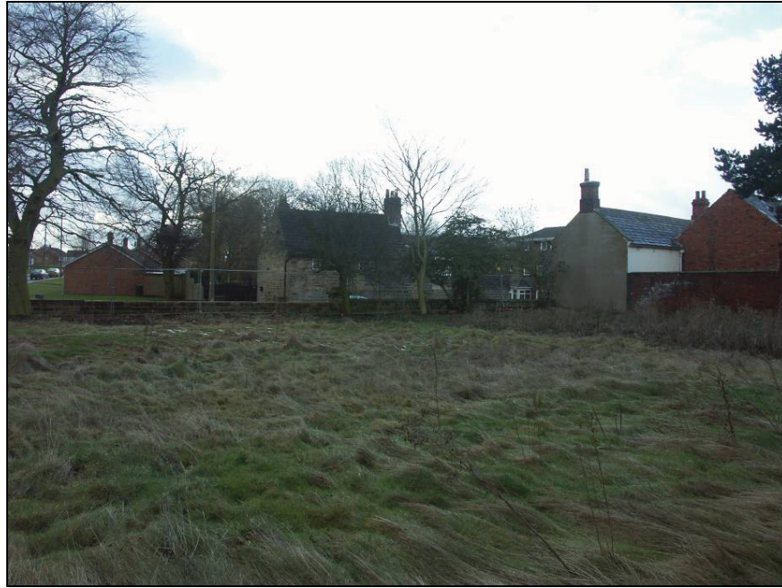
Fig. 24 View of out the front of the hall looking towards Church Street which would have been a former lawn.
