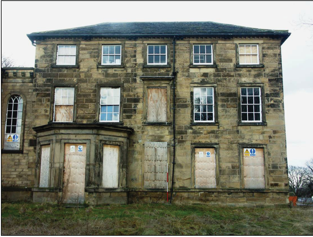
Fig. 27 Western elevation of Brierley Hall
