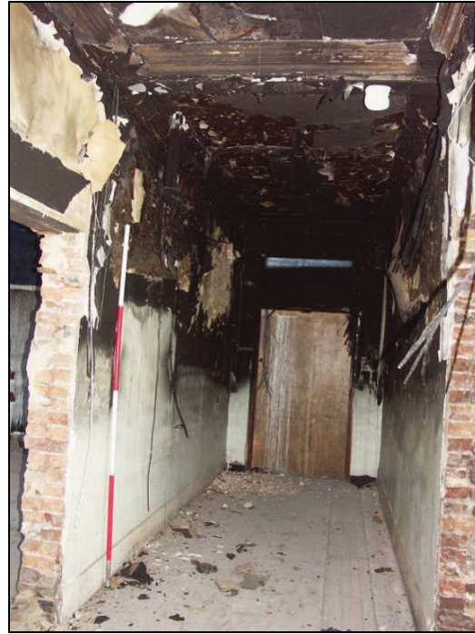
Fig. 35 Hallway on the first floor
