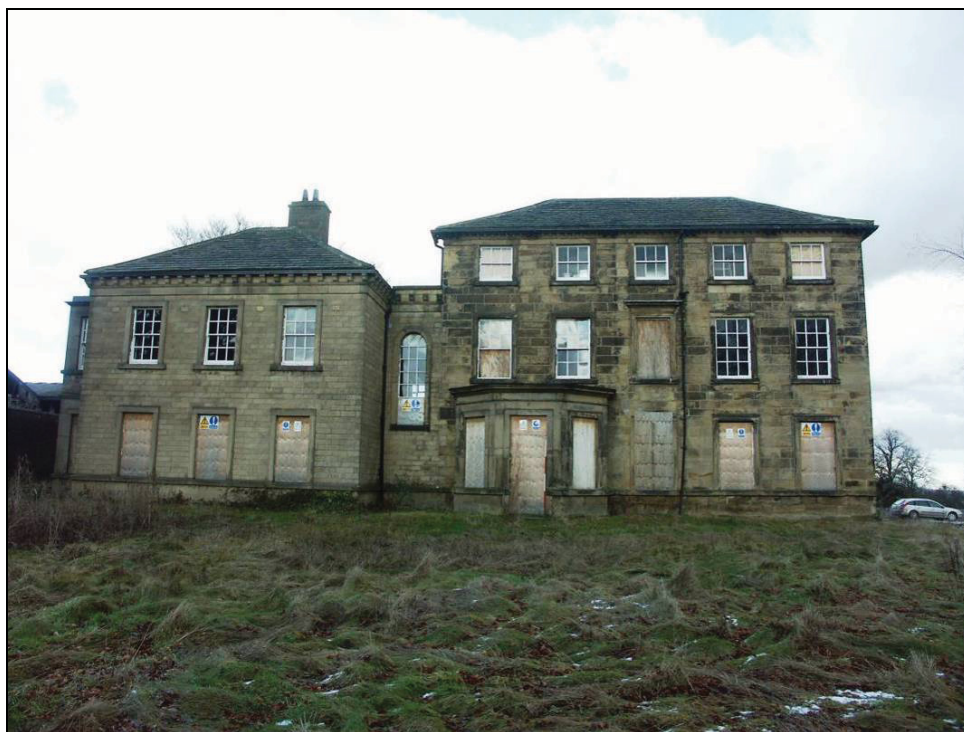
Fig. 25 Western elevation of Brierley Hall (on the left) and the north-western wing (on the right)
