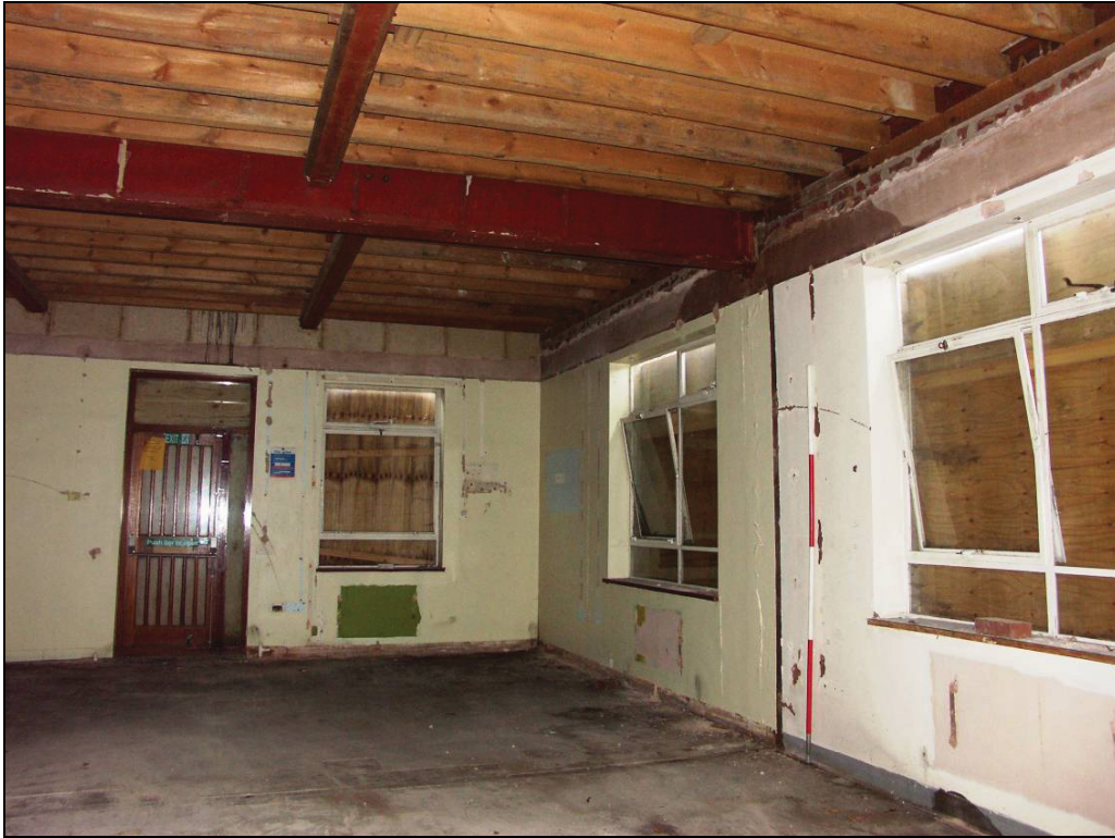
Fig. 50 Interior view of the modern building, looking north
