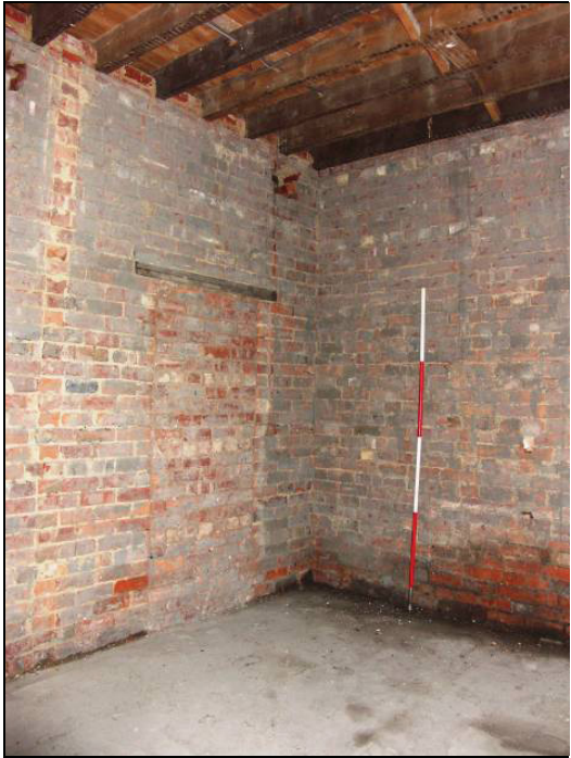
Fig. 48 View of a room in the rear extension
