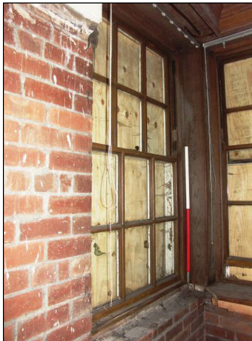
Fig. 45 Detail of horned sash window
