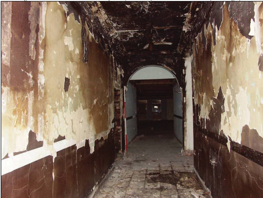
Fig. 29 Hallway on the ground floor
