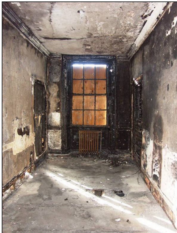
Fig.37 Window on the central bay of the first floor with additional radiator
