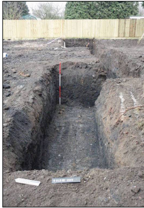
Fig. 8: Post excavation of soakaway 3 Facing East, scale 2m
