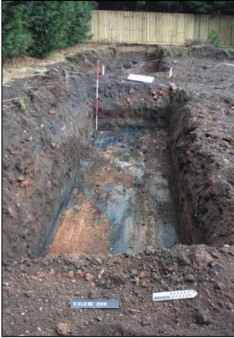
Fig. 7: Post excavation of soakaways 1 & 2. Facing West, scale 2m
