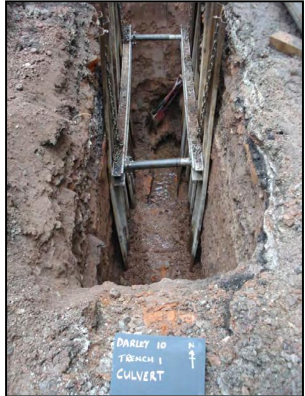
Trench 1 with culvert
