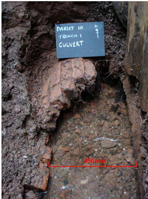
Fig. 5 Culvert (010) in Trench 1
