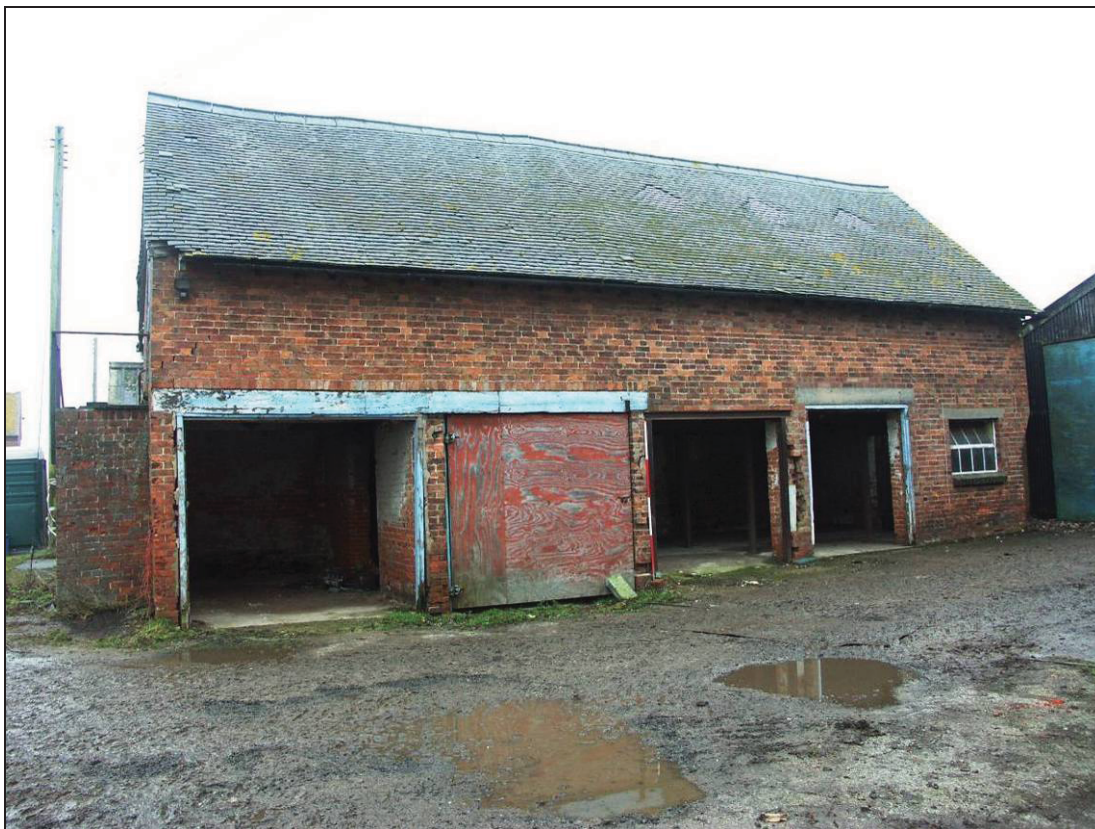
Plate 3: South elevation of Building B
