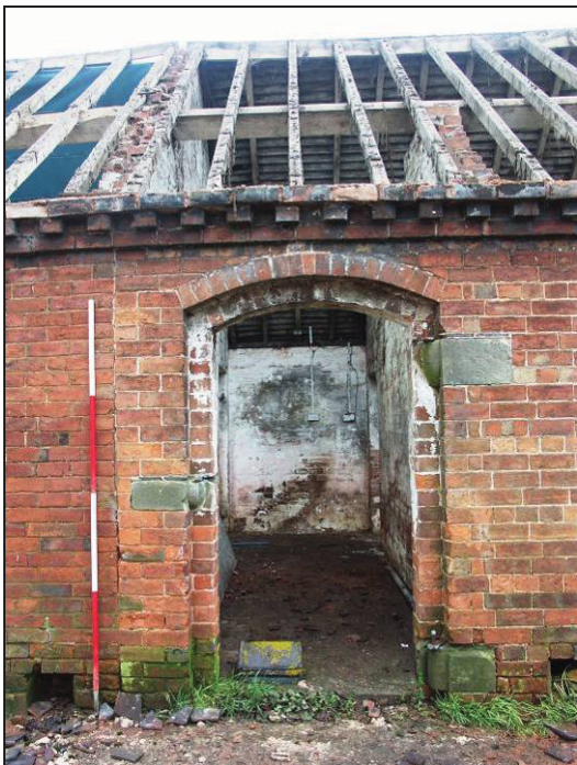
Plate 18: Doorway on the west elevation of Building E
