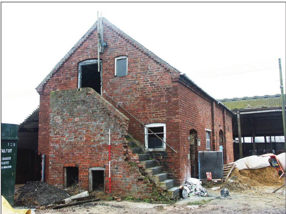
Plate 41: West elevation of Building K
