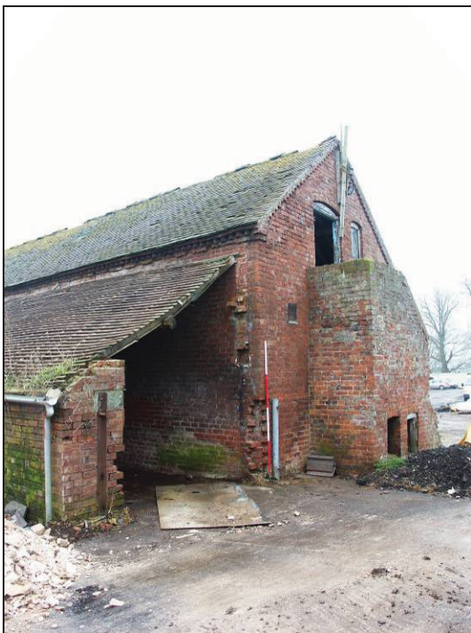
Plate 44: Lean-to on the north elevation of Building K
