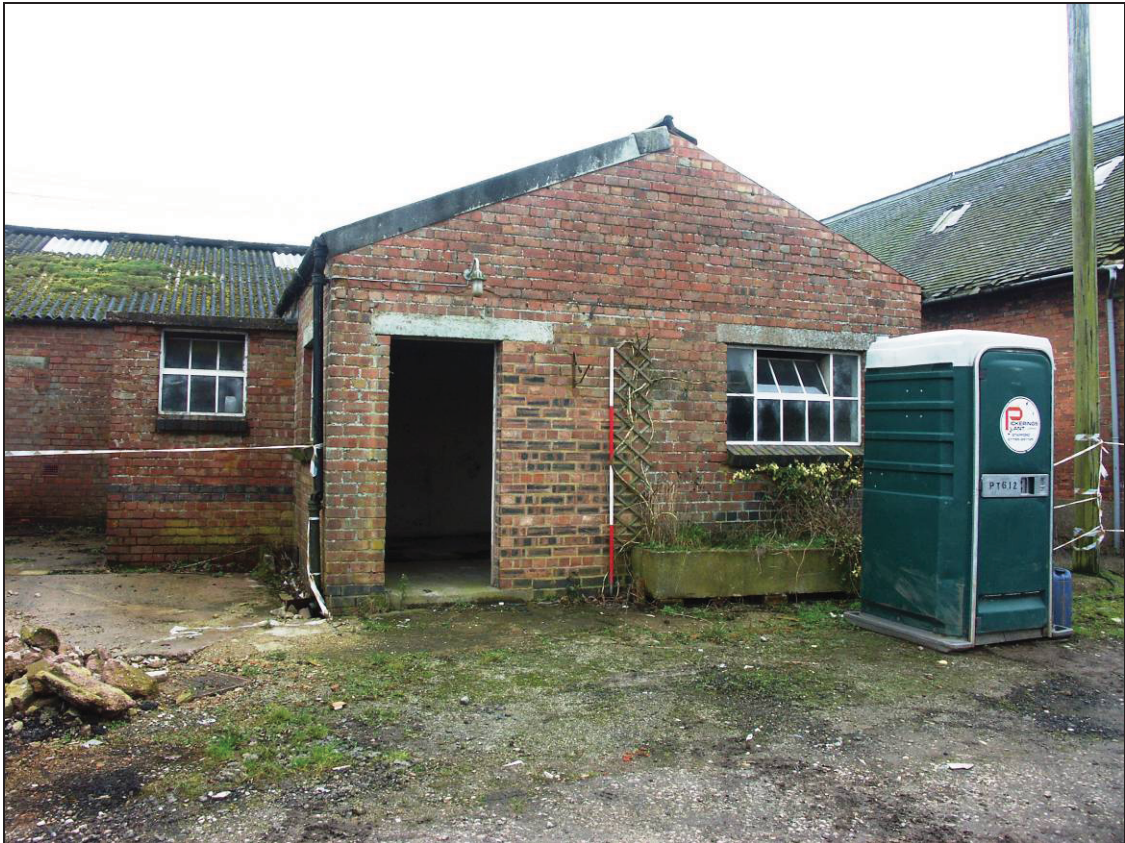
Plate 37: West elevation of Building J
