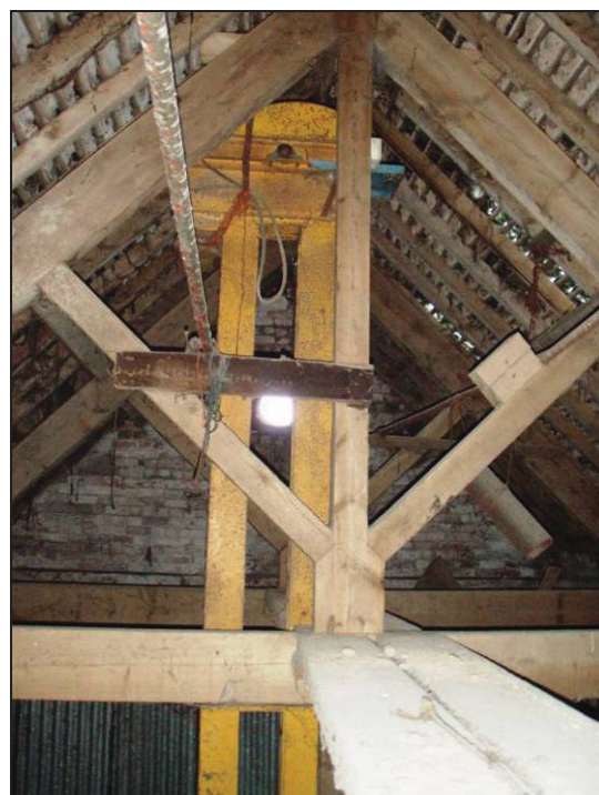
Plate 8: Detail of king-post truss
