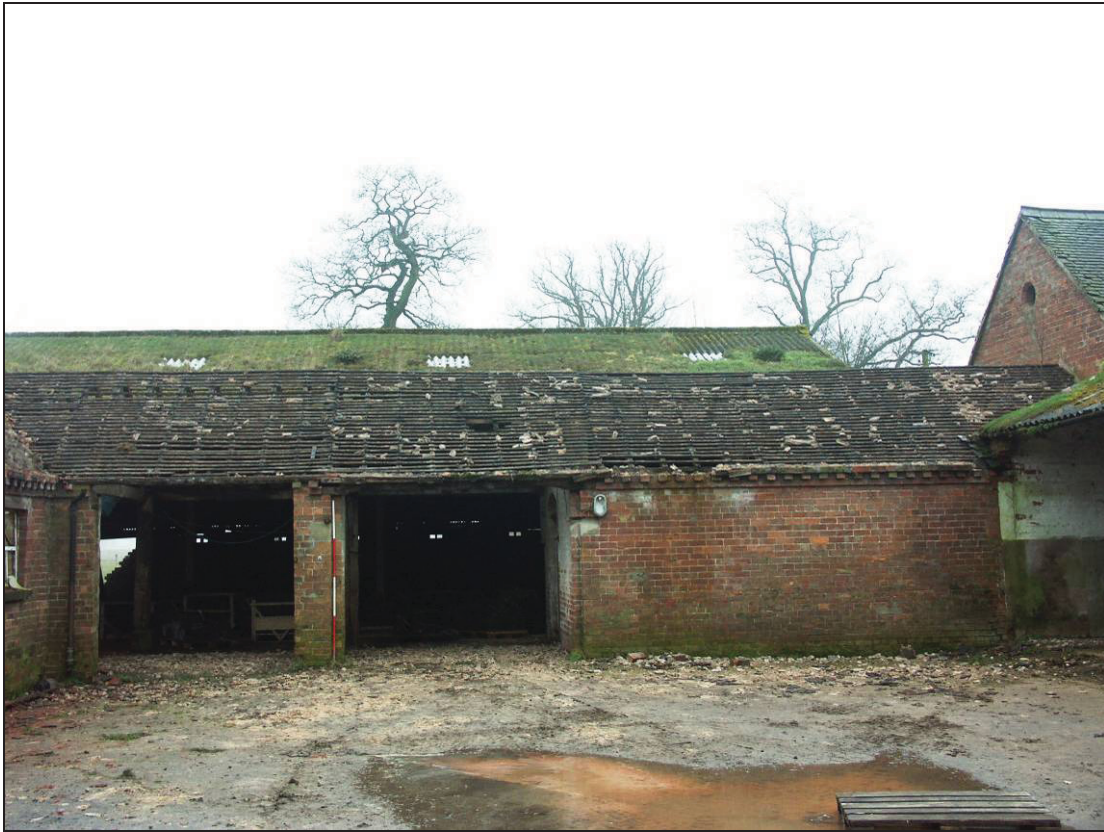
Plate 11: North elevation of Building D
