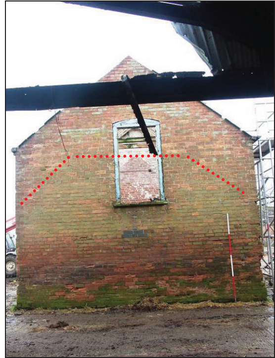
Plate 27: North elevation of Building F showing construction break (red dots)
