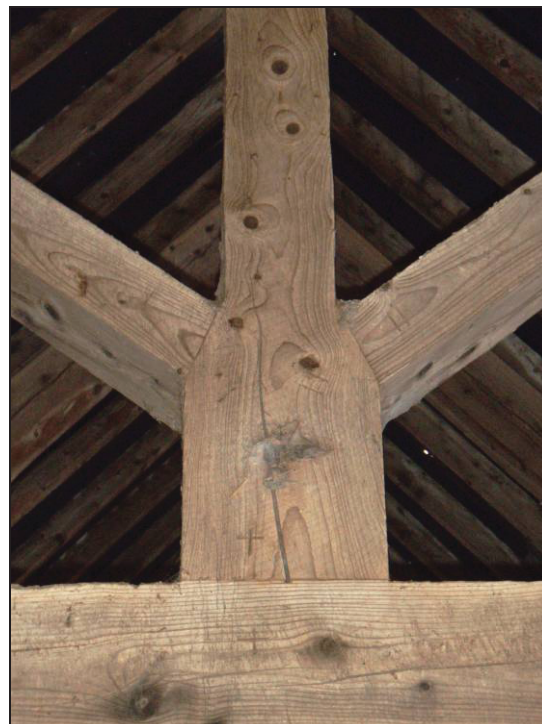
Plate 55: Detail of carpenter's marks on king-post
