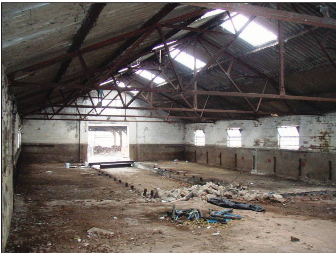
Plate 34: Inside Building H, looking north
