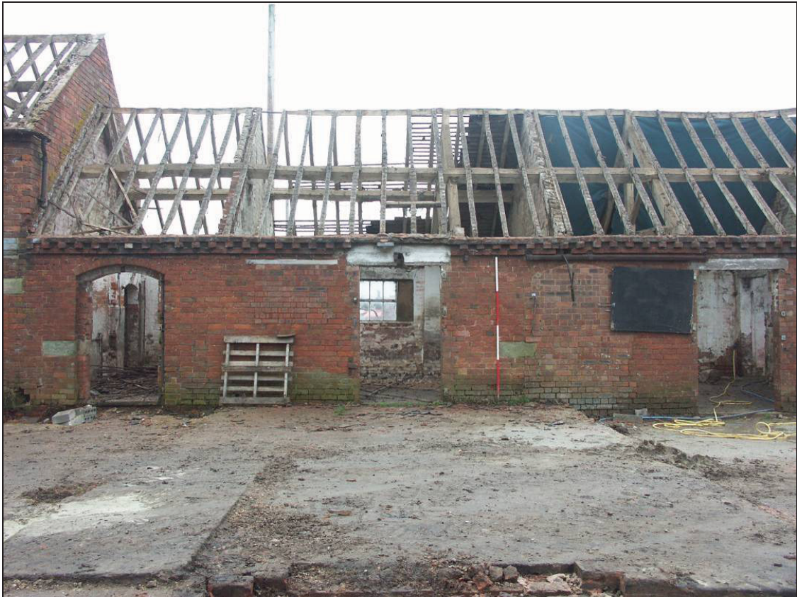
Plate 20: Northern end of west elevation of Building E
