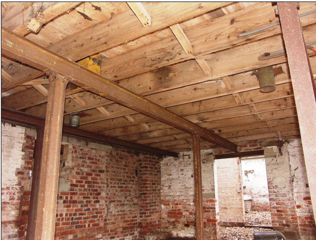
Plate 6: Ceiling with circular apertures for former drive of millstone
