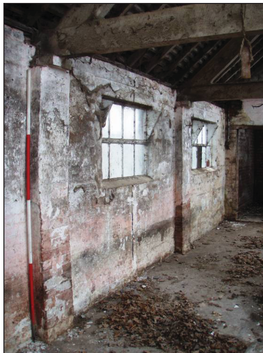
Plate 25: Southern side of Building E
