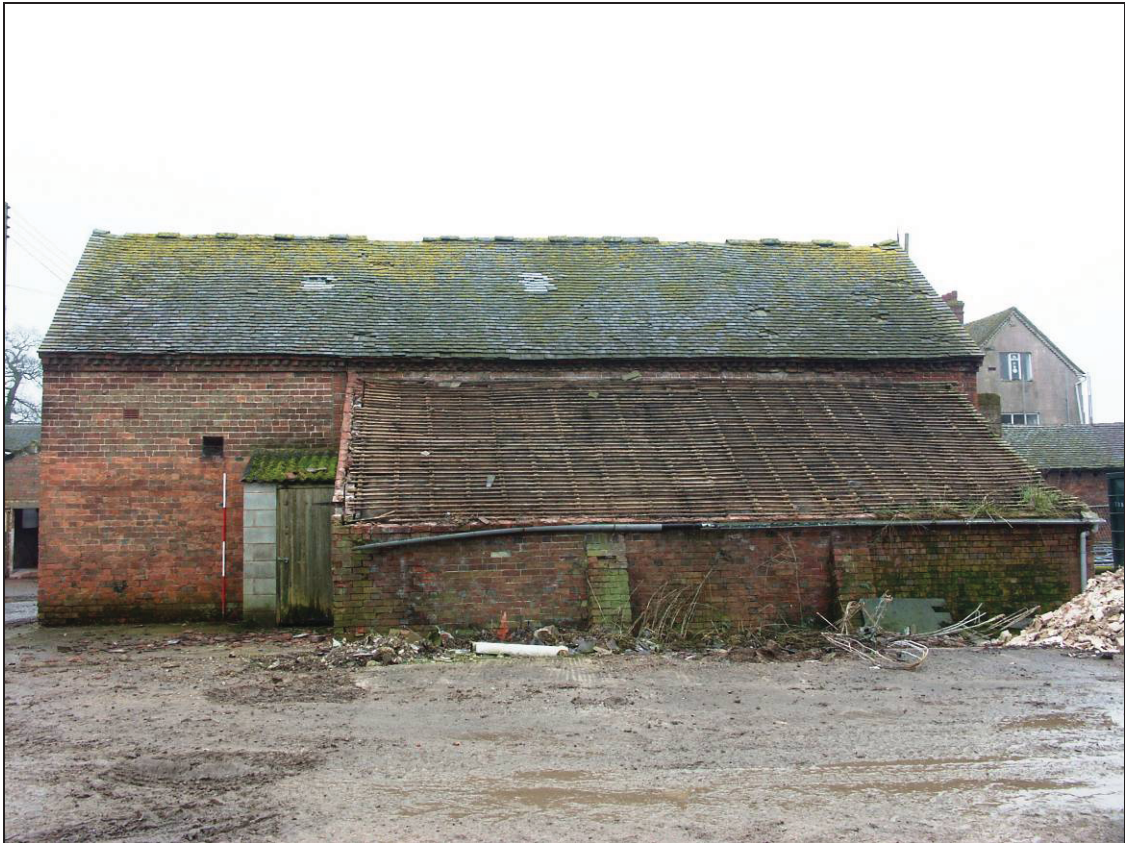
Plate 40: North elevation of Building K
