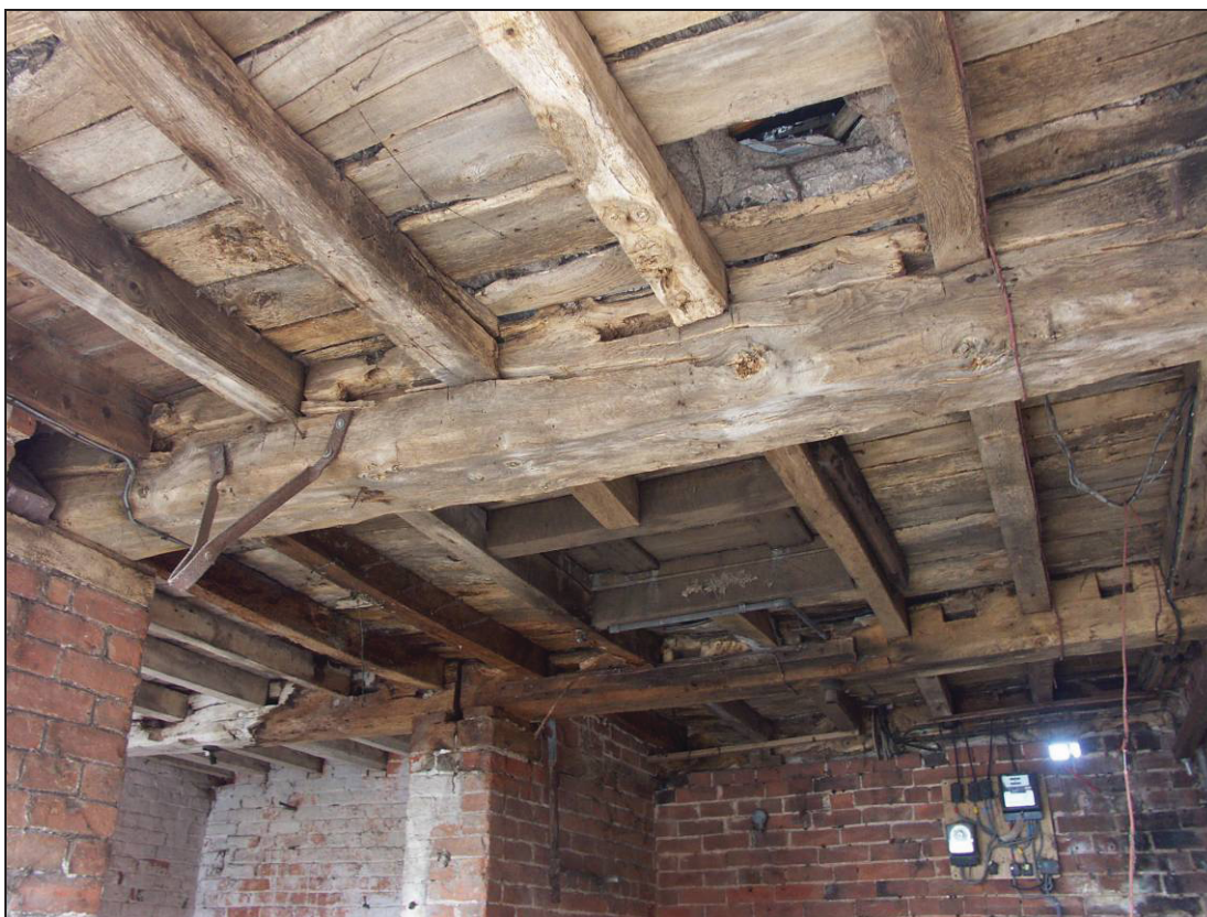
Plate 4: Timber ceiling structure in Building B
