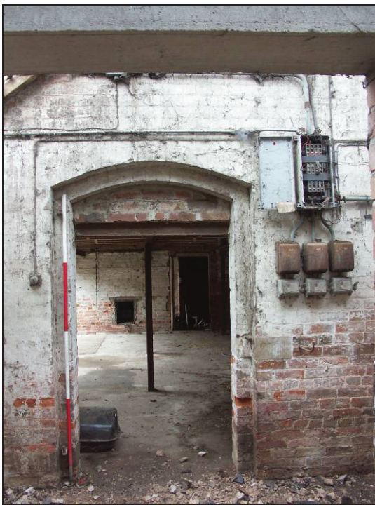
Plate 12: Doorway on the western end of Building D
