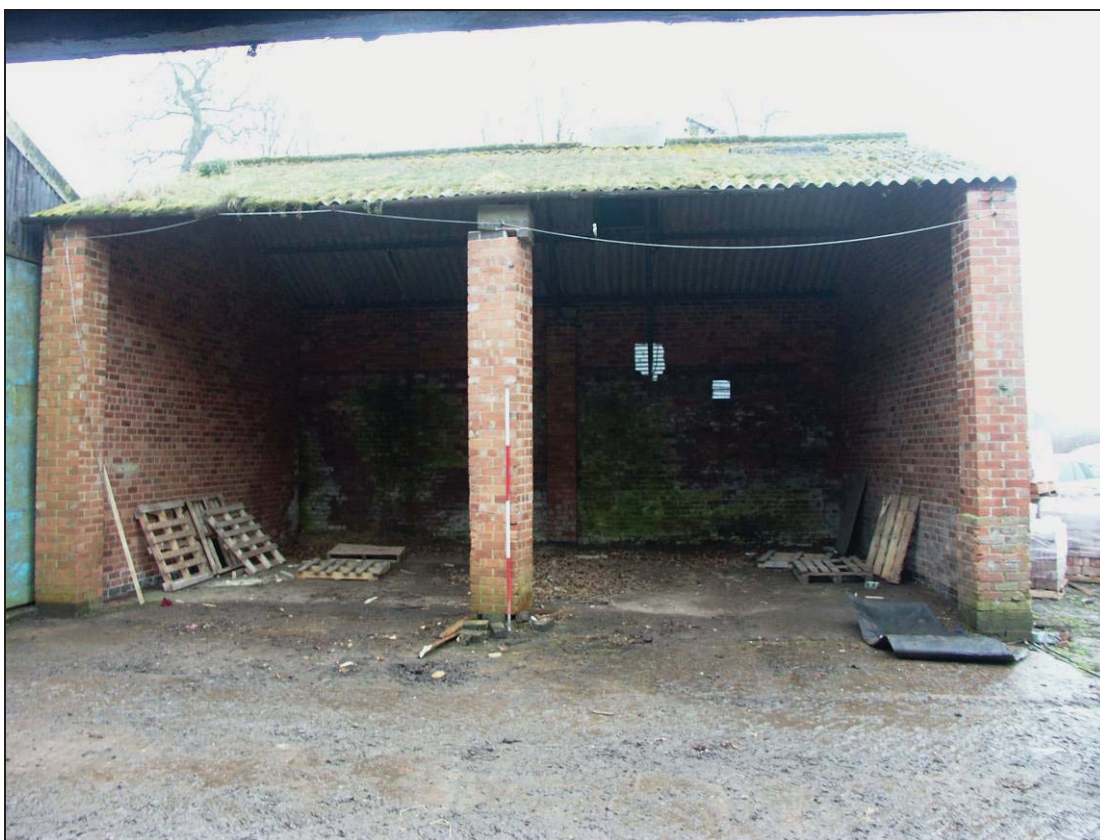
Plate 1: North elevation of Building A with open front
