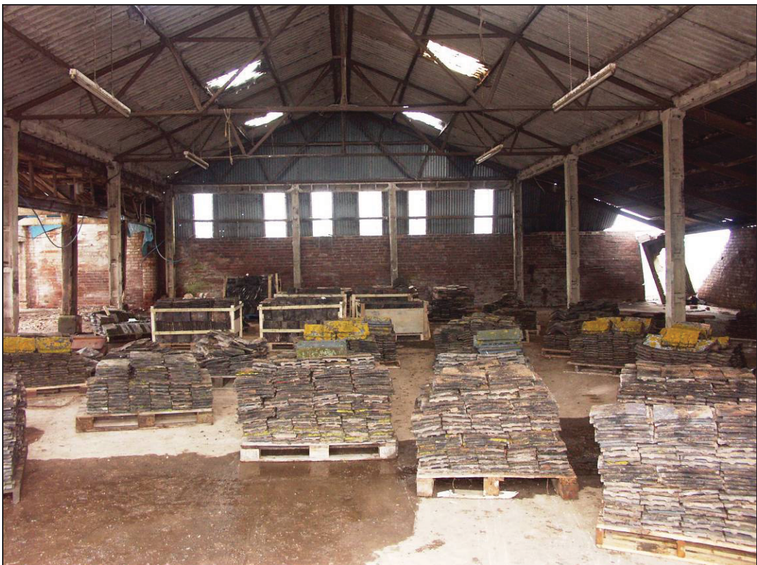
Plate 10: Inside Building C, looking east
