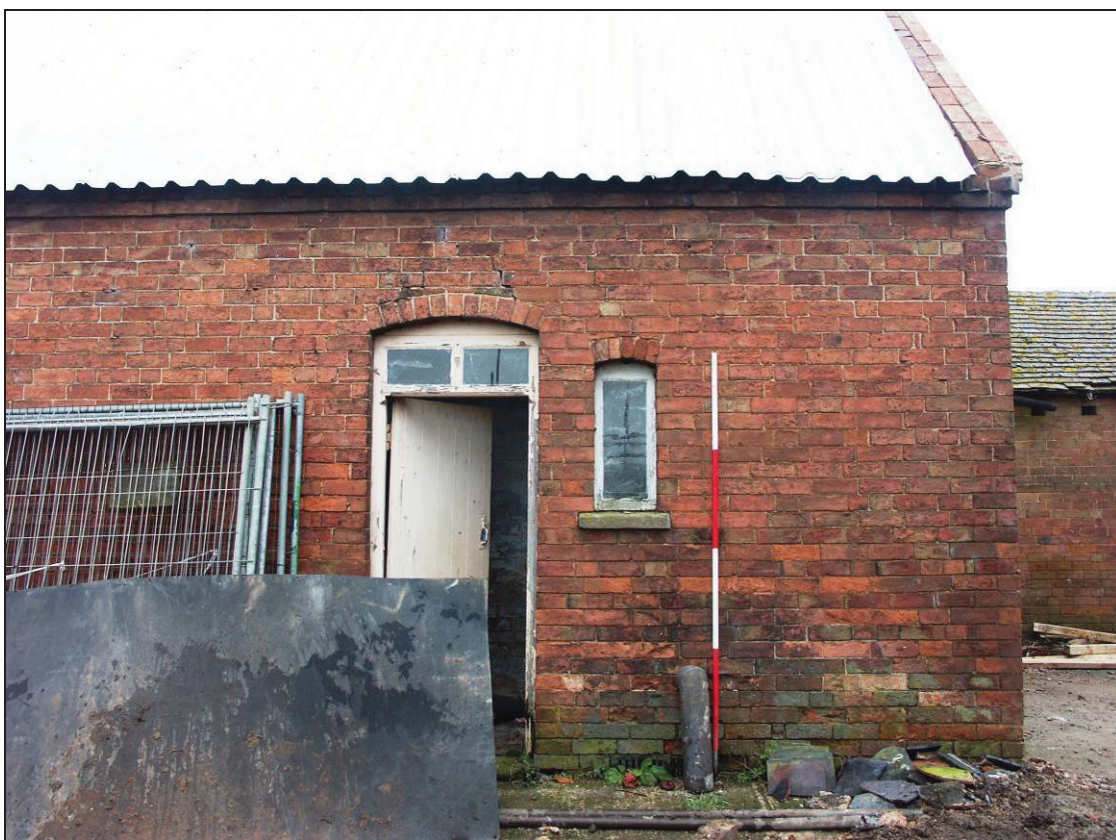
Plate 53: Eastern bay on the south elevation of Building M
