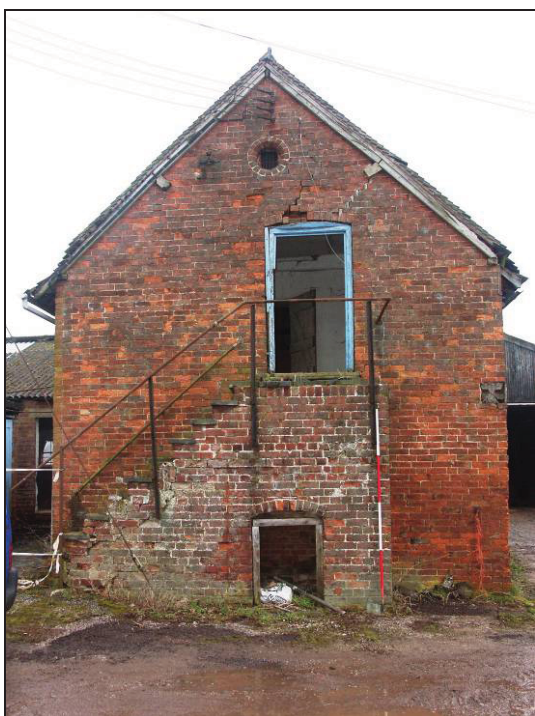
Plate 7: West elevation of Building B
