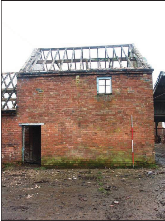
Plate 26: West elevation of Building F
