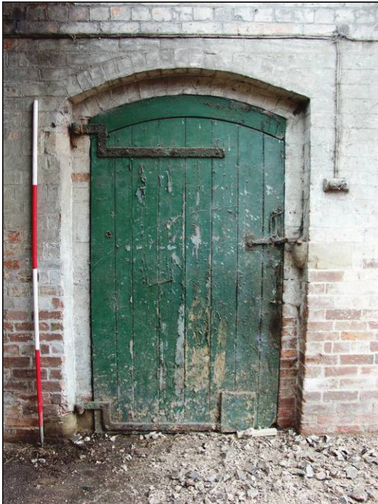
Plate 14: Doorway of the western side of Building D
