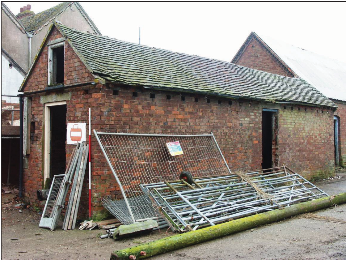
Plate 48: North elevation of Building L
