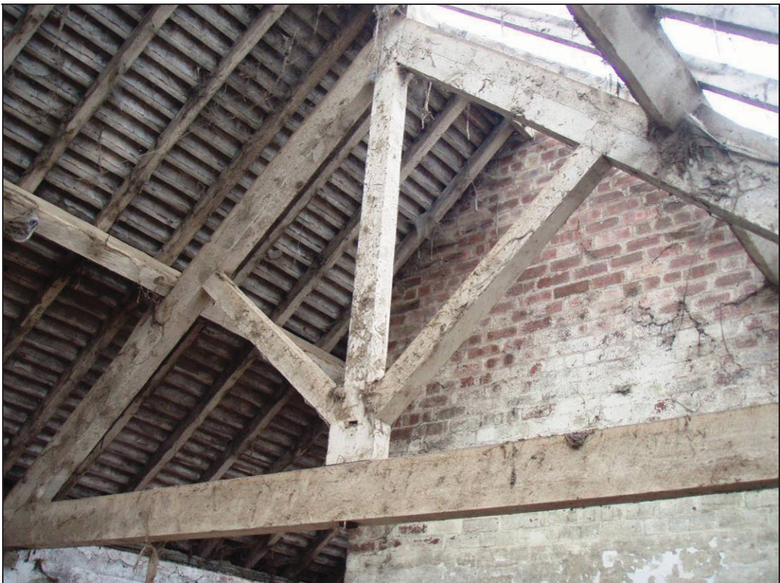
Plate 23: Timber king-post truss within the southern side of Building E
