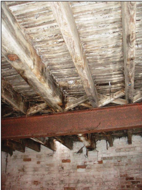
Plate 29: Ceiling structure of Building F
