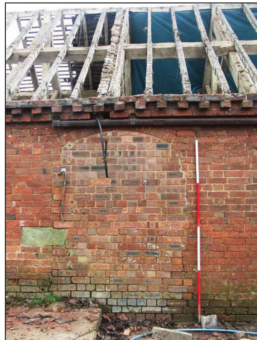
Plate 19: Blocked-up doorway of Building E
