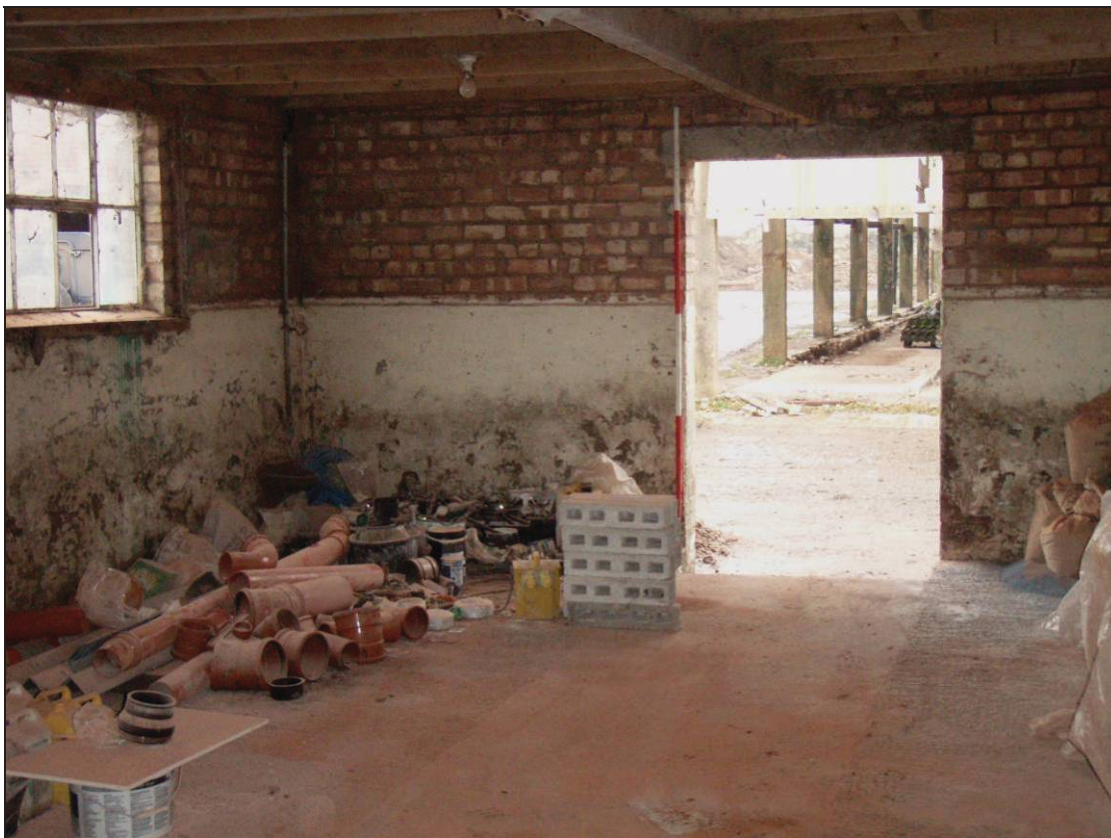
Plate 36: Inside Building I, looking north
