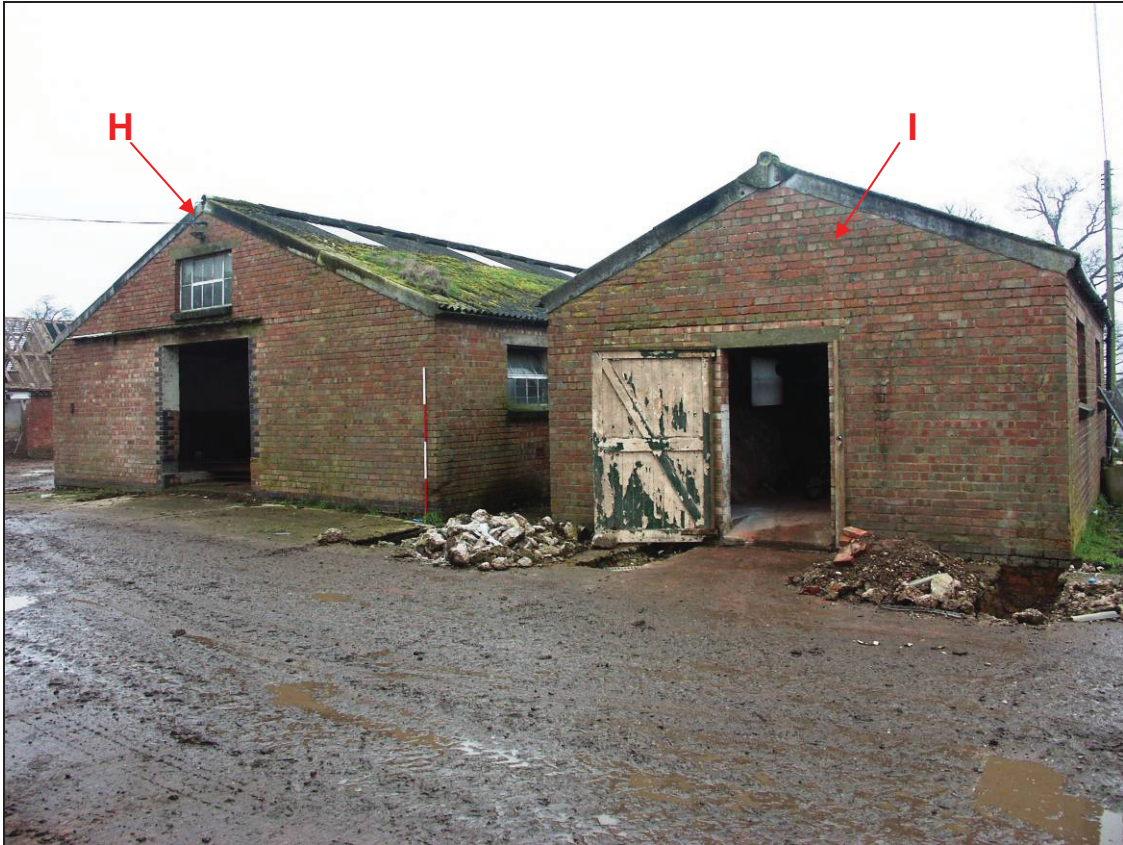
Plate 32: North elevation of Building H on the left and Building I on the right
