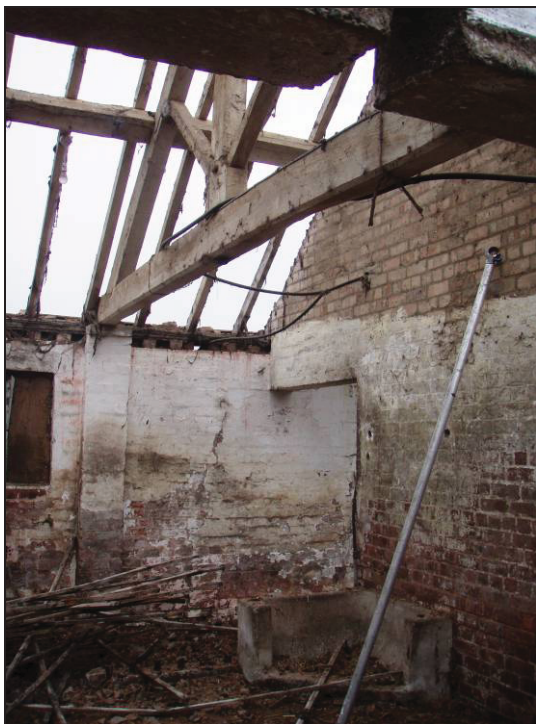
Plate 24: Northern side of Building E, looking south
