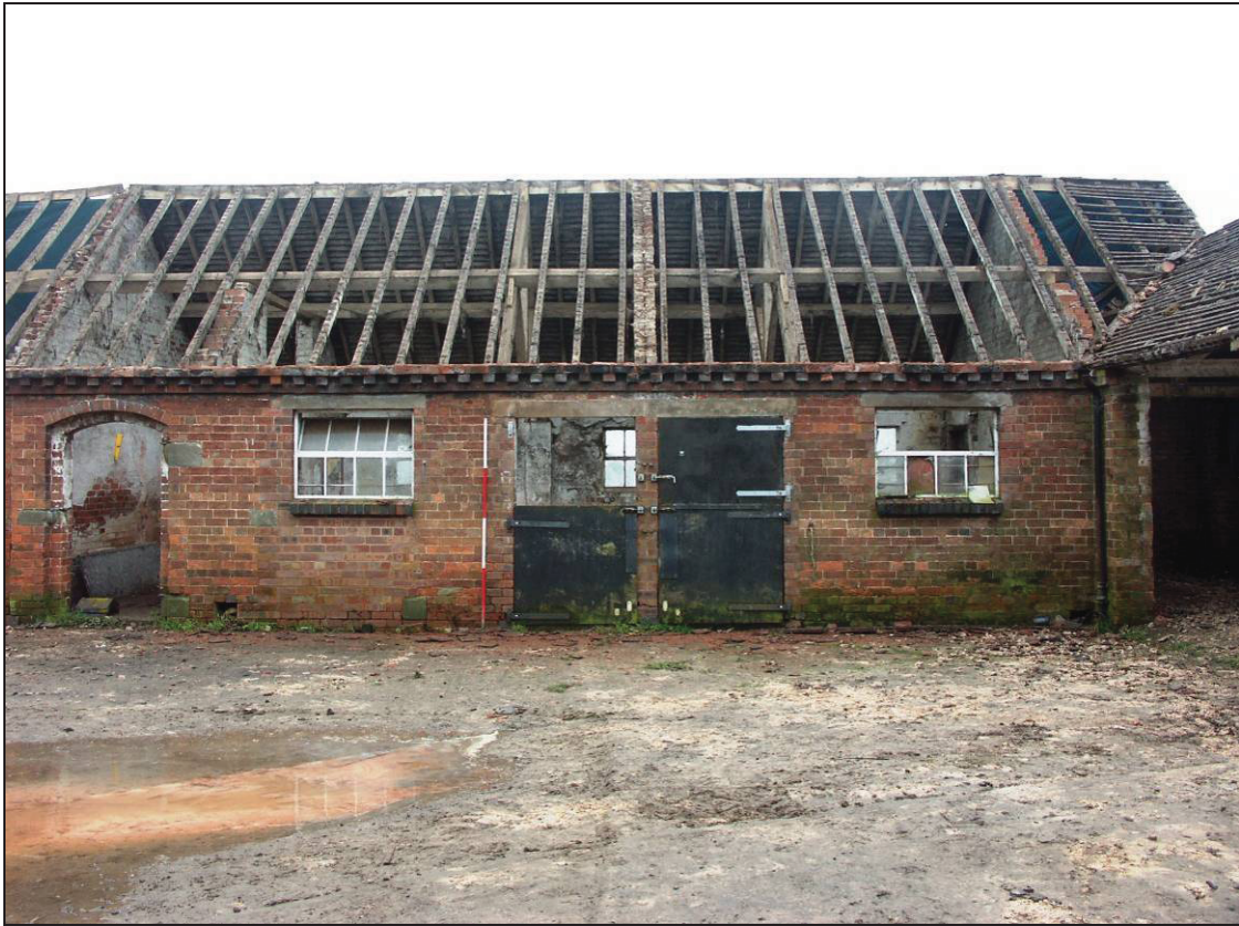
Plate 17: Southern end of the west elevation of Building E
