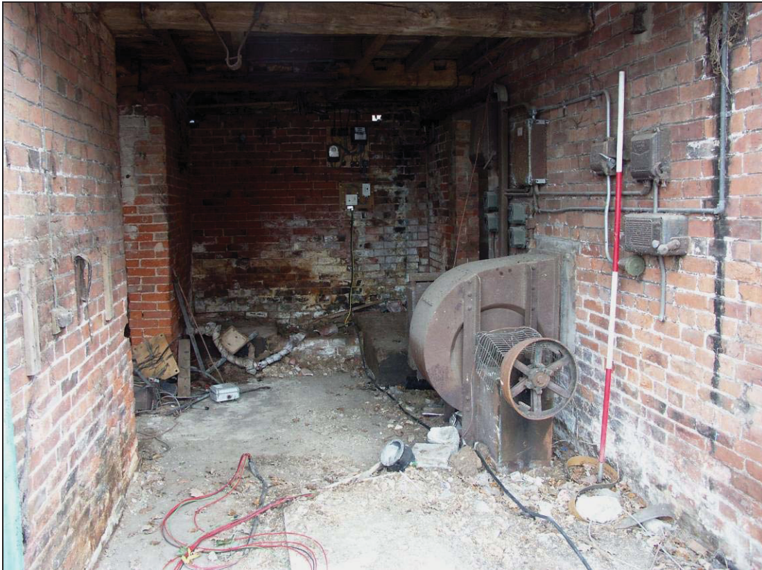
Plate 5: Electric winnower threshing machine on the ground floor of Building B
