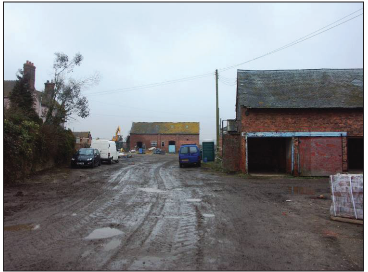
View of the central lane of Bagot's Bromley Farm, looking north
