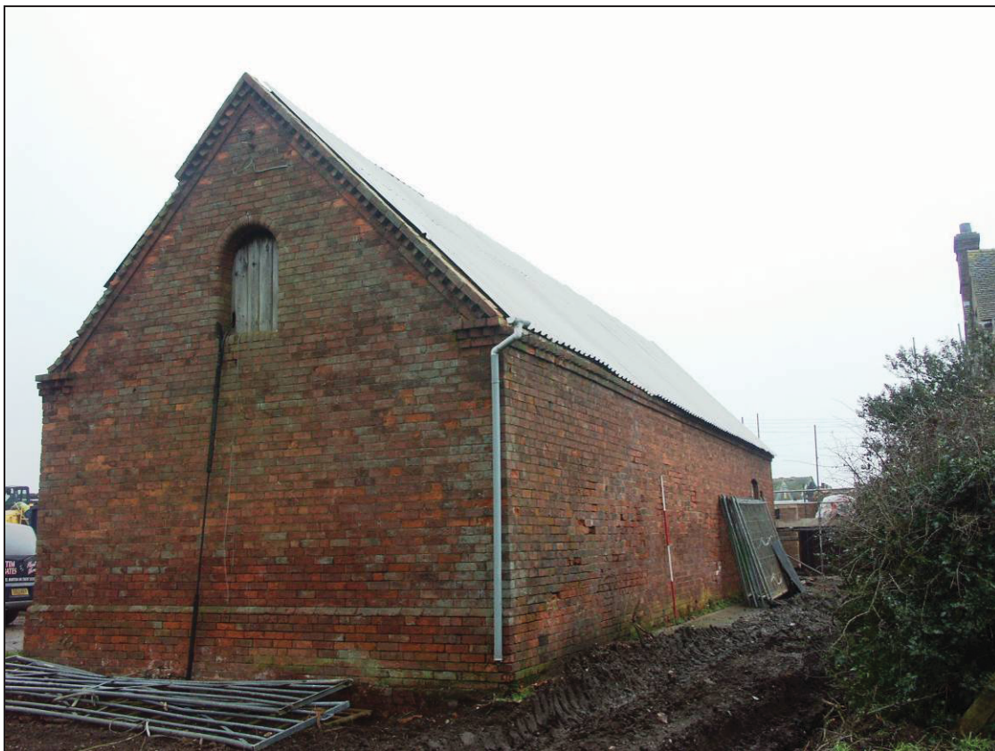
Plate 52: West and south elevations of Building M
