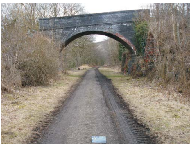
Figure 27: Feature 26- Bridge Near Litton Tunnel. Scale = 1m.
