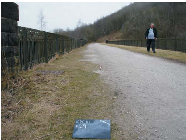
Figure 30: Feature 29- Miller's Dale Viaduct (South). Scale = 1m.
