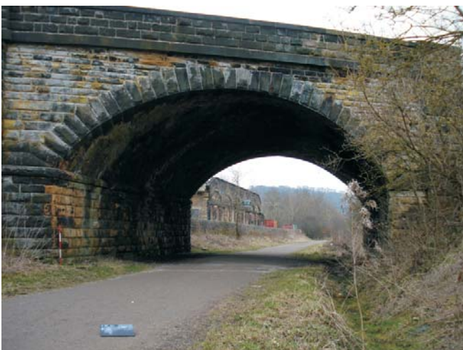
Figure 17: Feature 16- Bridge. Scale = 1m.
