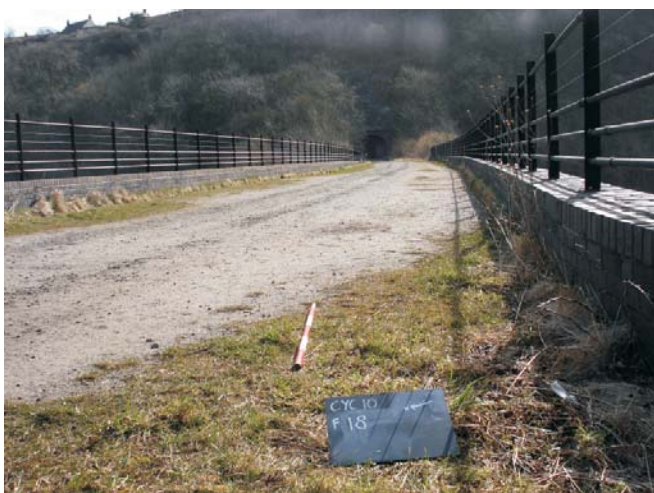
Figure 19: Feature 18- Monsal Viaduct. Scale = 1m.
