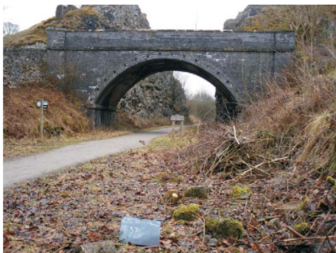
Figure 38: Feature 37- Bridge. Scale = 1m,
