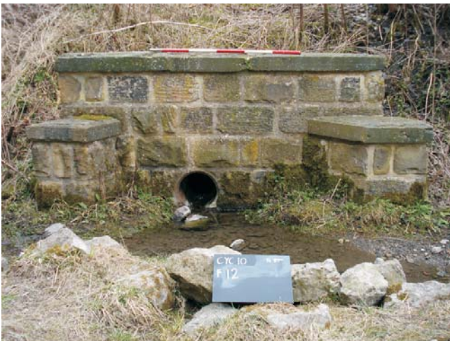
Figure 13: Feature 12- Culvert. Scale = 1m.
