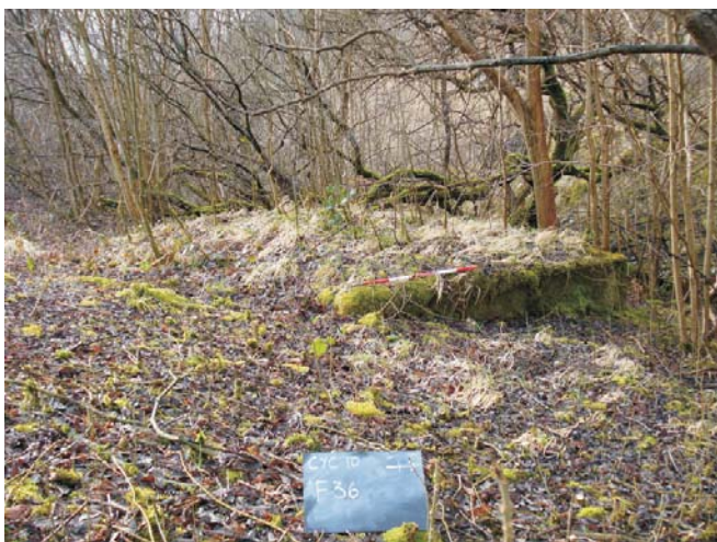
Figure 37: Feature 36- Concrete structure, line side hut. Scale = 1m.
