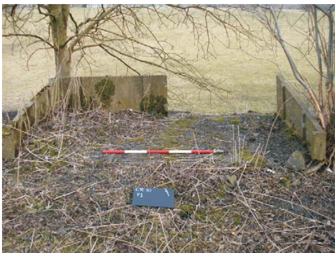
Figure 2: Feature 1- Concrete structure, line side hut. Scale = 1m.
