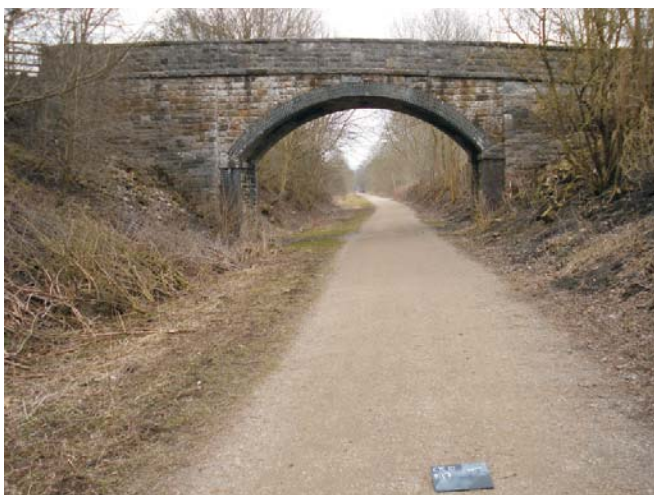
Figure 18: Feature 17-Bridge. Scale = 1m.
