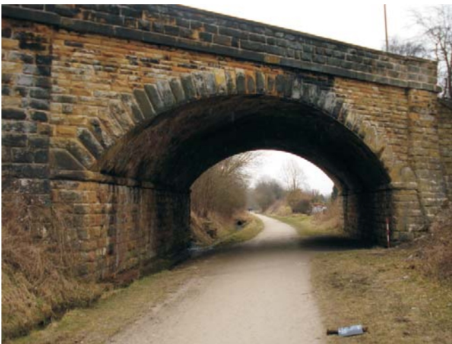
Figure 16: Feature 15-Bridge. Scale = 1m.
