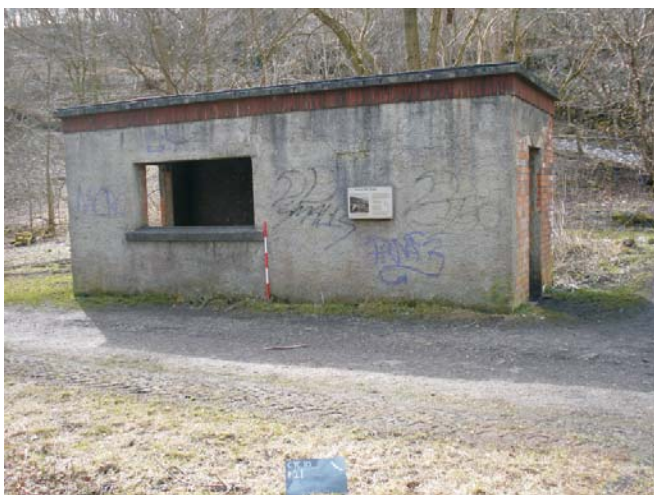
Figure 22: Feature 21- Brick Structure Near Monsal Rail Station. Scale = 1m.
