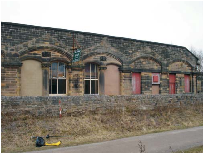
Figure 11: Feature 10-Hassop Railway Station. Scale = 1m.
