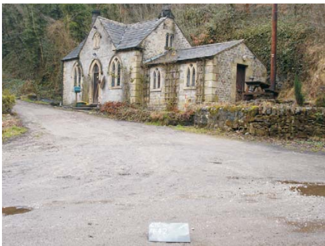
Figure 43: Feature 42- Lodge to Picton Hall. Scale = 1m.
