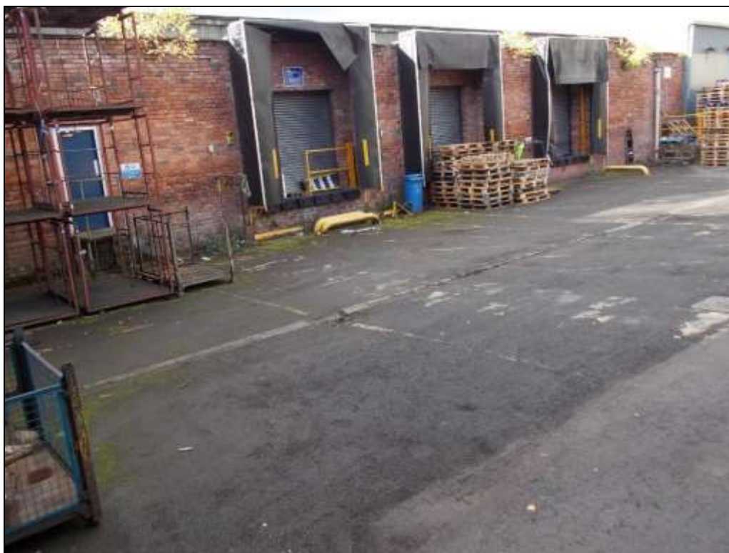
Figure 67: Eastern elevation of Building G facing onto the backyard.
