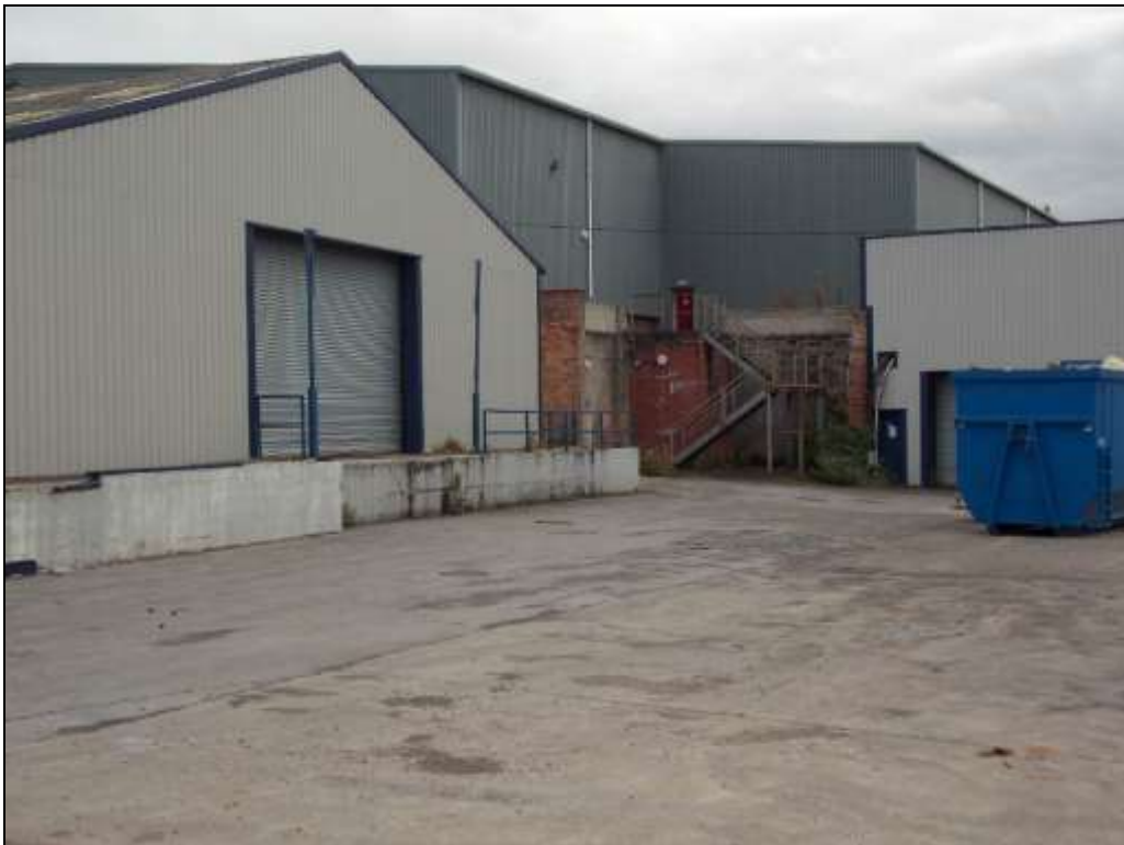
Figure 46: Southern wing of Building A with a raised concrete platform.
