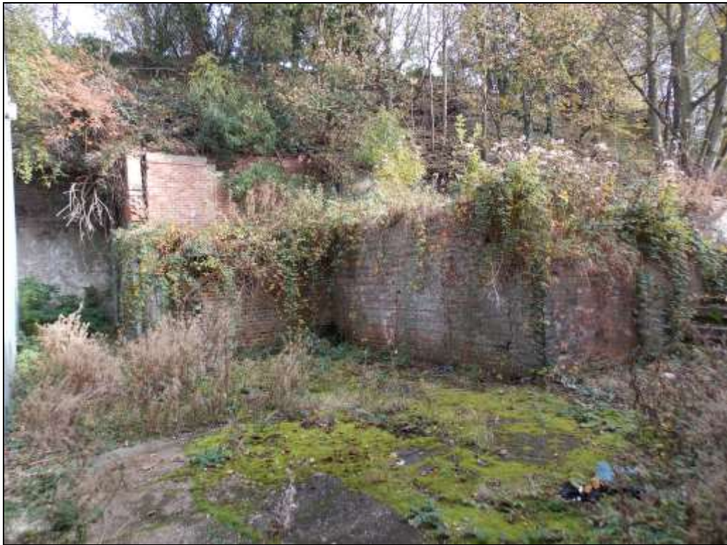
Figure 35: View east of brick remains, which potentially represent the extent of the structure in 1968. A pair of stairs is indicated by the arrow.
