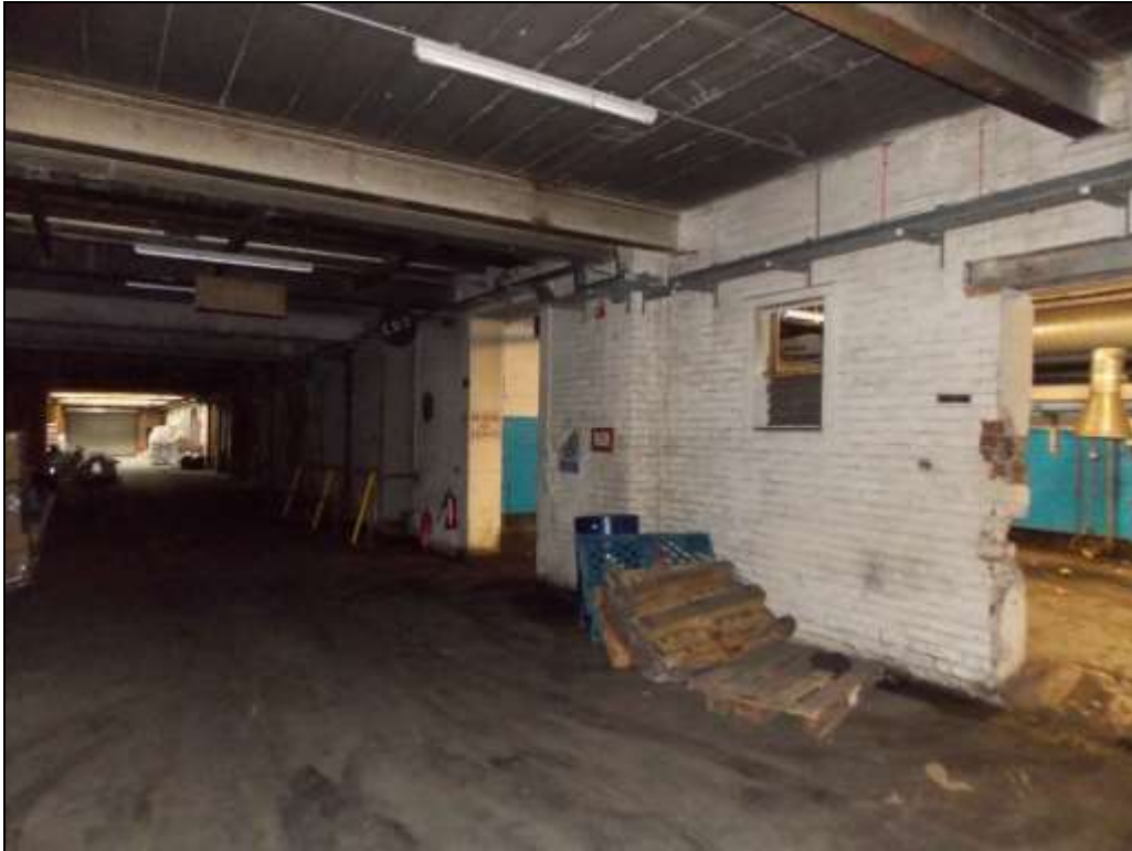
Figure 72: Internal view of the basement of Building H.
