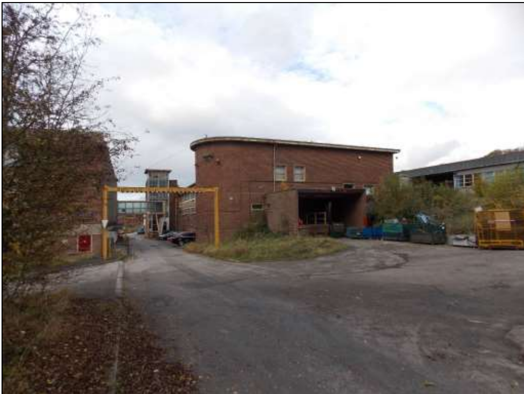
Figure 80: Southern end of Building K with the cross-wing facing onto the central lane.
