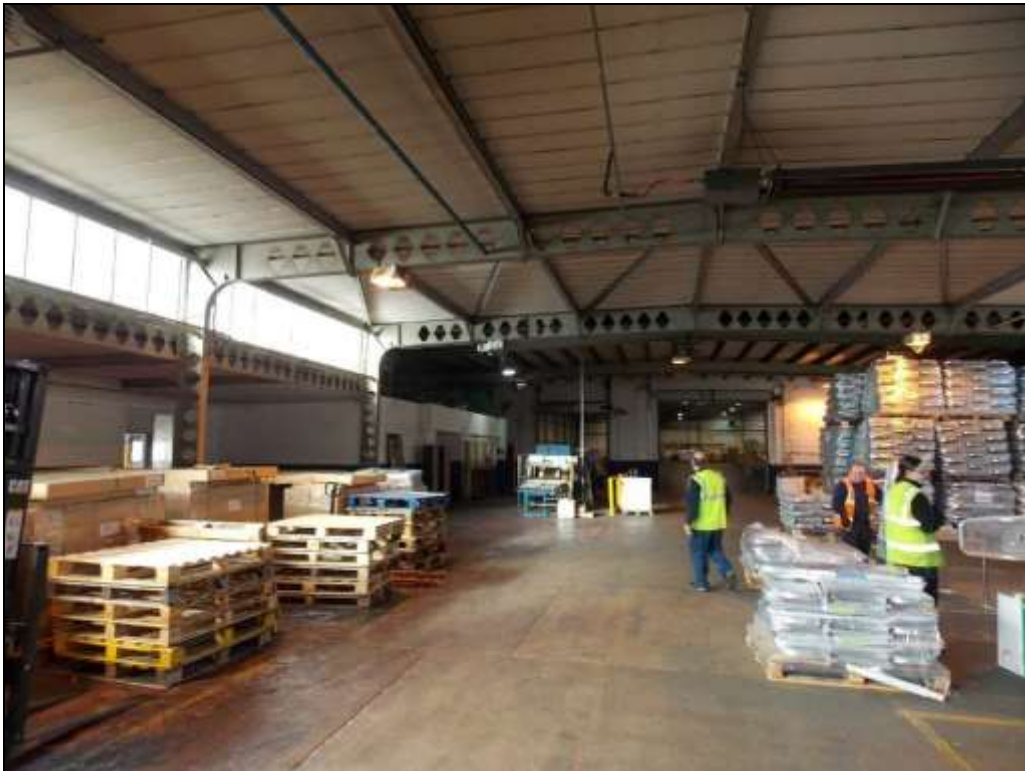
Figure 69: Internal view of Building G.
