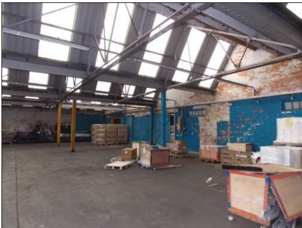
Figure 78: North-light roof of Building J.
