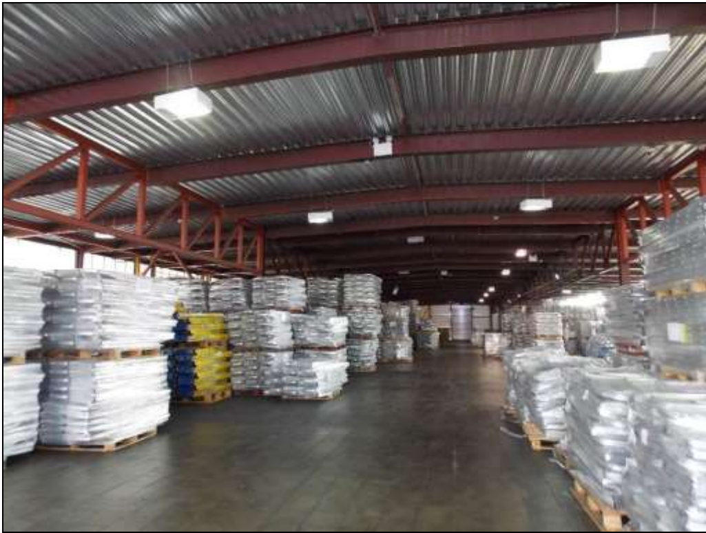
Figure 65: Internal view of Building F.
