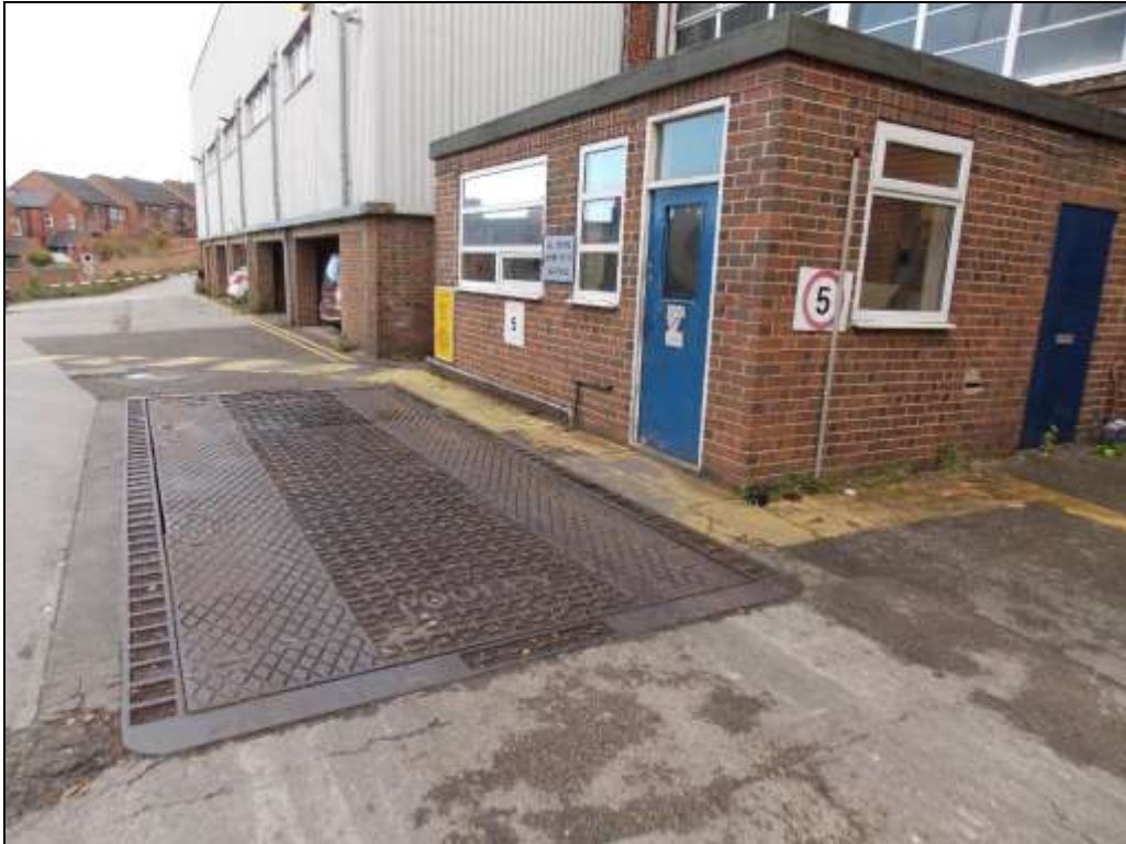
Figure 82: Gate house and adjacent weighing bridge.
