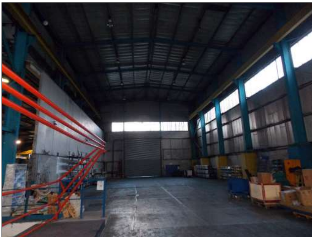
Figure 51: Internal view of Building C.
