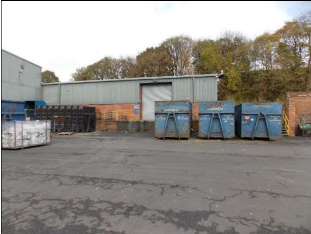
Figure 62: General view of Building E, looking north-east.
