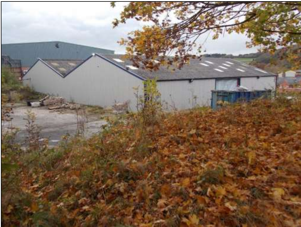
Figure 45: General view of Building A, looking south.
