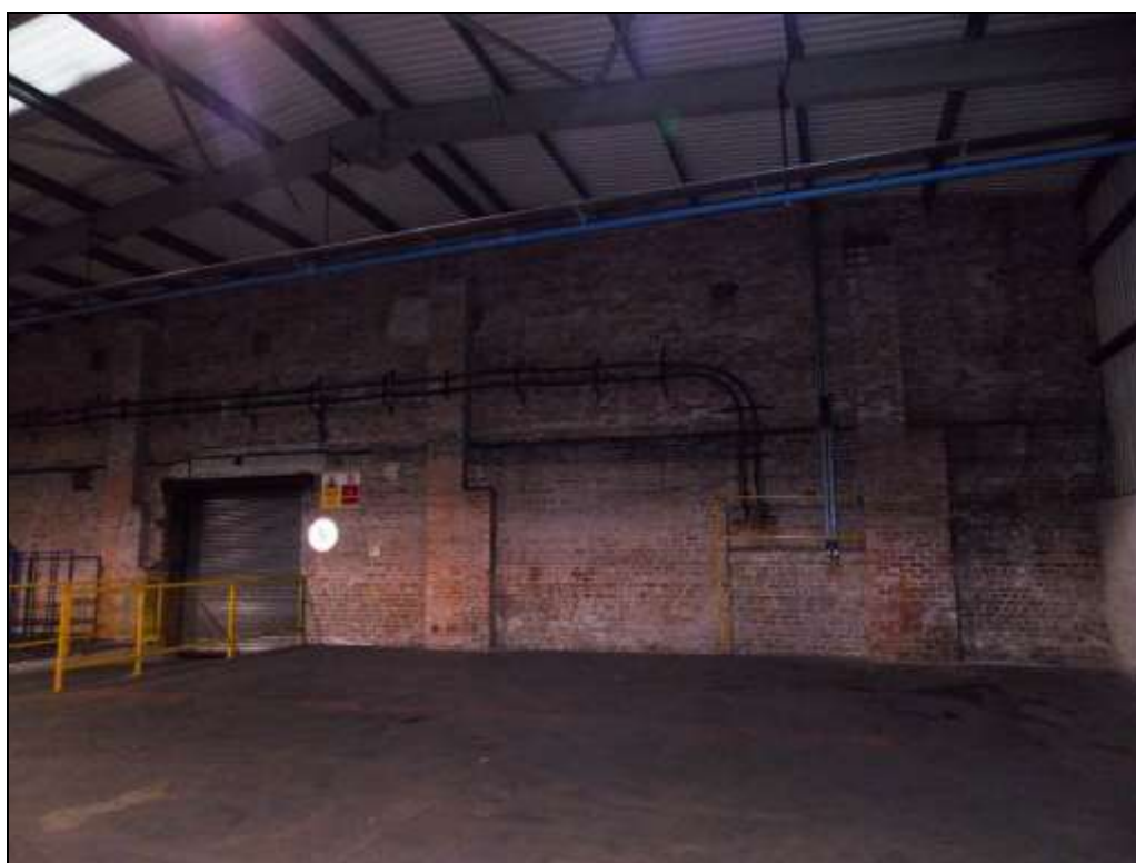
Figure 60: Internal view of the northern brick wall.
