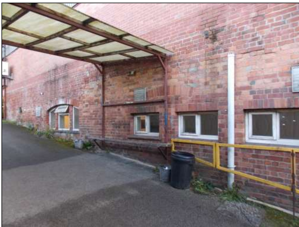
Figure 58: Northern elevation with further arched-heads of former windows.
