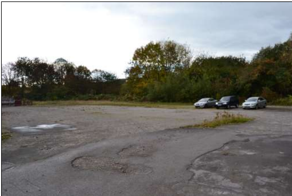
Figure 44: View south-west across the car park.
