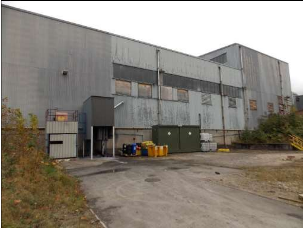
Figure 48: General view of Building B, looking north-east.
