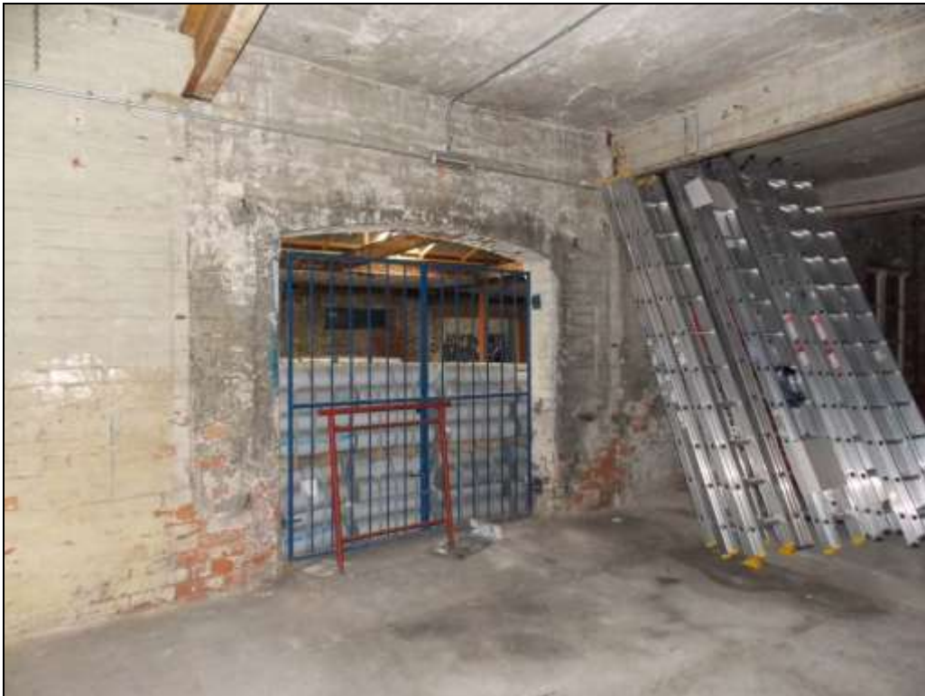
Figure 75: Detail of the doorway viewed from inside the adjacent Building D.
