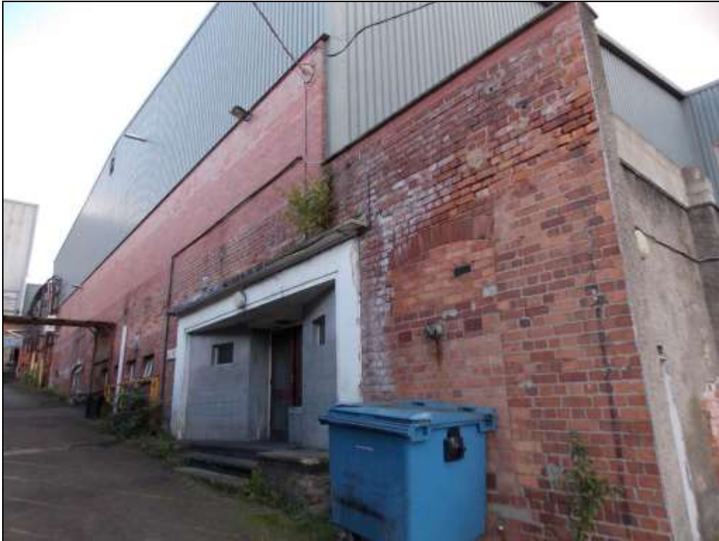
Figure 54: Northern elevation of Building D with blocked-up arched opening.
