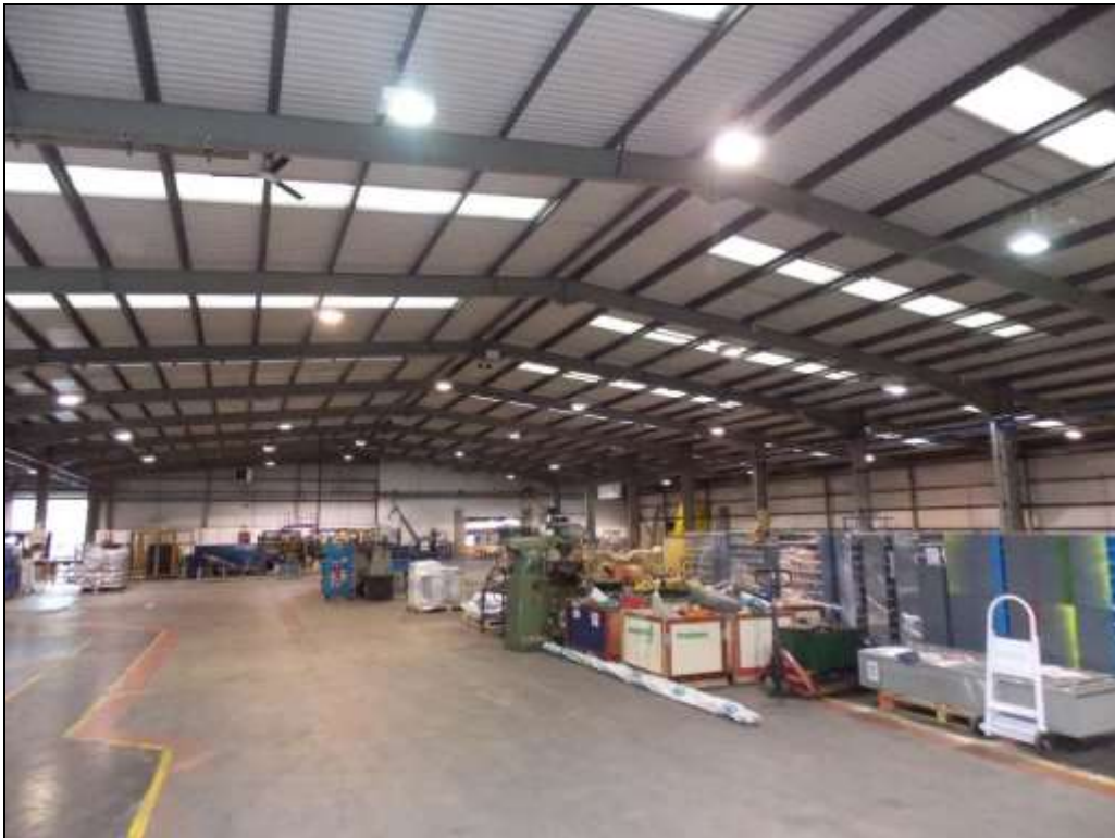
Figure 61: General internal view of Building D.
