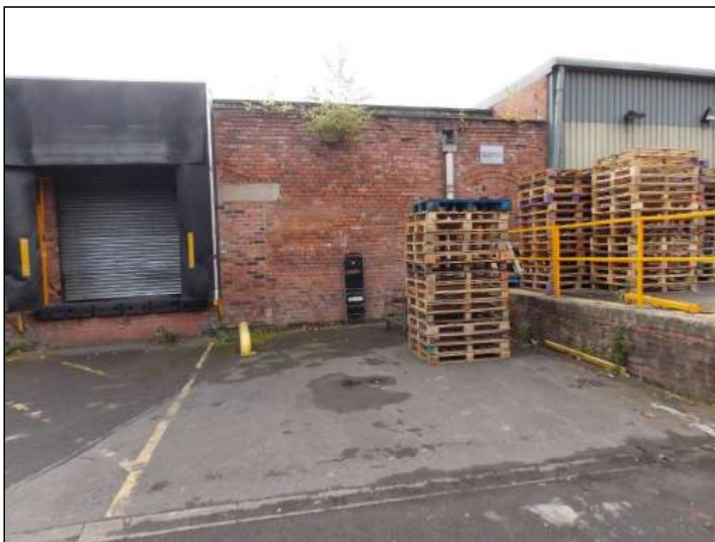
Figure 68: Blocked-up arched openings within the eastern elevation.
