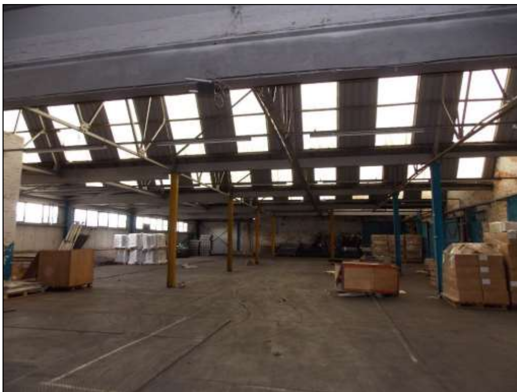
Figure 77: Internal view of Building J.
