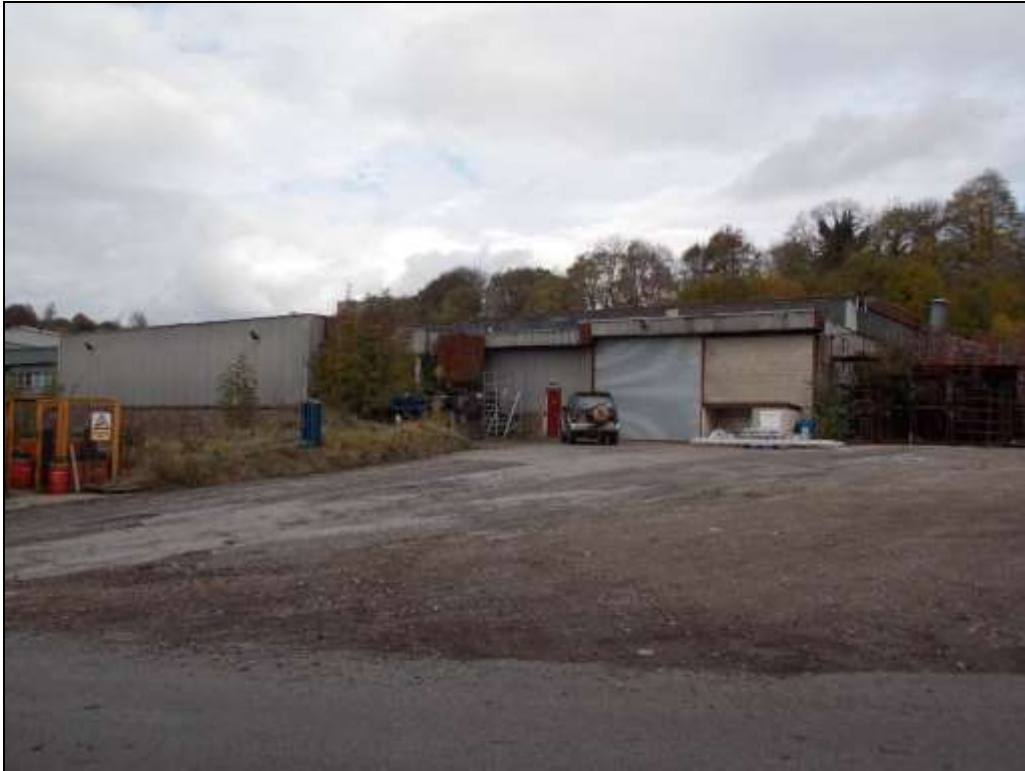
Figure 66: General view of Building G, looking north-east.
