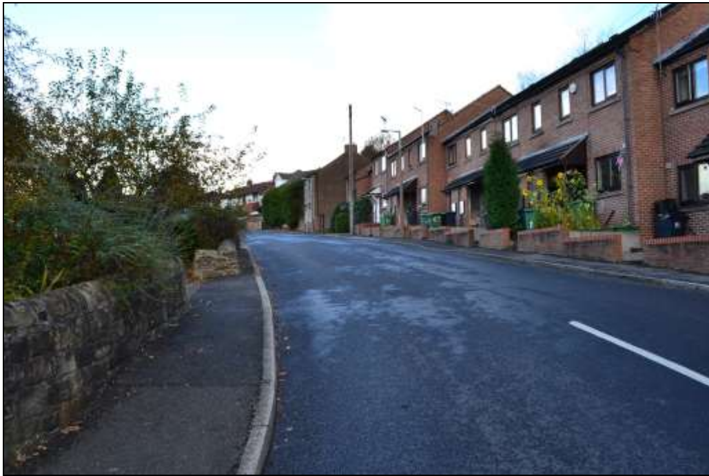
Figure 97: View north along Becksitch Road within the WHS Buffer Zone.
