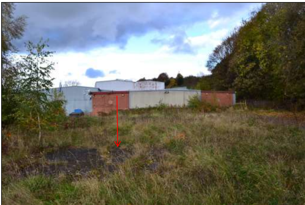
Figure 38: View north of one of the concrete platforms to the south of Building E (arrow).
