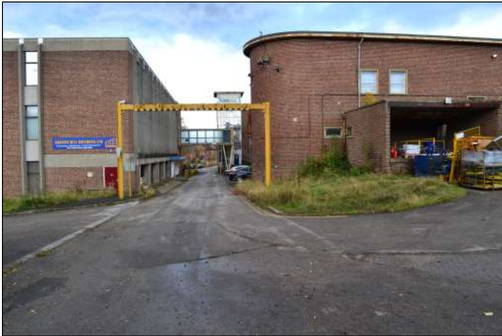
Figure 43: View north of the access road running between Buildings K and M. The entrance to the car park is to the left.
