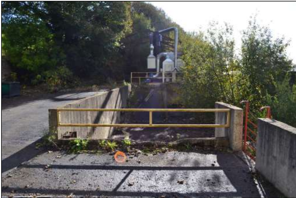
Figure 33: View south-east across the eastern boundary of the PDA, showing the steel structure in the background.
