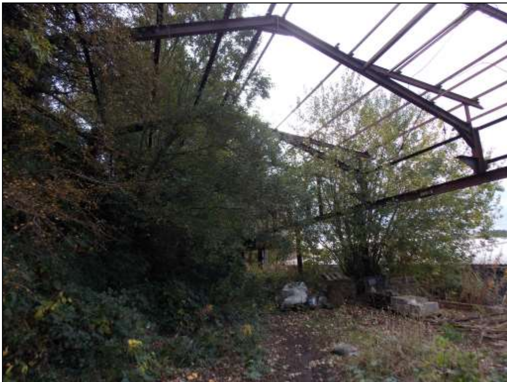
Figure 34: View south-east from within the overgrown steel structure.
