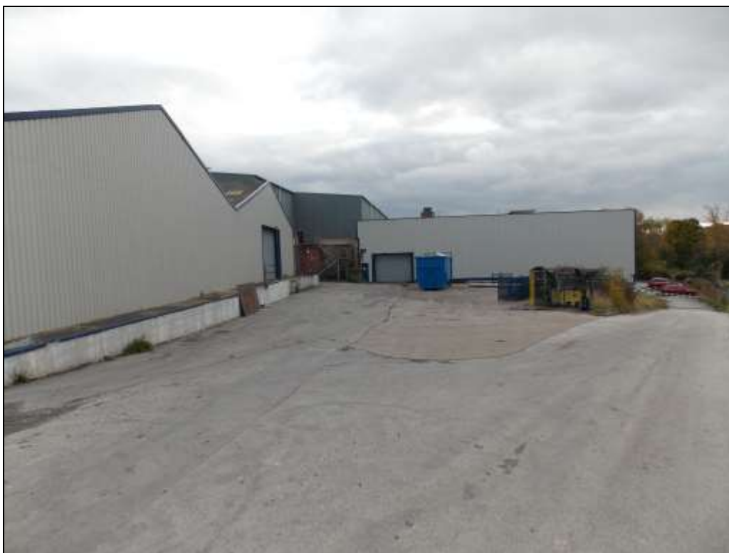
Figure 26: View south of the former site of a building, adjacent Buildings A and J.
