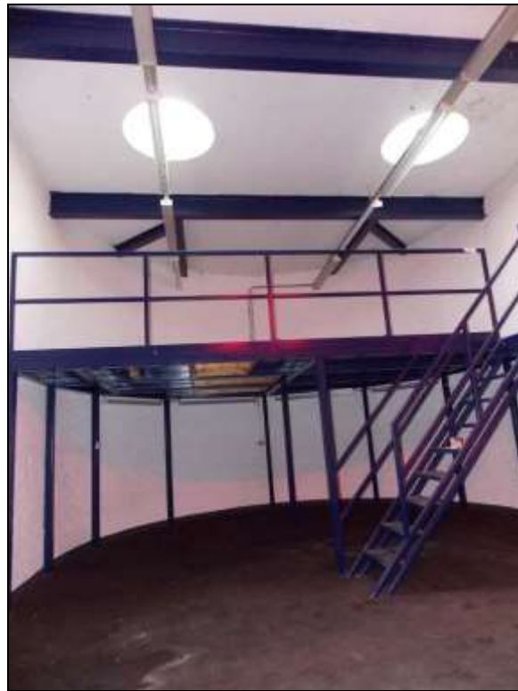
Figure 88: Detail of the curved wall of Building K and circular skylights.
