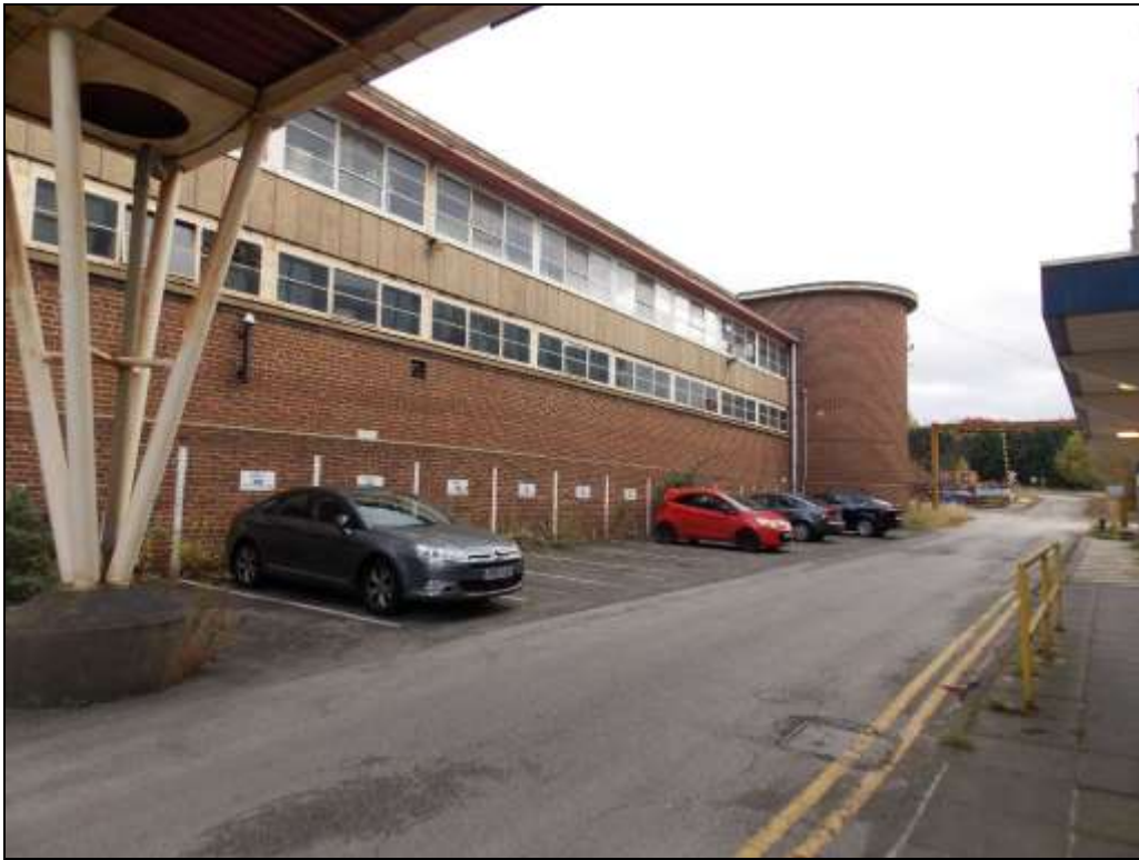
Figure 79: General view of Building K, looking south-east.
