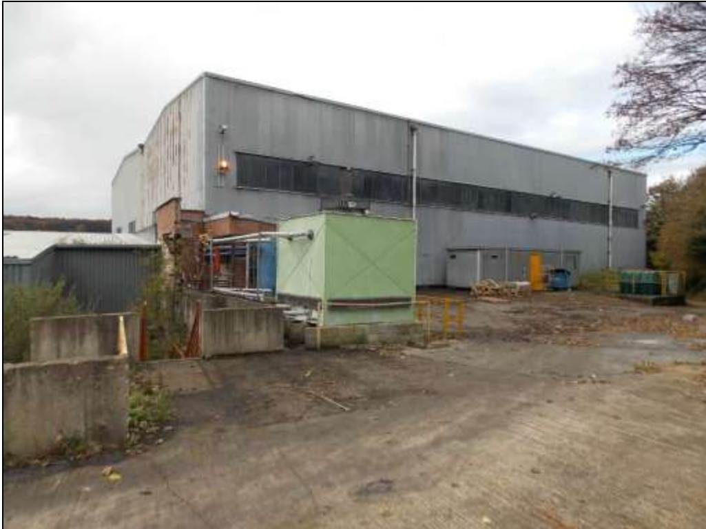
Figure 50: General view of Building C, looking west.
