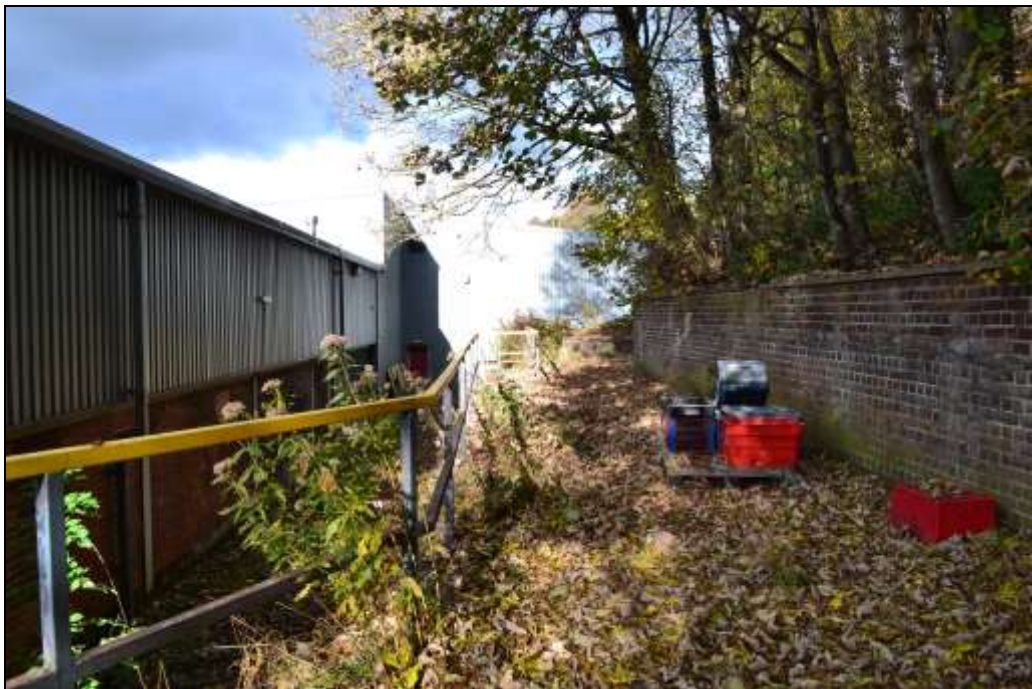
Figure 36: View north-west along the eastern boundary of Building E. The brick retaining wall is shown to the right.
