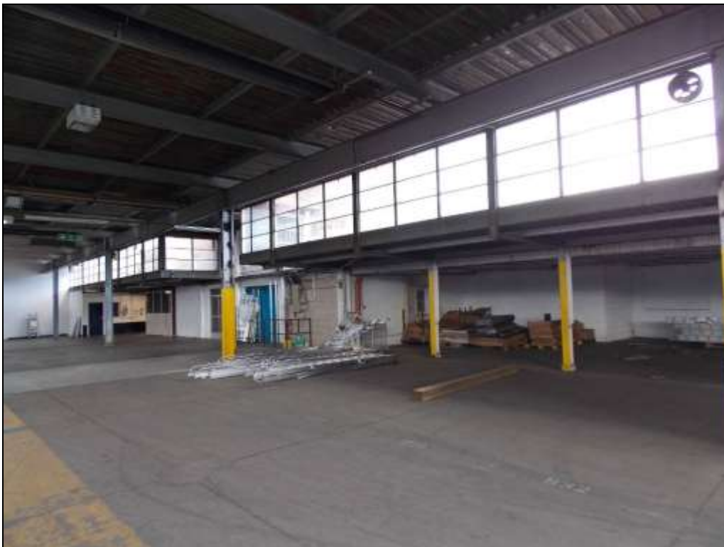
Figure 84: Internal view of Building K.
