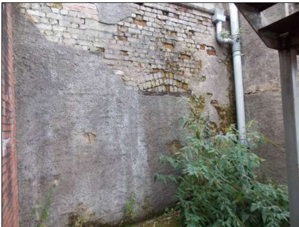
Figure 57: Detail of segmental arched-head of a former opening.
