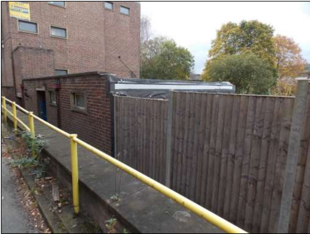
Figure 89: General view of Building L facing onto the central lane.
