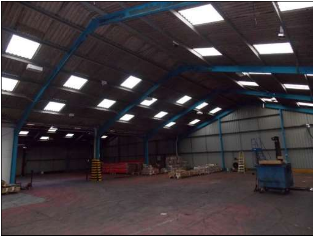
Figure 47: Internal view of Building A.
