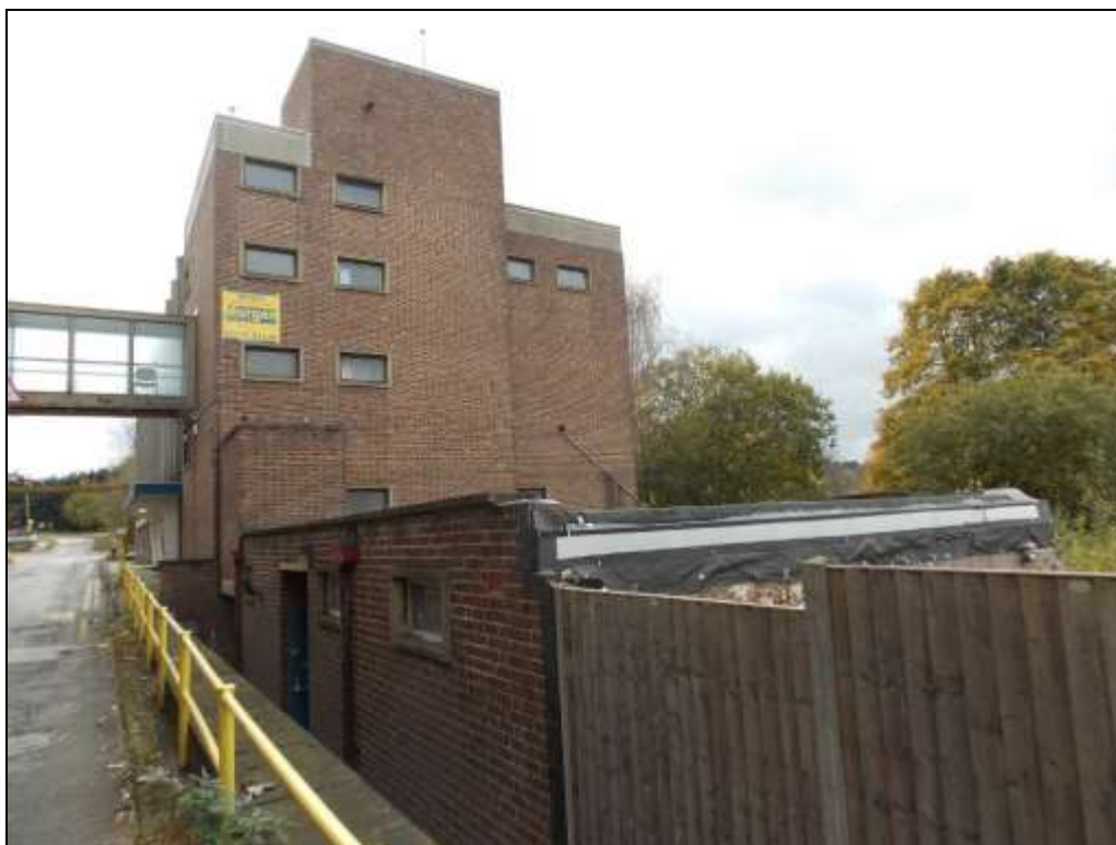
Figure 92: General view of Building M facing onto the central lane.
