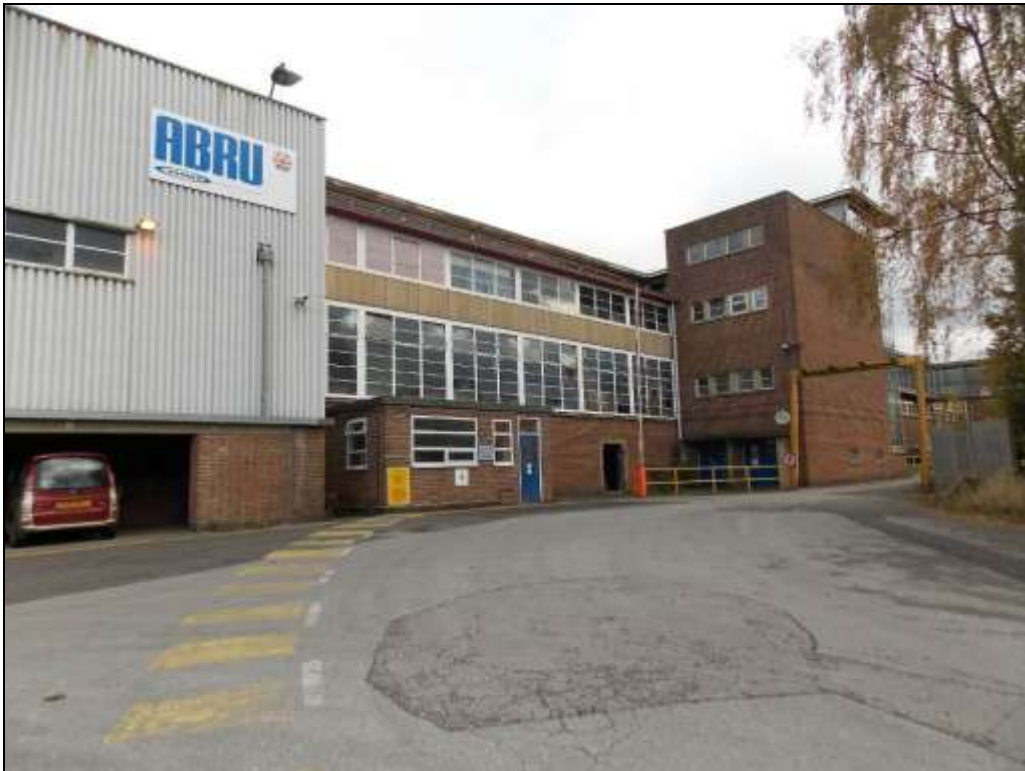
Figure 81: Northern end of Building K with gate house.
