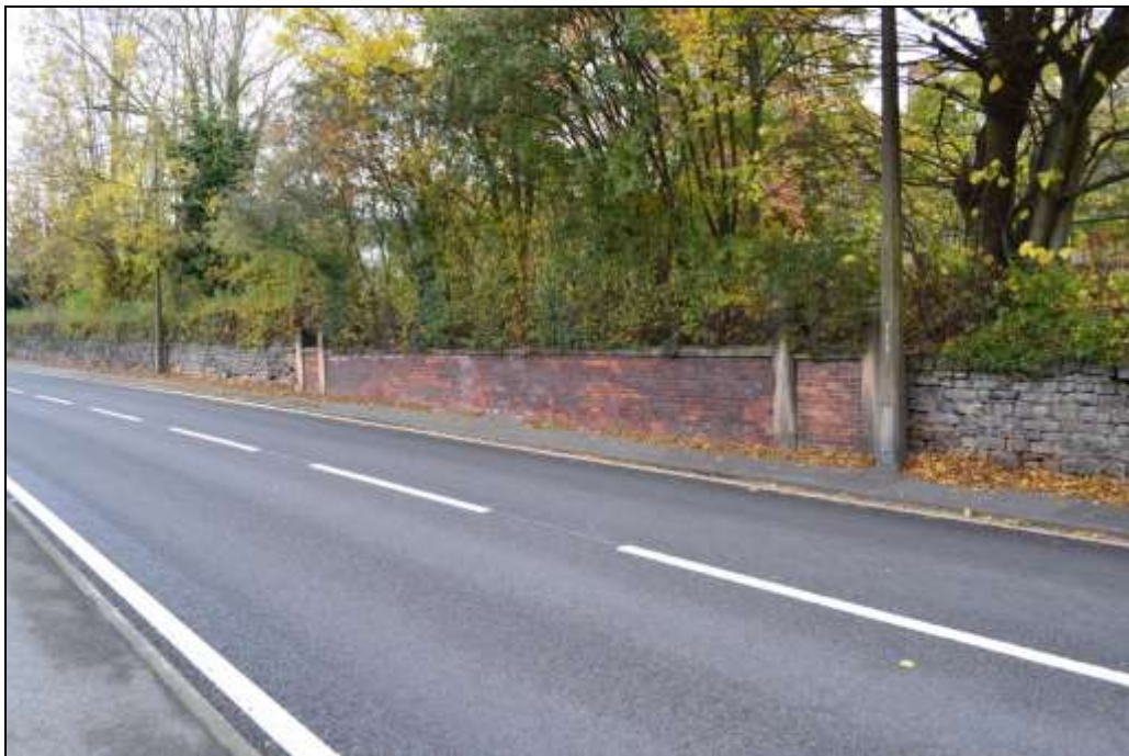
Figure 18: The stone and brick wall which forms the southwestern boundary of the PDA. The former entrances to the two late 19 th century villas are indicated by the two sets of sandstone pillars.
