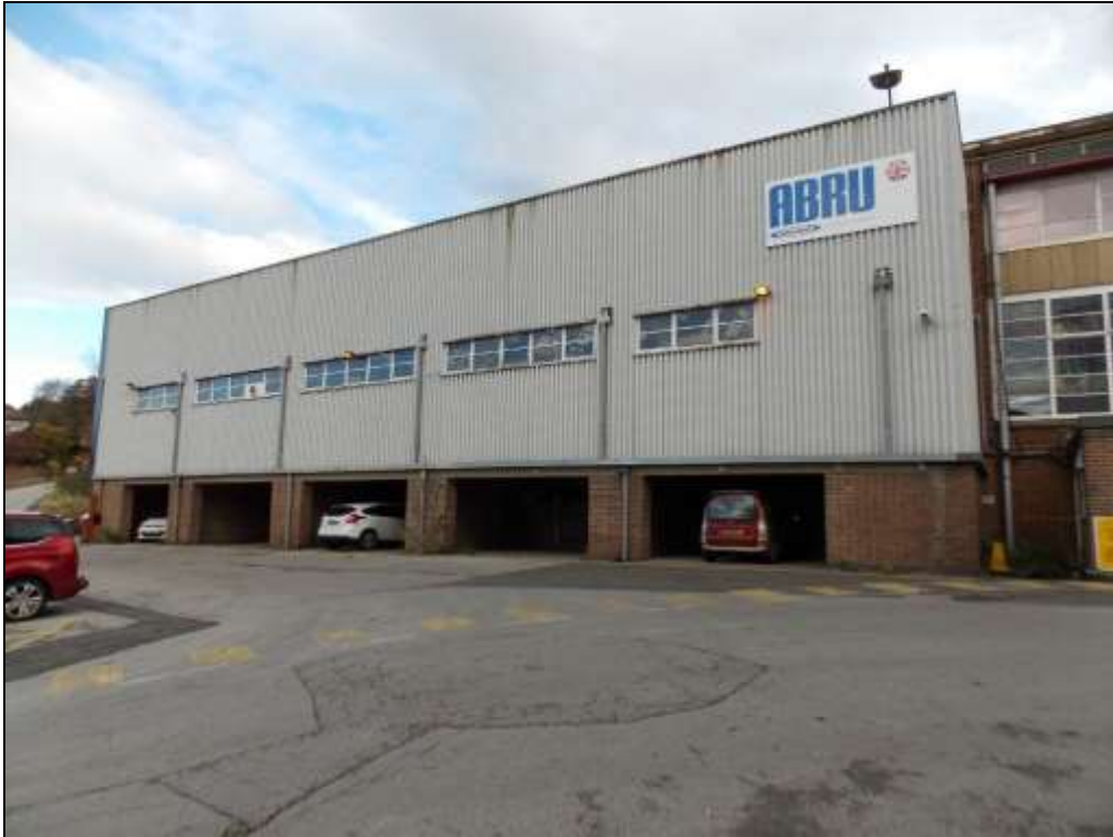
Figure 76: General view of Building J, looking north-east.
