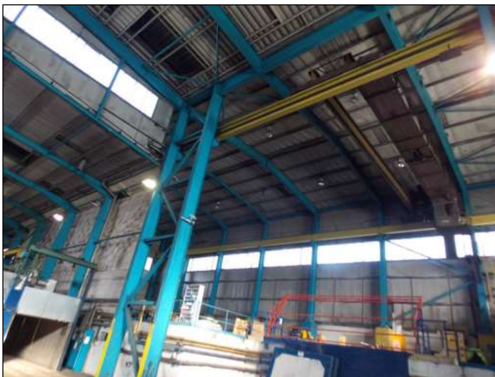
Figure 52: Building C with gantry.
