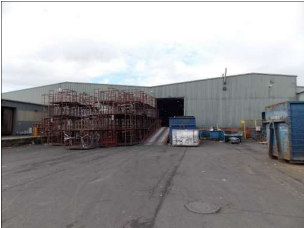
Figure 53: General view of Building D, looking north-west.
