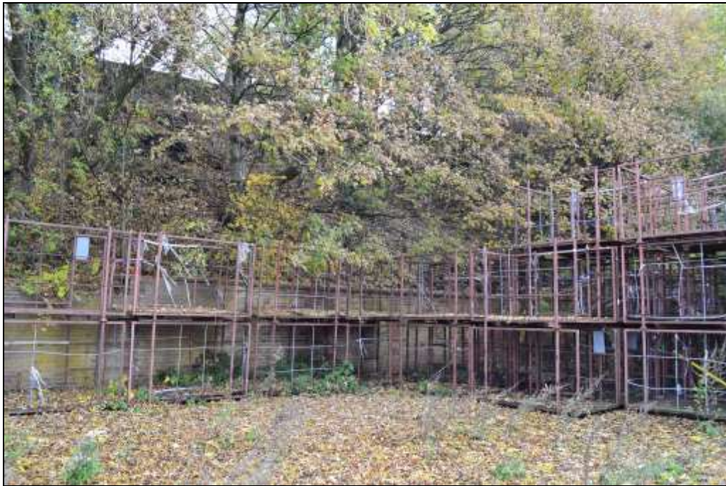
Figure 37: View east of the numerous metal storage containers against the brick retaining wall. The slope of the landscape beyond is quite steep.
