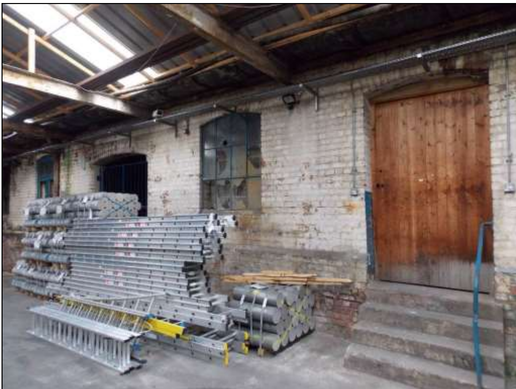
Figure 74: Detail of windows and doorways along the eastern wall.
