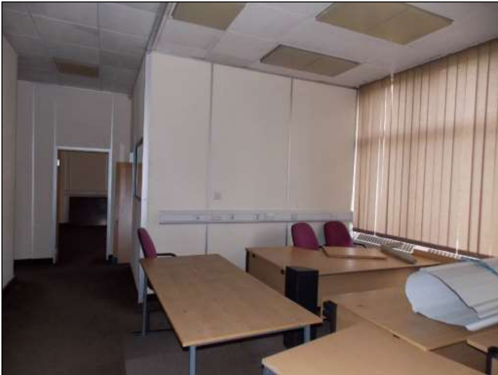
Figure 93: Office room within the ground floor of Building M.
