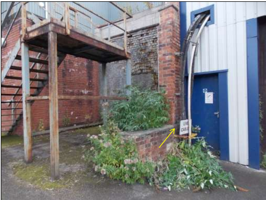
Figure 56: Remains of chamfer plinth (arrow) and blocked-up arched opening.
