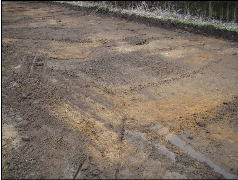
Figure 10: Part of Section C of the pipeline showing the construction sand amongst the topsoil.
