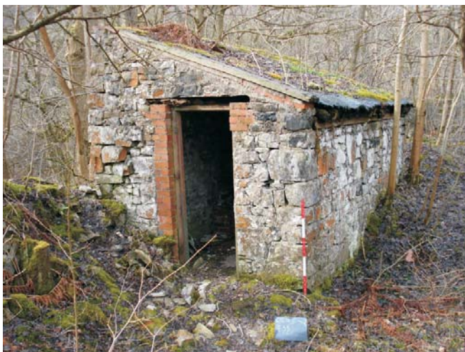
Figure 39: Feature 38- Station House at Blackwell Halt. Scale = 1m.
