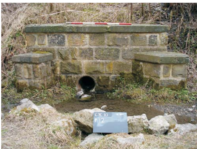
Figure 13: Feature 12- Culvert. Scale = 1m.
