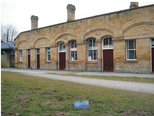
Figure 14: Feature 13- Bakewell Station. Scale = 1m.
