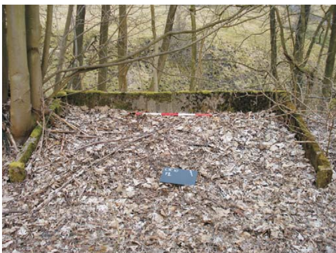
Figure 3: Feature 2- Concrete structure, line side hut. Scale = 1m,
