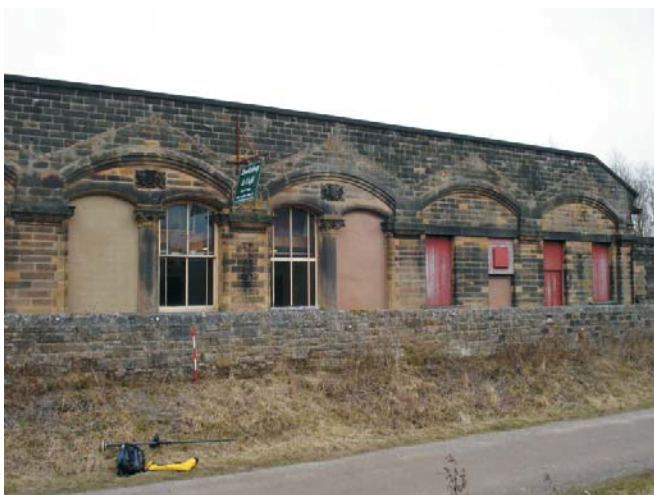
Figure 11: Feature 10-Hassop Railway Station. Scale = 1m.
