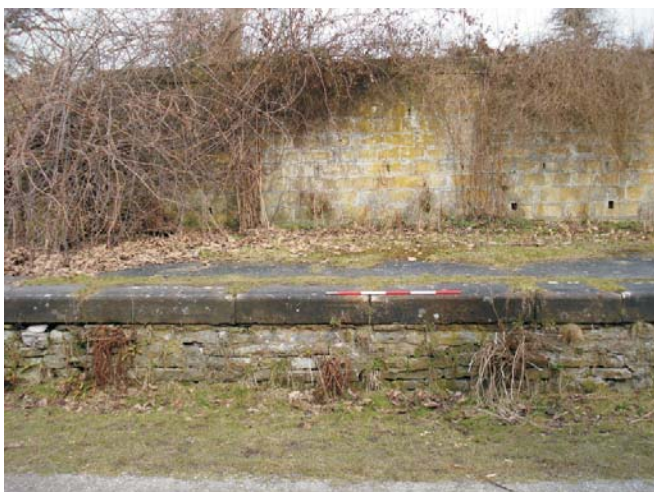
Figure 5: Feature 4- Platform at Great Longstone Railway Station. Scale = 1m.
