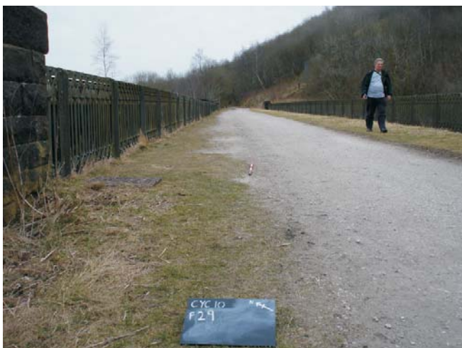
Figure 30: Feature 29- Miller's Dale Viaduct (South). Scale = 1m.
