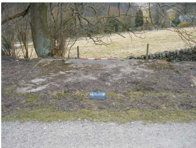
Figure 9: Feature 8- Concrete structure, line side hut. Scale = 1m.
