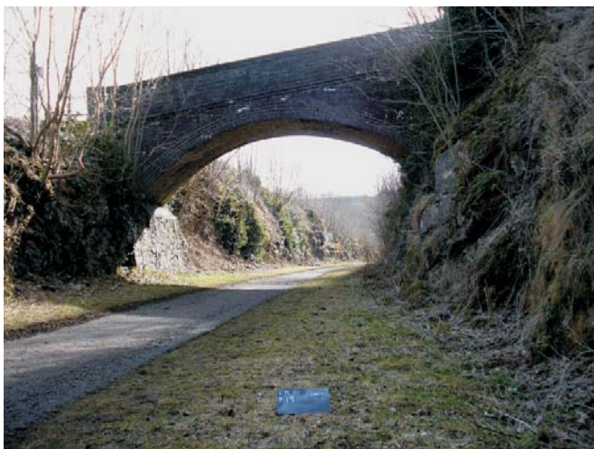
Figure 20: Feature 19-Bridge East of Monsal Railway Station. Scale = 1m.
