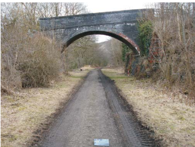
Figure 27: Feature 26- Bridge Near Litton Tunnel. Scale = 1m.
