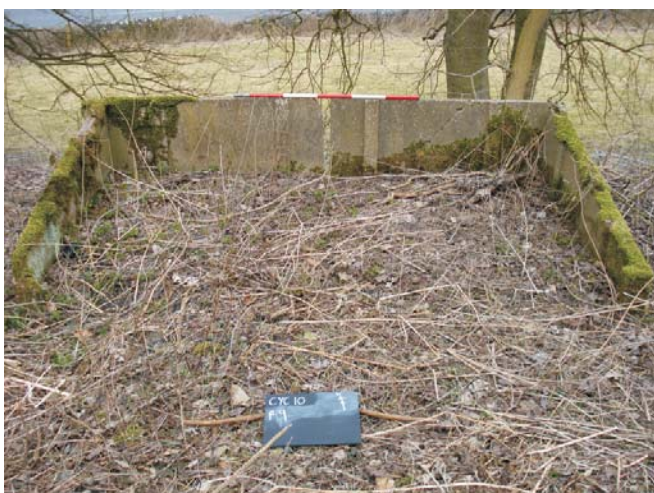
Figure 10: Feature 9- Concrete structure, line side hut. Scale = 1m,
