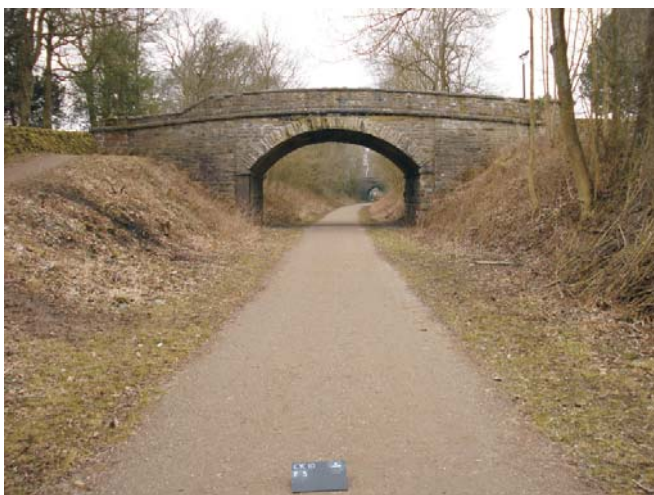
Figure 4: Feature 3- Road Bridge near Great Longstone Railway Station. Scale = 1m.
