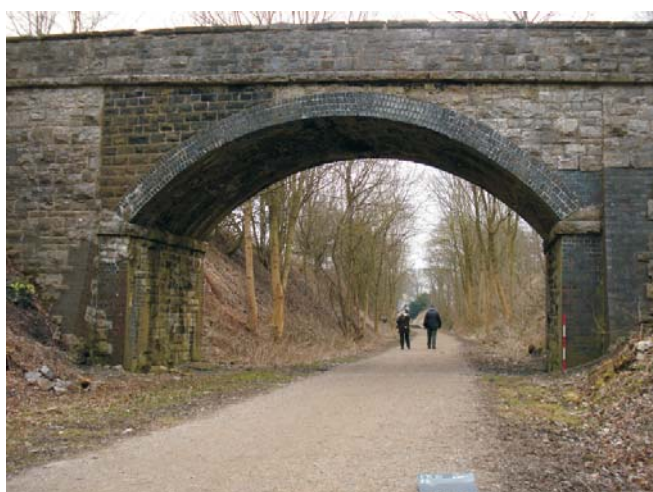
Figure 7: Feature 6- Road Bridge near Great Longstone Railway Station. Scale = 1m.
