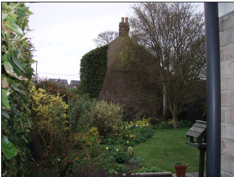
Figure 11. Farmhouse, north facing elevation
