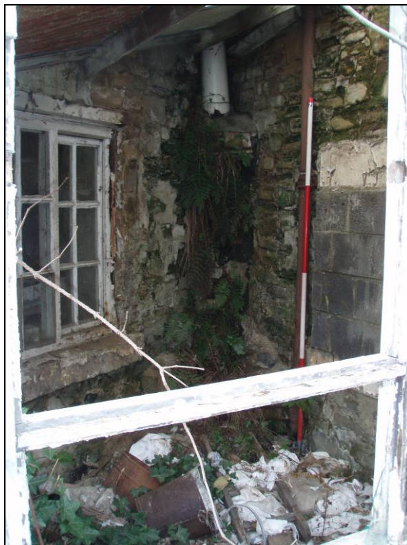
Figure 13. Farmhouse, lean-to interior
