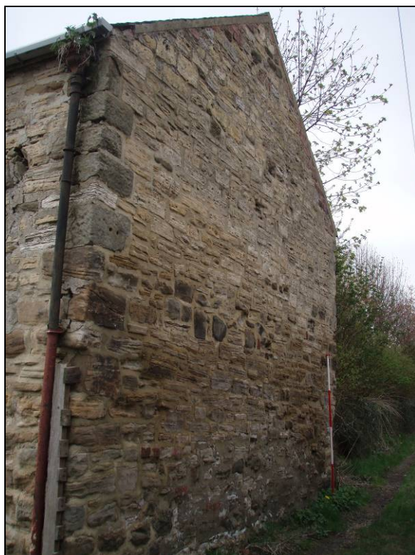
Figure 21. West barn, north facing elevation
