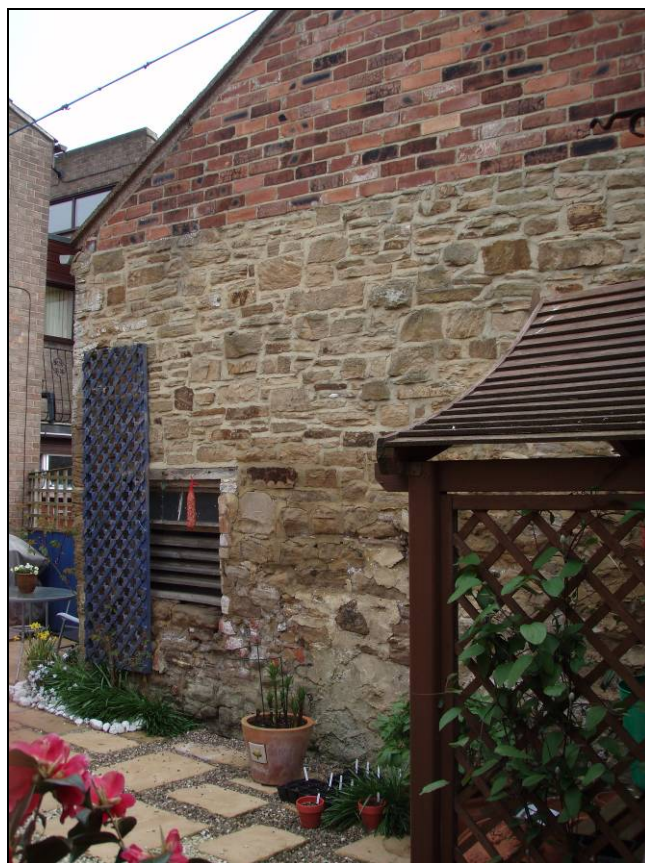
Figure 19. East barn, west facing elevation
