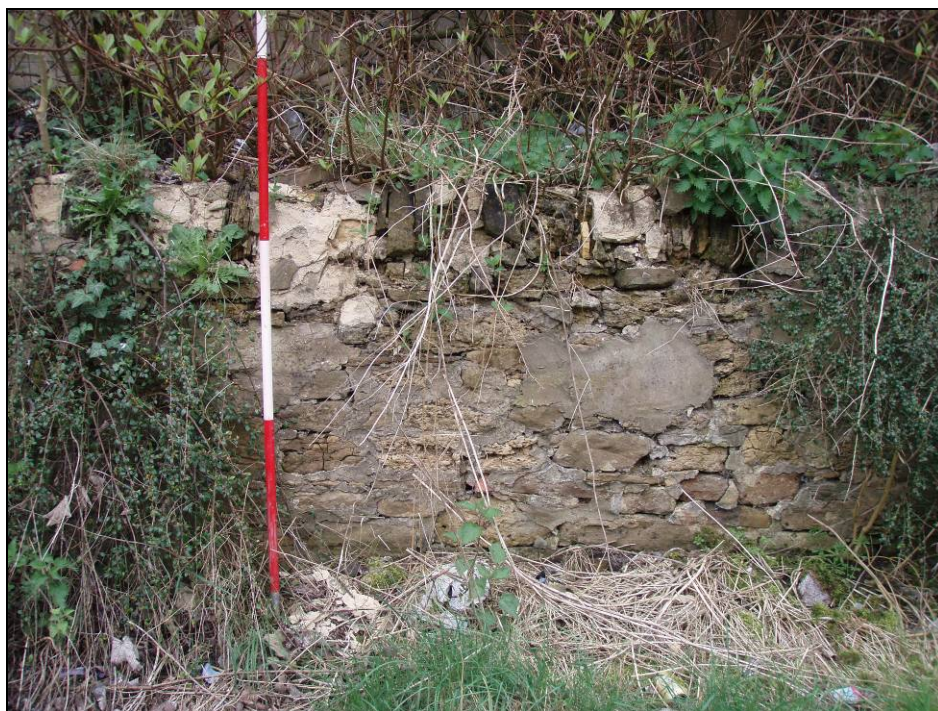
Figure 23. East – west wall
