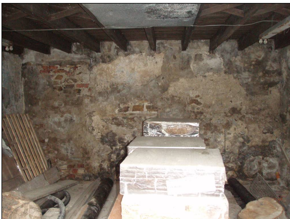
Figure 18. East barn, interior
