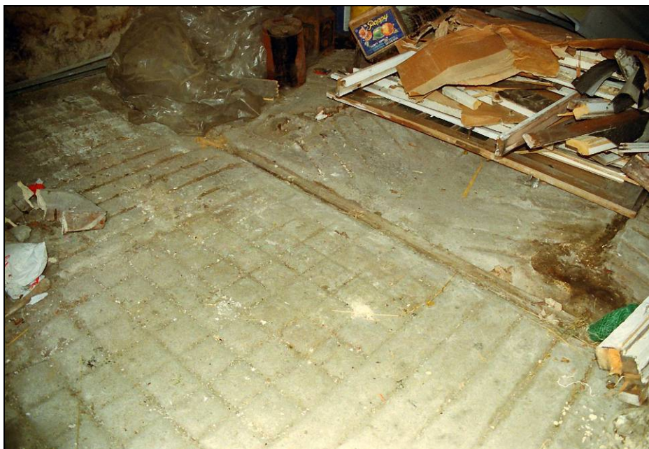
Figure 22. West barn, interior floor
