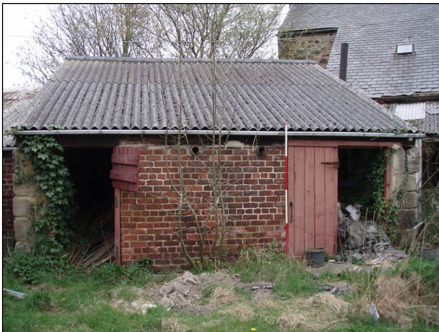
Figure 15. Sheds attached to farmhouse
