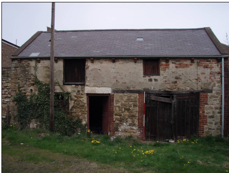
Figure 17. East barn, South facing elevation
