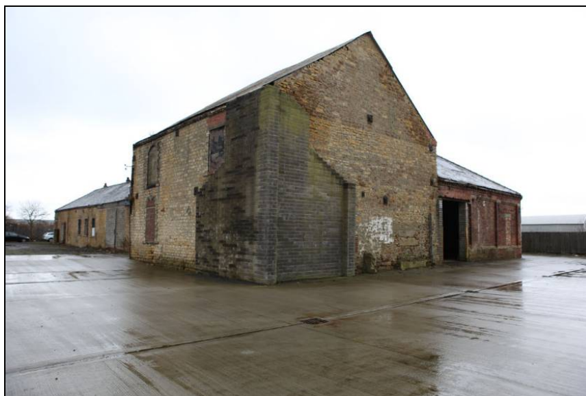
Fig. 11 Former NCB Workshops
