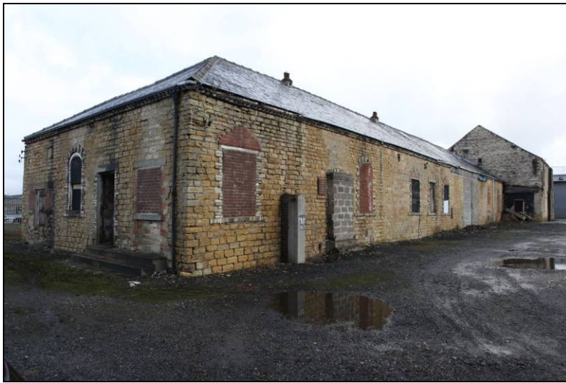
Fig. 9 Former NCB Workshops
