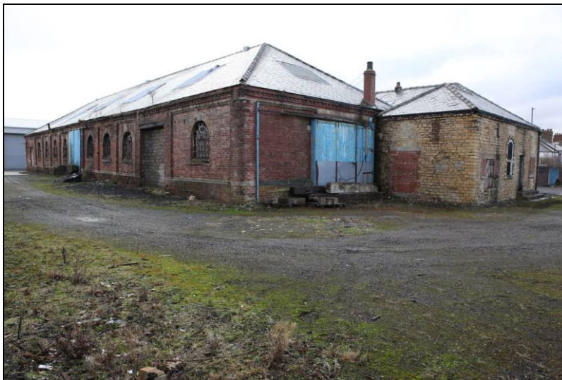
Fig. 10 Former NCB Workshops
