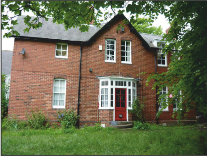
Fig. 9 East facing elevation
