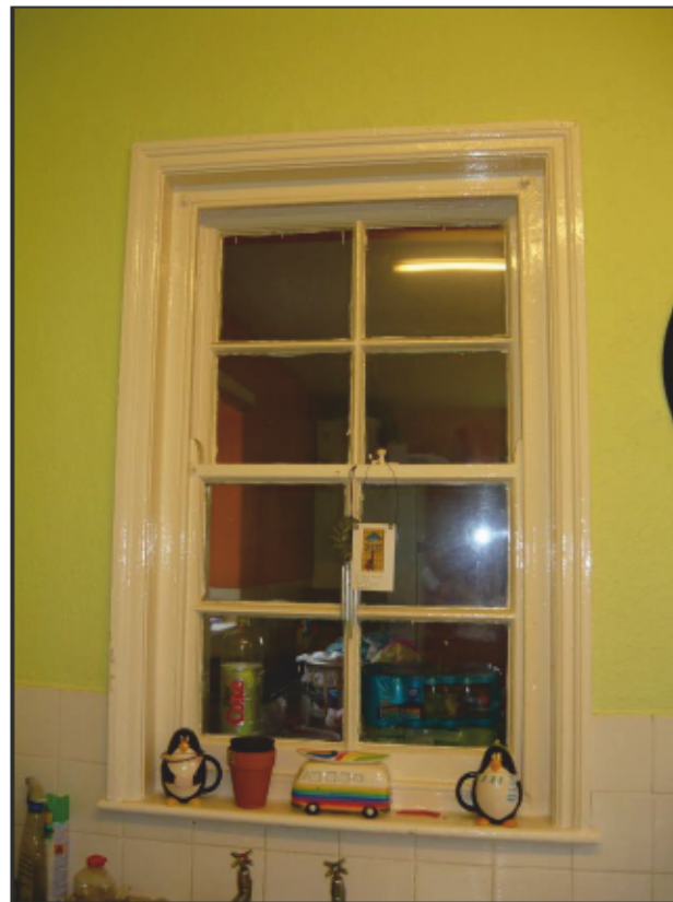
Fig. 18 Internal sash window to utility room
