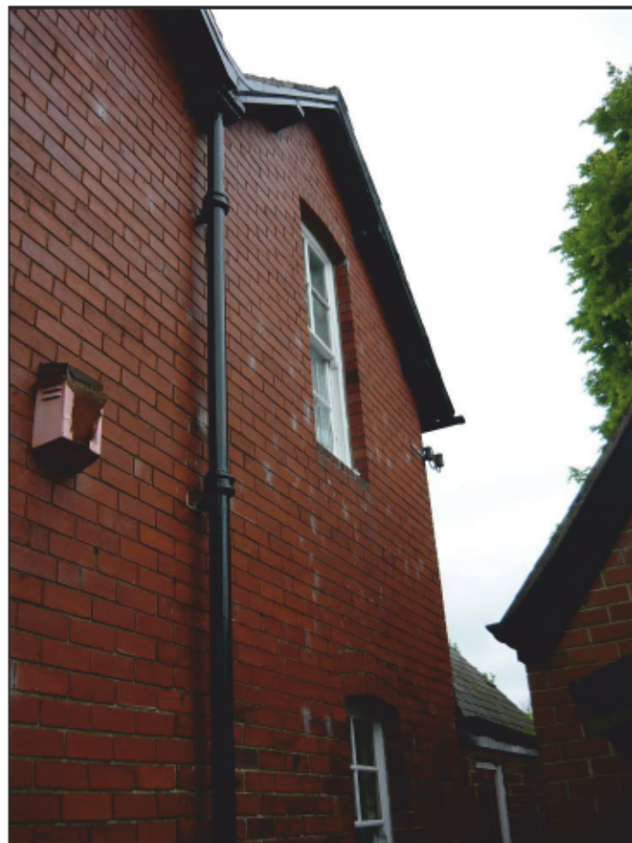
Fig. 12 North facing elevation first floor window
