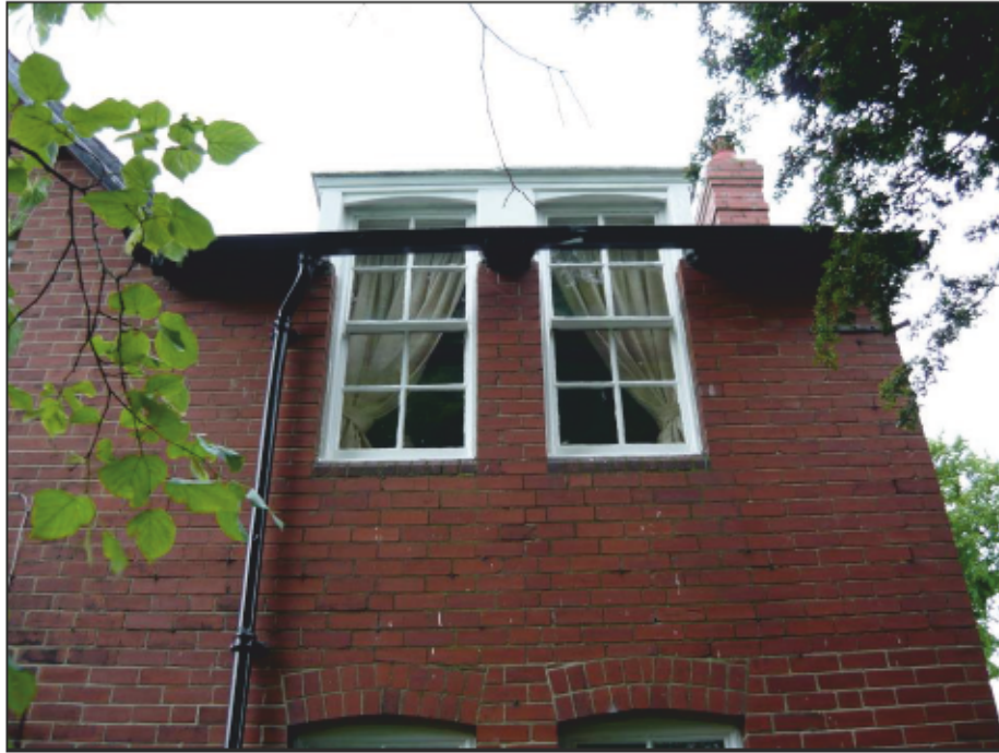
Fig. 11 East facing elevation first floor windows
