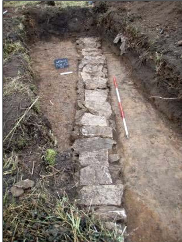
Fig. 11 View of Culvert (503) in Trench 5. Looking west. (Scale: 2m)
