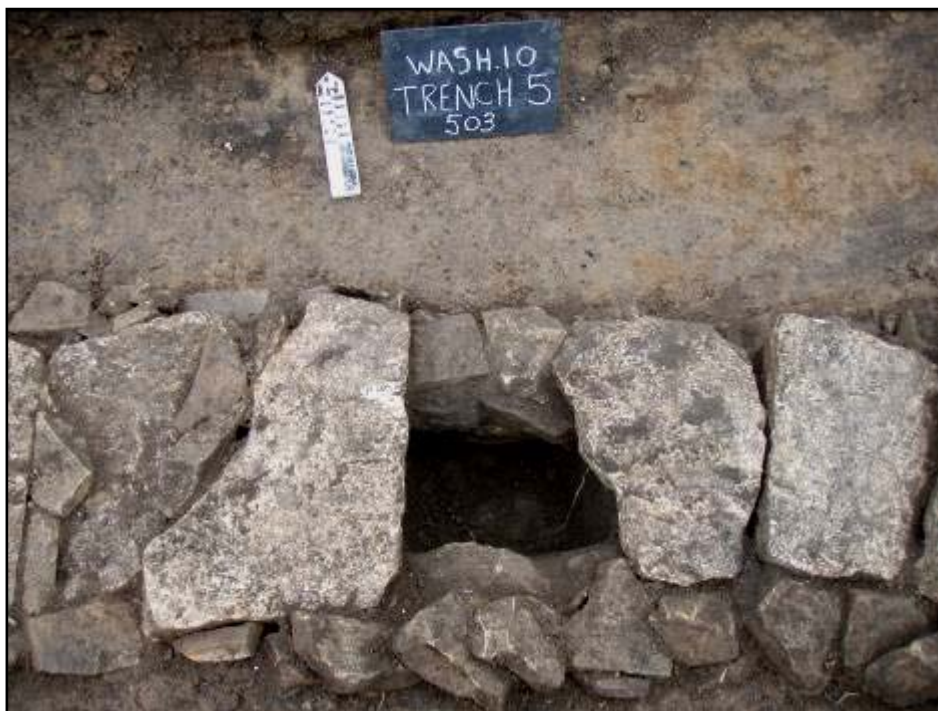
Fig. 12 View of Culvert (503) in Trench 5. Looking north. (Scale: 0.25m)
