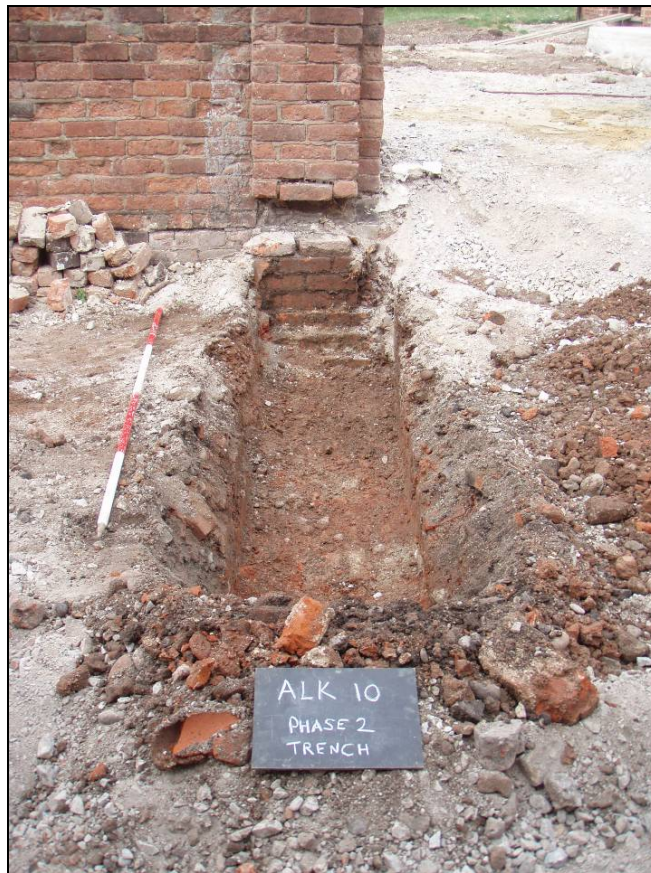
Fig. 12: Foundation trench for realignment of external wall. Facing west. Scale 2m
