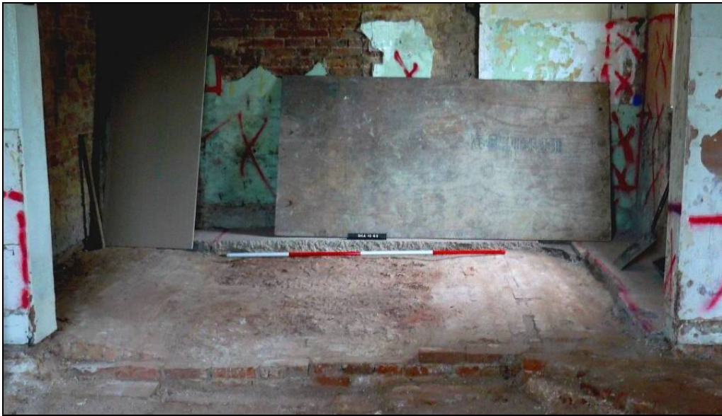
Fig. 7: Room G3, top sections of vaulted cellar roof (304) exposed below (301). Facing north. Scale 2m
