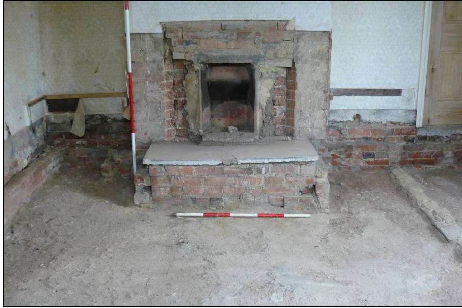
Fig. 10: Room G7A, Floor level (702) and fireplace. Facing east. Scale 1m & 2m
