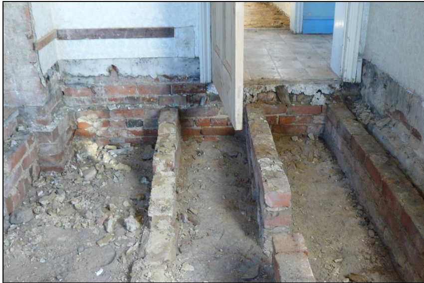
Fig. 9: Sleeper walls (701) which supported wooden floor in Room G7. Facing east
