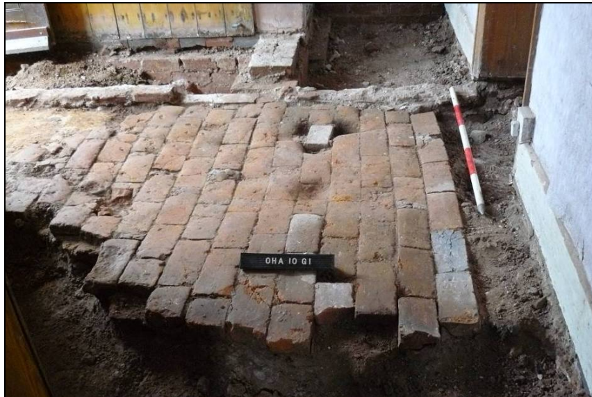
Fig. 4: Brick floor (103) in room G1 with (106) in the foreground. Facing east. Scale 1m.
