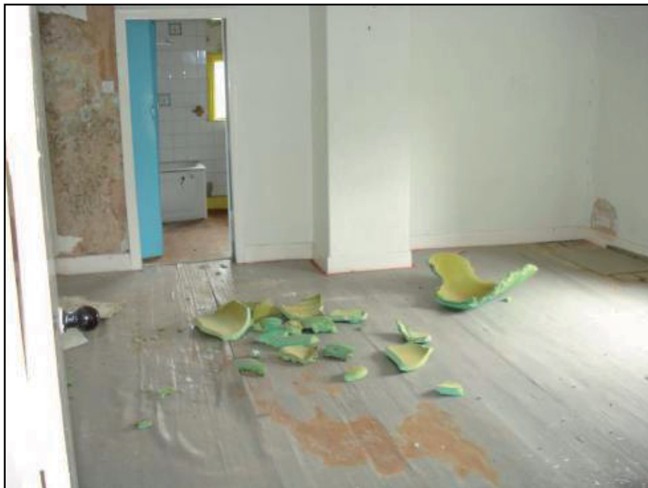
Fig- 27 Room 11 with Room 12 beyond
