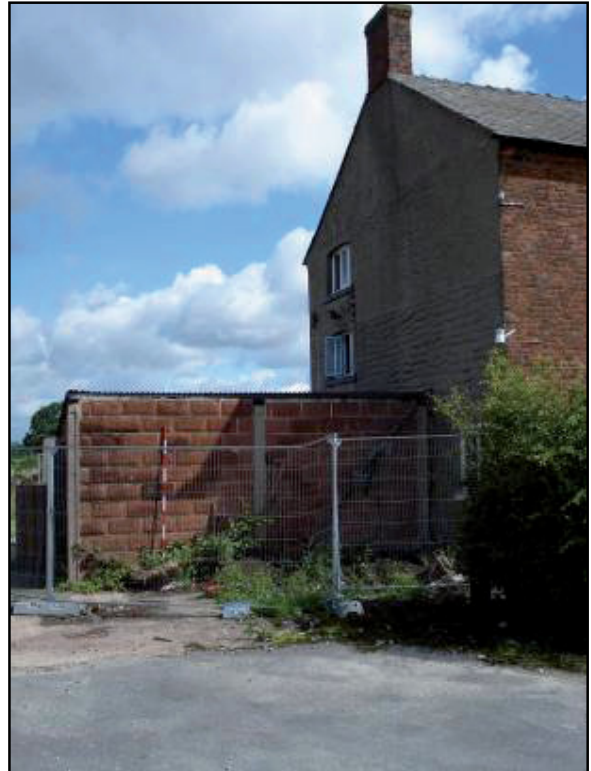
Fig 11- Detail of Garage on South Elevation
