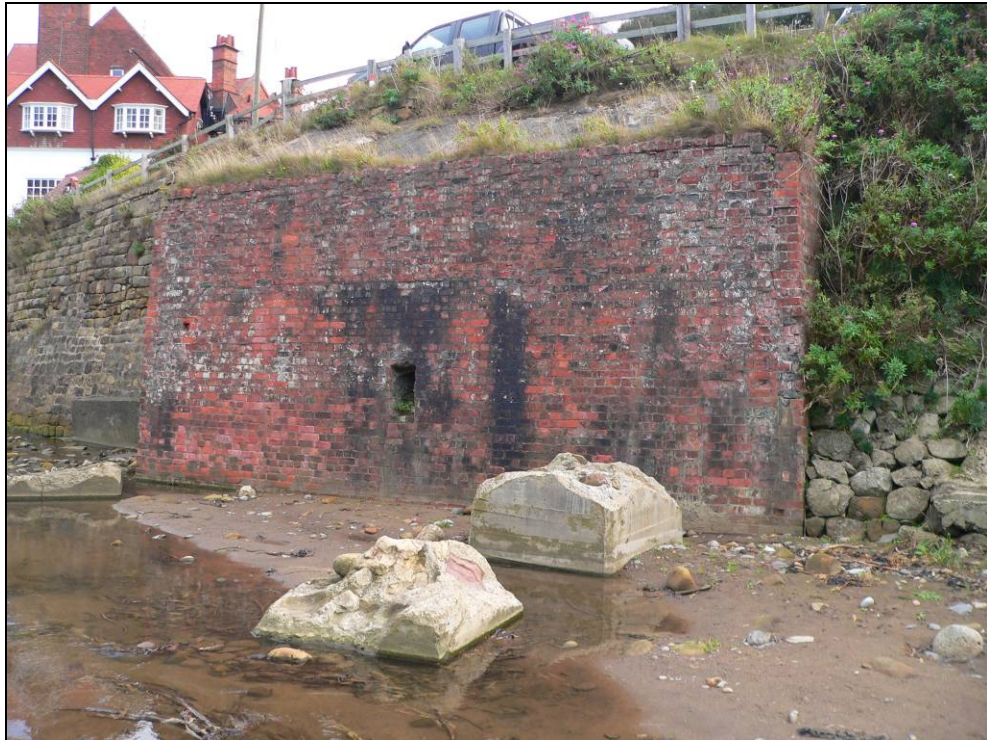
Figure 5.2.10 Anti-tank blocks in Sandsend beck beneath the remains of a former brick-built railway viaduct.
