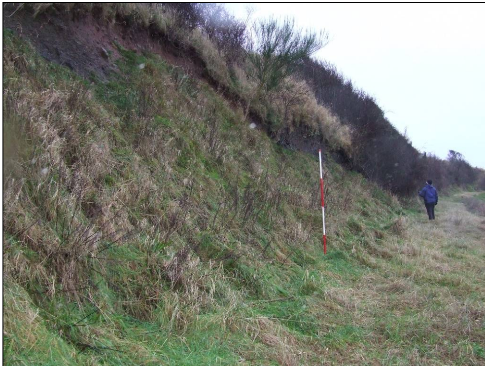
Fig 5.13.6 The cliff face below the enclosure. The ranging pole is roughly parallel to the centre of the enclosure.
