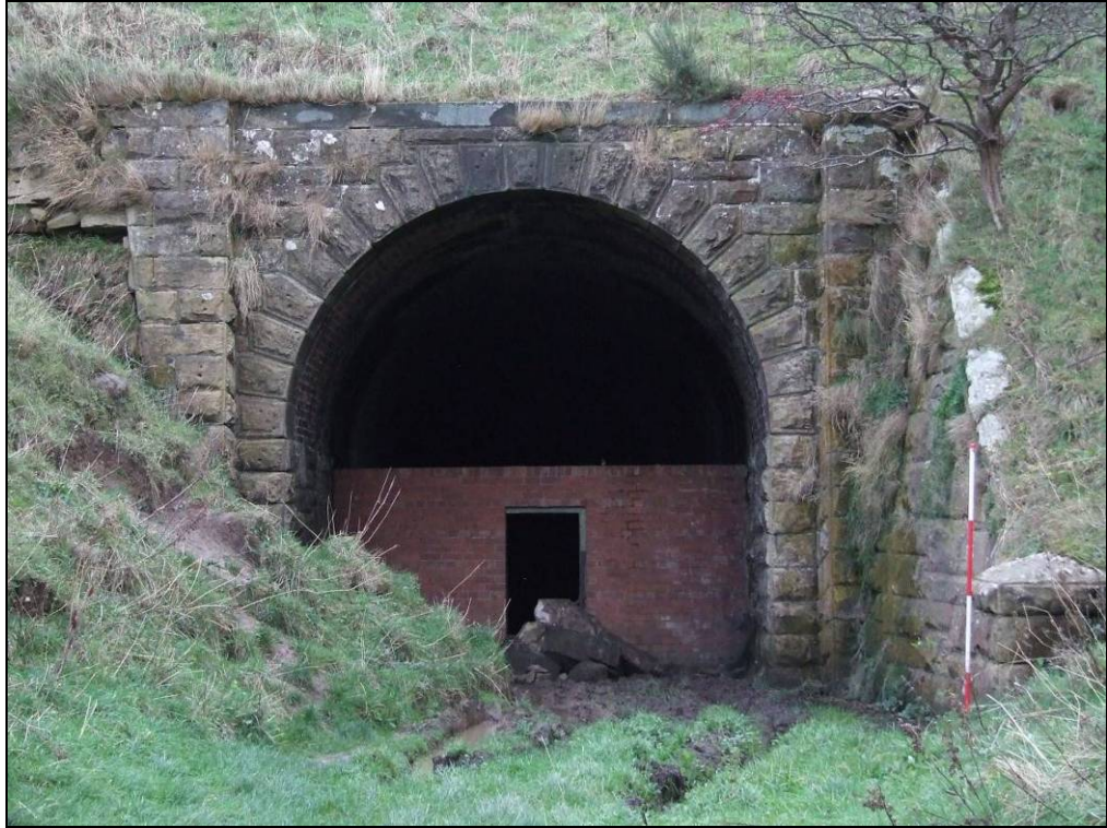
Figure 5.2.7 Tunnel mouth (422) at Kettleness end looking south.
