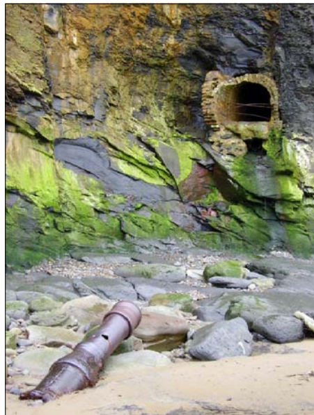
NERCZA2_0065: GPS 24-25. Outfall Sewer
