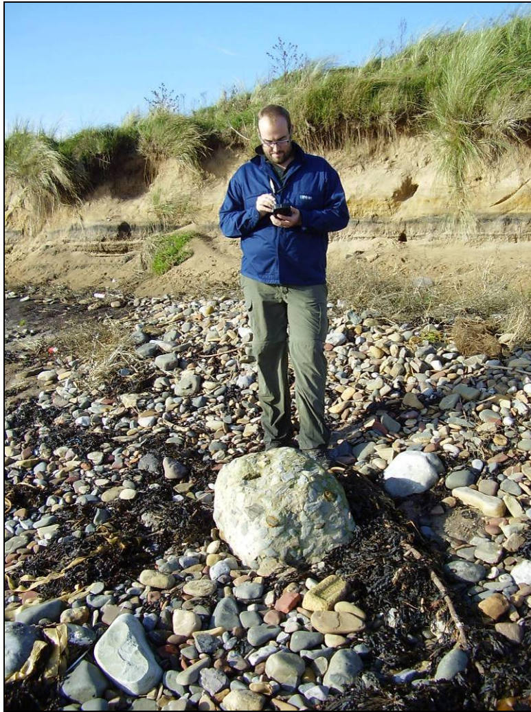
Fig 5.9.11 A heavily eroded anti-tank block in the make up of a storm beach at Low Hauxley.
