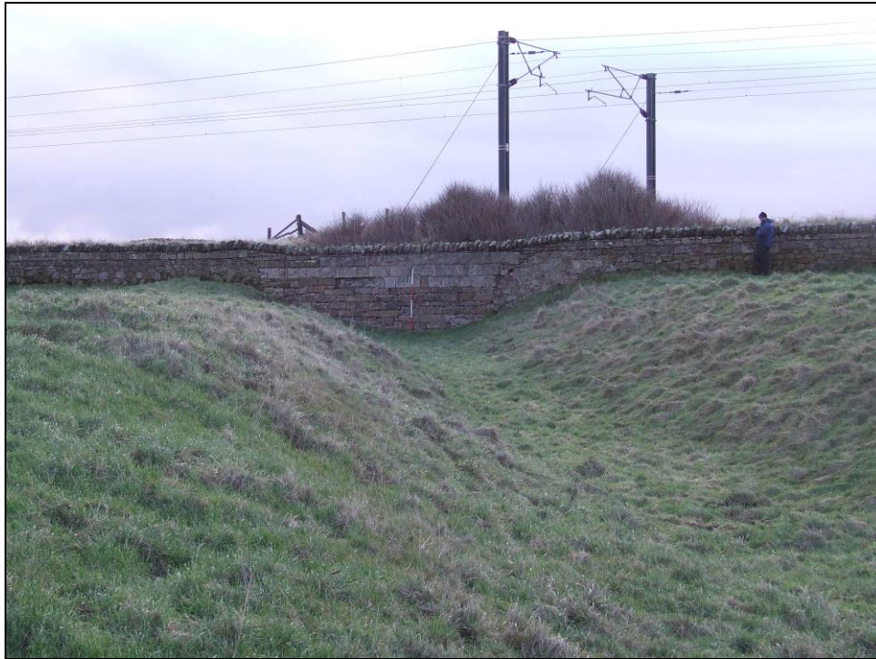
Fig 5.12.5 The former railway cutting, showing the modern route of the line behind the stone wall.
