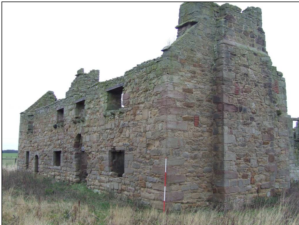
Fig 5.8.7 The later Dower house at Low Chibburn
