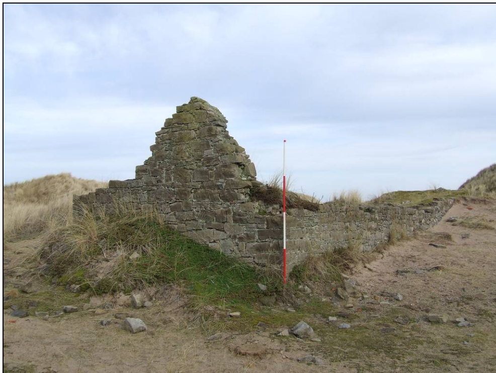
Fig 5.14.17 Partially upstanding gable end of Longhouse (409)
