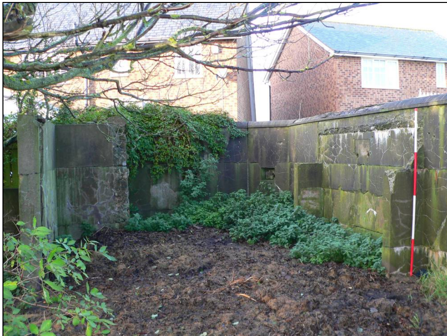
Fig 5.7.7 The defended latrine block (440) with blocked up loopholes now visible.
