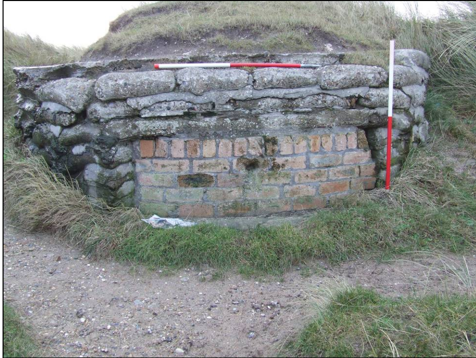
Fig 5.7.21 Circular pillbox (506) showing brick-blocked aperture.
