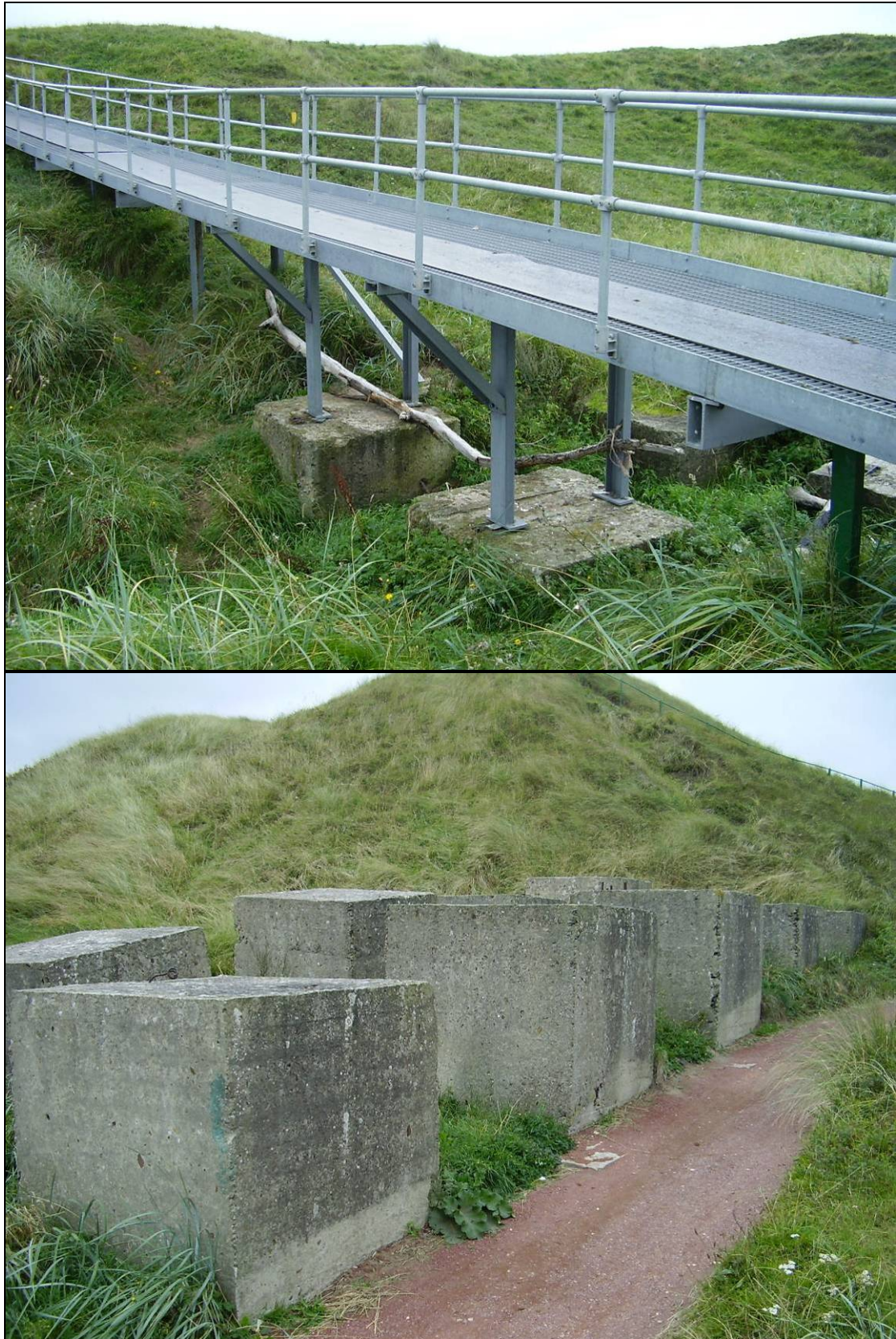
Fig 5.5.13 Top: Anti tanks block utilised as a foundation for a modern bridge. Bottom: Cache of anti tank cubes probably removed from their original location.
