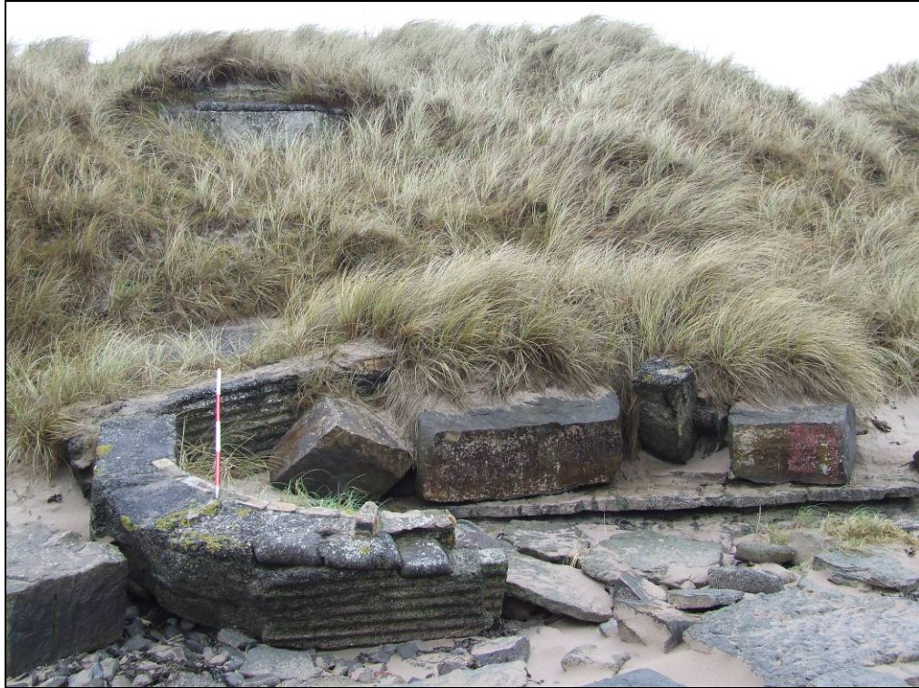
Fig 5.16.23. Probable pillbox eroded onto the beach near Seahouses; there are many such examples along this stretch of coast.
