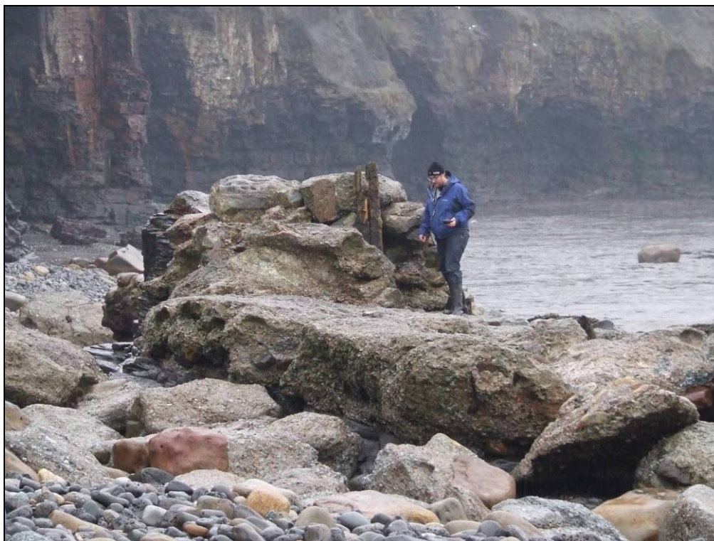
Figure 5.2.14 A rapidly eroding Alum pier at Sandsend that is exposed to direct wave action.
