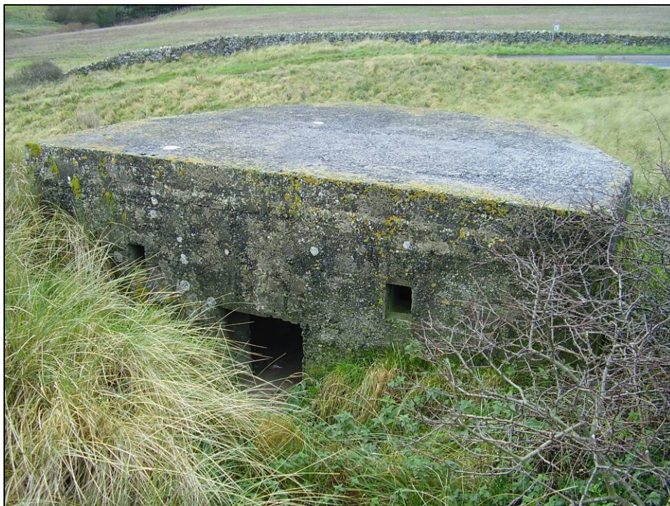
Fig 5.15.8 The rear entrance of the same pillbox.
