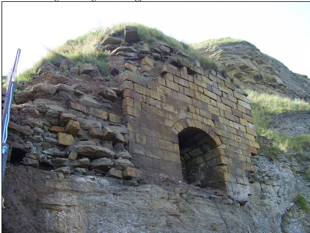
Figure 5.3.3. Remains of alum house exposed in the cliff face at Hummersea.
