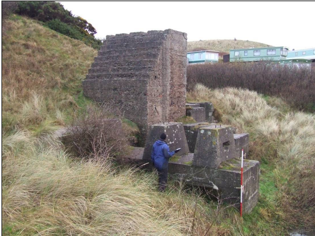
Fig5.16.25 Concrete base for winding gear for the quarry 2km to the south.
