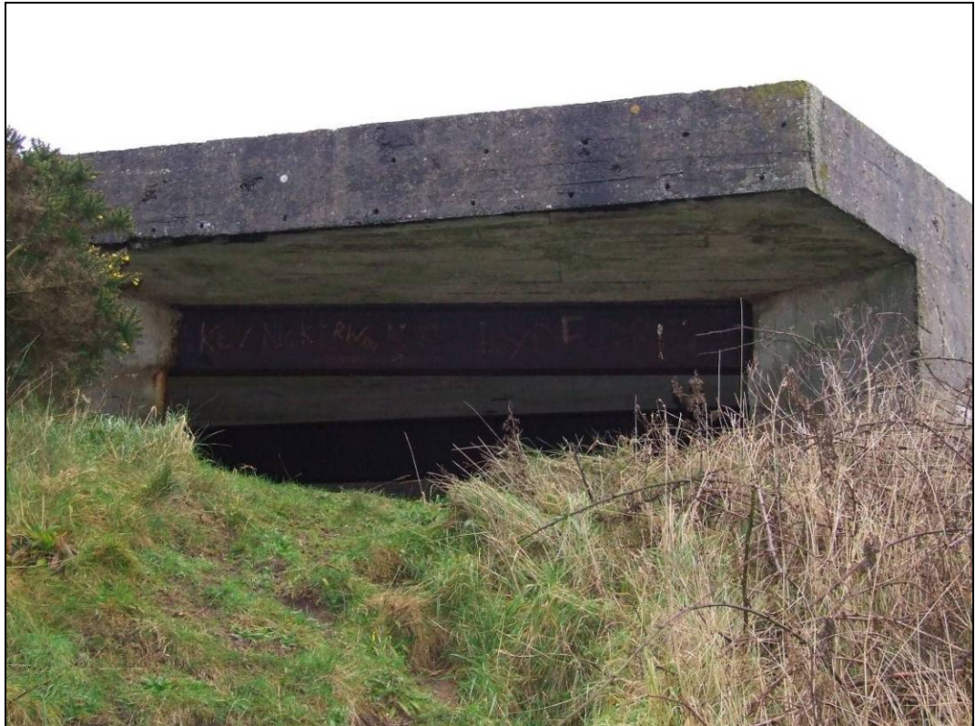
Fig 5.16.13 Budle battery (500), clearly demonstrating scale of construction.
