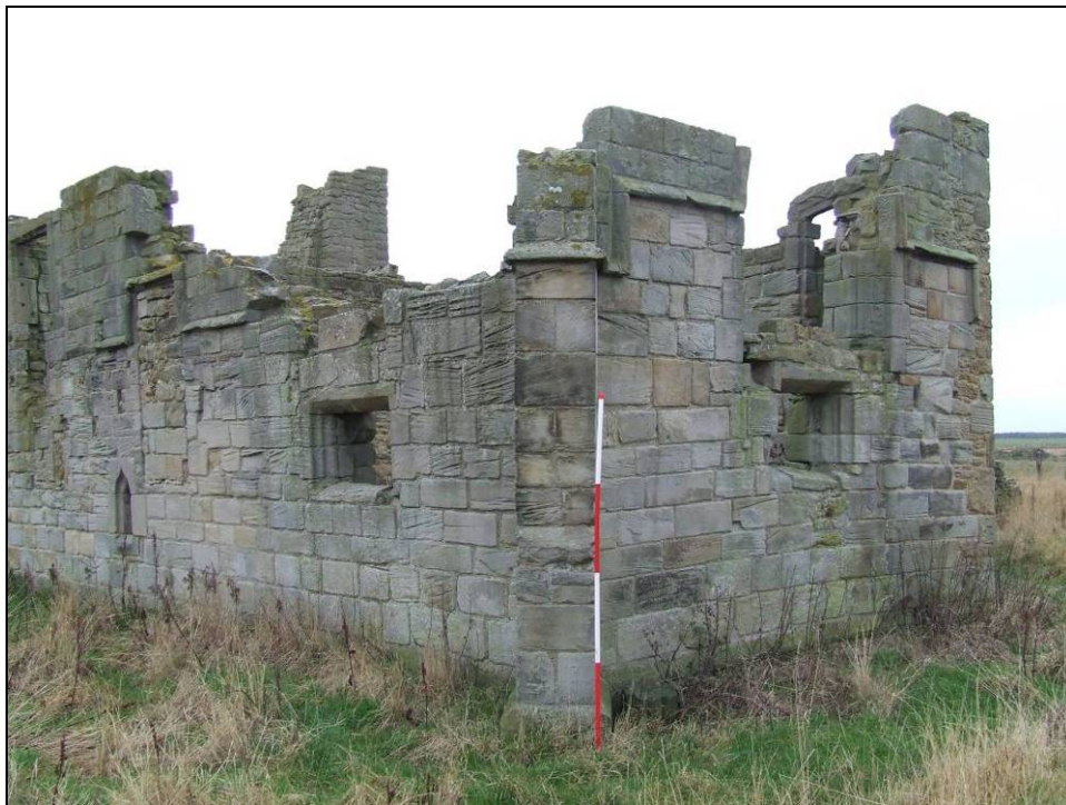
Fig 5.8.5 Part of the original Preceptory at Low Chibburn, with Second World War alterations to windows.
