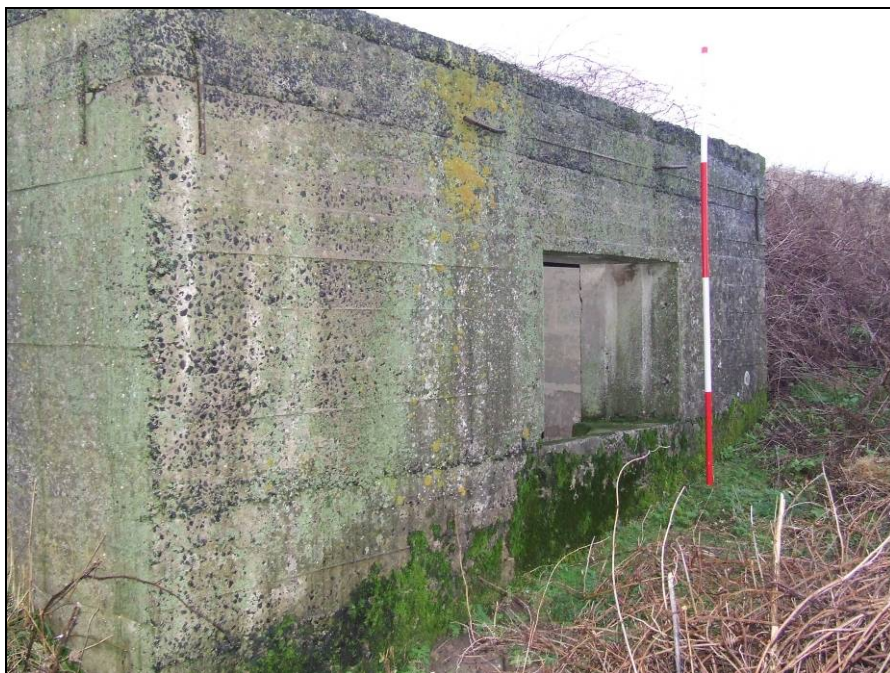
Fig 5.15.9 The front of the 6 inch gun emplacement (370)
