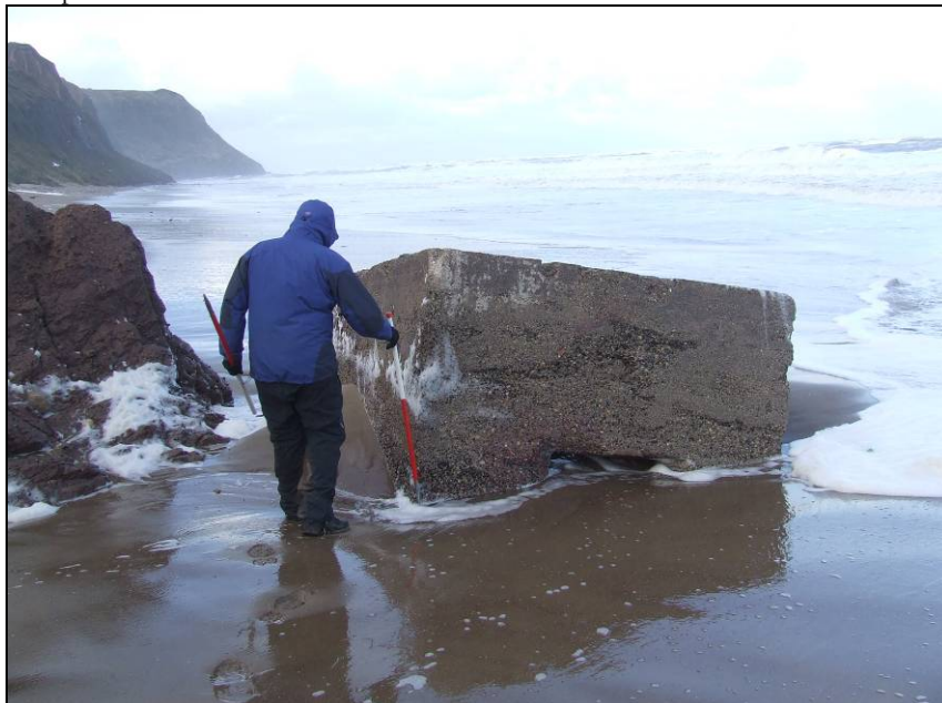
Figure 5.3.16 The same slumped pillbox as above more exposed to wave action, this time looking north. This photograph was taken in early December 2009 and demonstrates the changeable nature of the beach deposits and environmental conditions.
