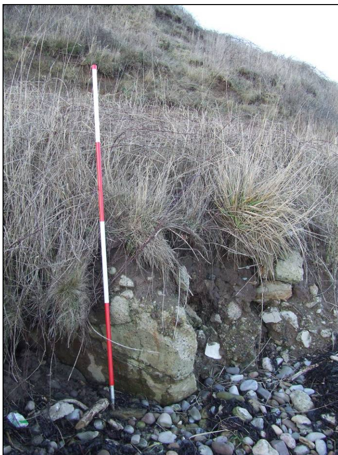
Fig 5.16.22. Concrete of Second World War date eroding out of the cliff base on the beach near Boulmer.
