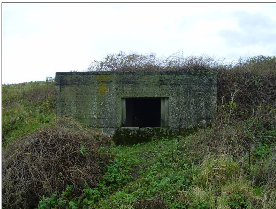
Fig 5.15.10 The same emplacement looking head on at the gun aperture.
