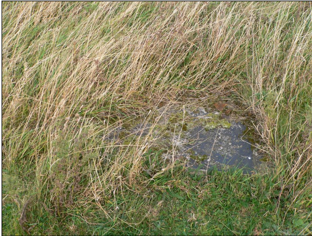
Fig 5.4.19 Remains of sealed hatch into ROC Cold War monitoring post.
