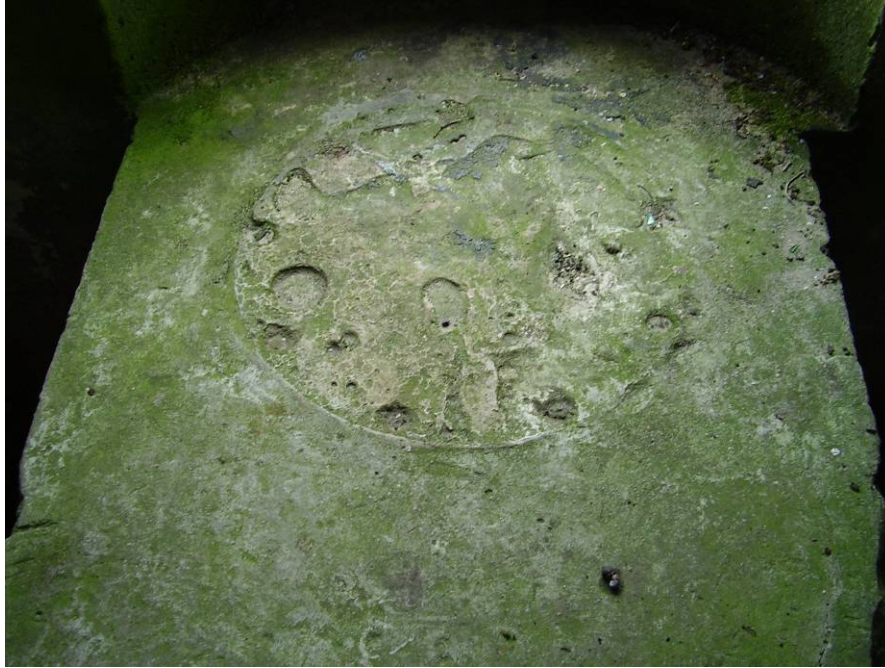
Fig 5.15.11 The concrete mounting for a 6 inch gun which would have been overlain by a metal mounting for the gun to swivel on.
