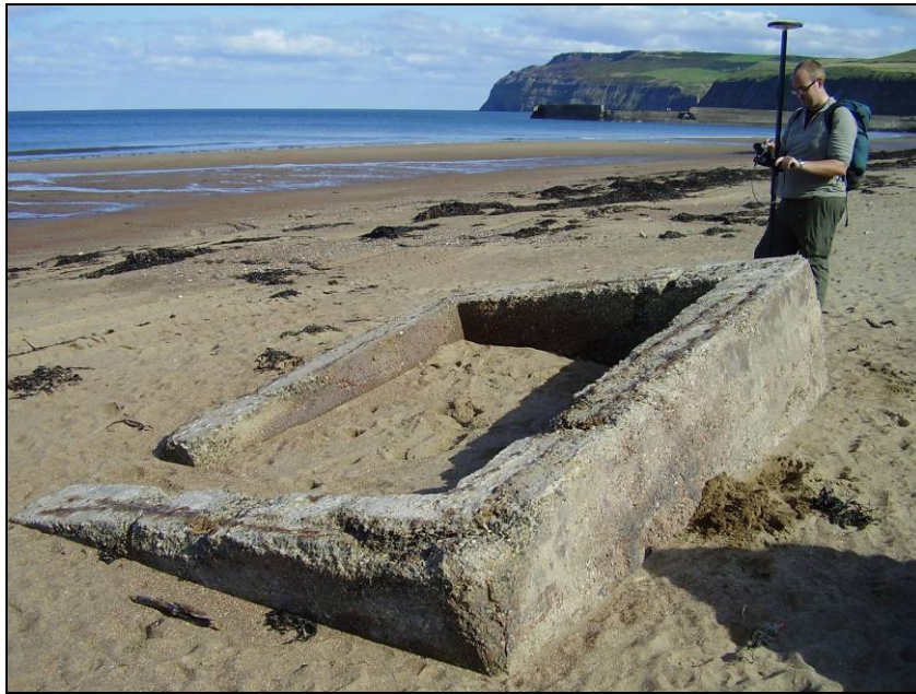
Figure 5.3.15 Slumped pillbox on the beach looking south towards Skinningrove harbour as seen in September 2009 .
