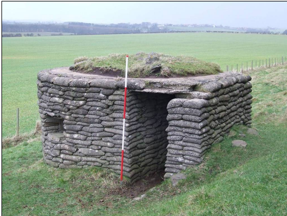
Fig.5.16.1 Pillbox constructed of concrete sandbags south of Dunstan Steads.
