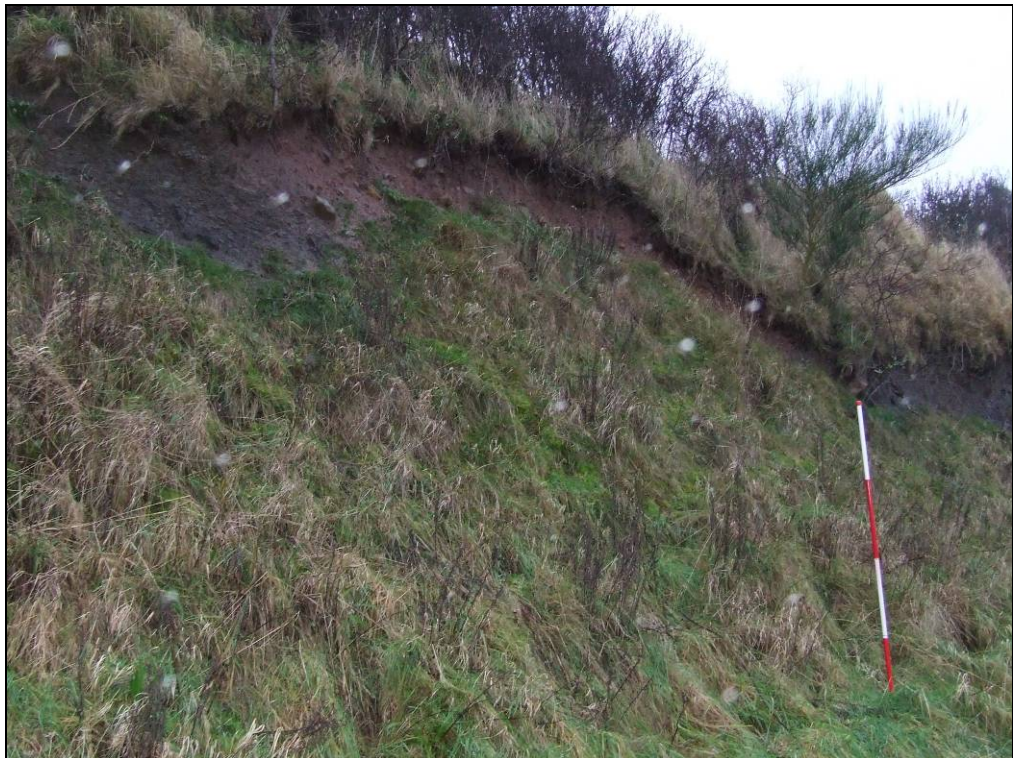
Fig 5.13.2 One of the cliff face slumps below the Fenham enclosure
