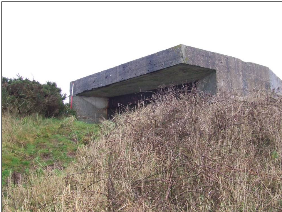
Fig. 7.8 The large gun emplacement at Budle Bay viewed from the south (1m scale visible).
