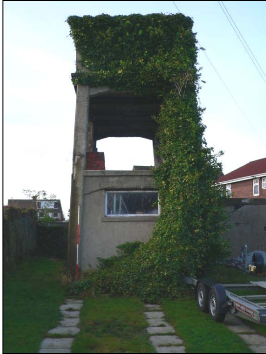
Fig 5.7.6 The WW1 water tower and store rooms underneath.
