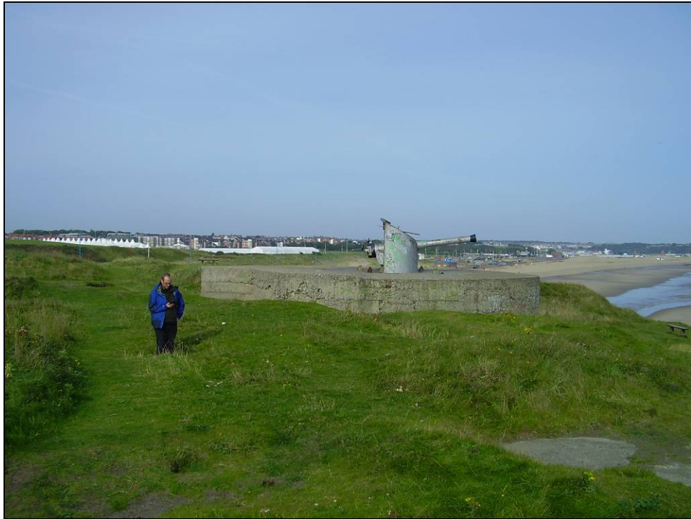
Fig 5.6.7 The position and depth of one of the weapons pits with one of the WW1 gun positions visible in the foreground.
