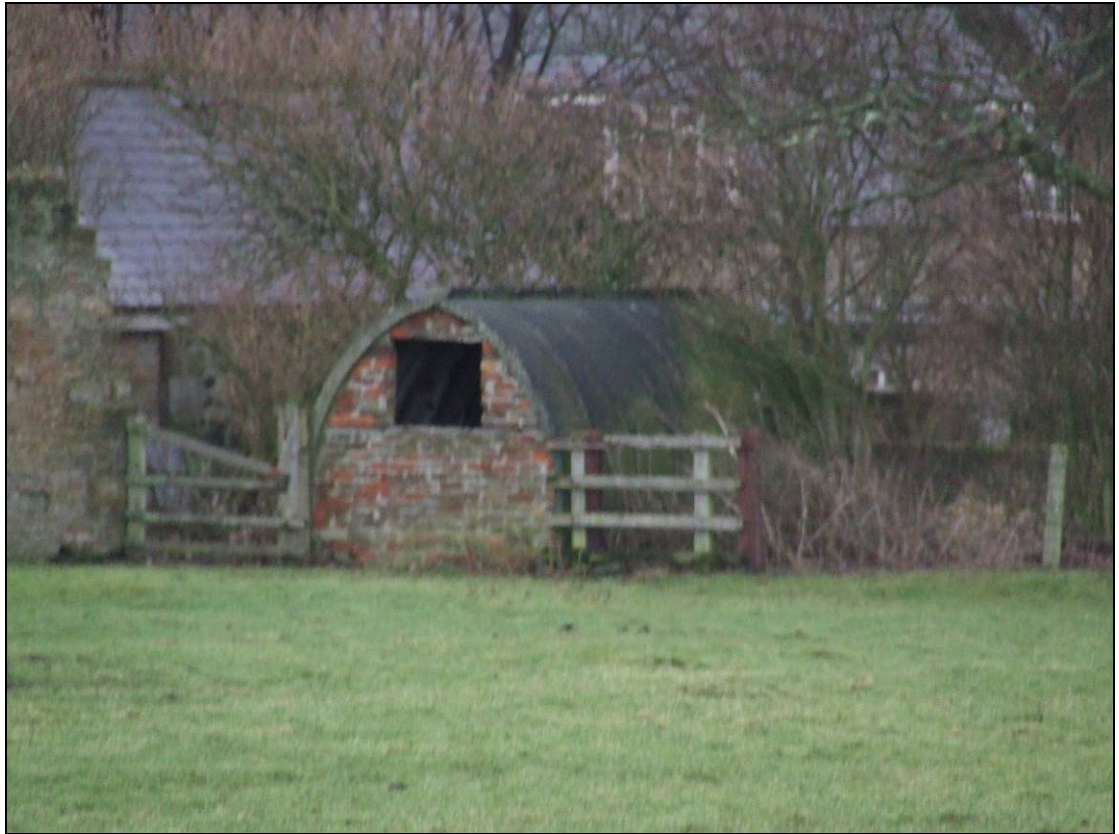
Fig 5.16.20. Stanton air raid shelter in garden of the Old Rectory, Howick.
