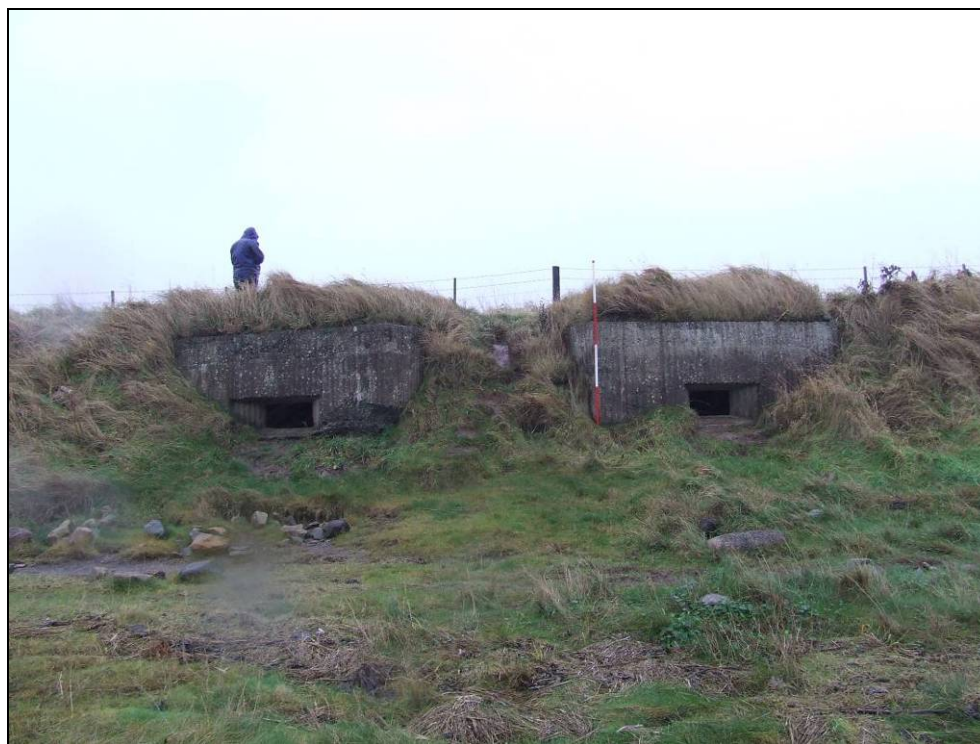
Fig 3.4 Unusual double pillbox on the shore at Goswick, survey by the Northumberland coast AONB survey, linked by underground access, see section 5.16
