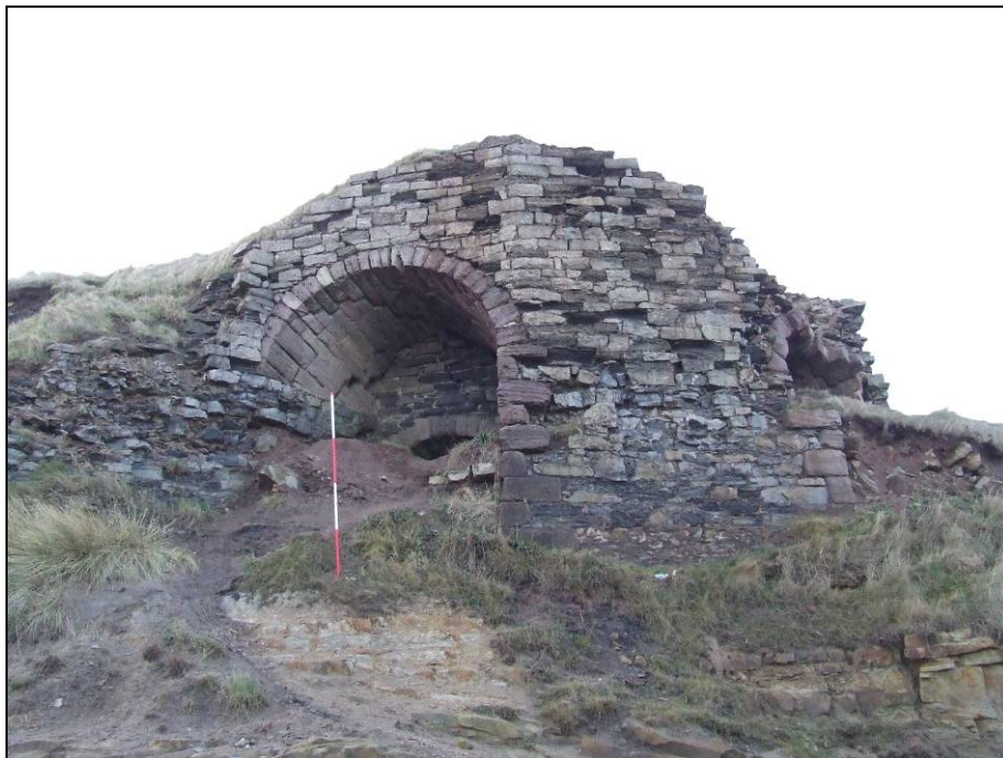
Fig 5.12.6 Kiln 458 on the cliff edge, is being eroded.
