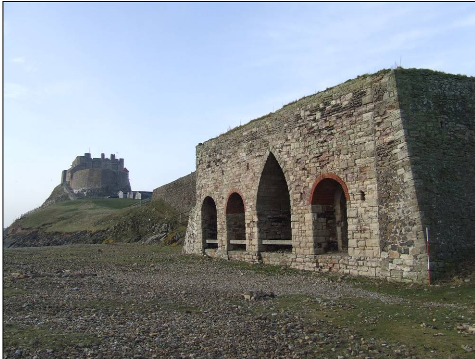
Fig 5.14.11 The impressive Lime Kilns (403) below Lindisfarne Castle
