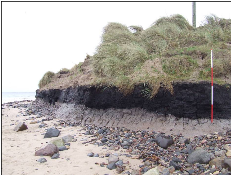
Fig. 6.1 A band of exposed peat in the eroding cliff section at Low Hauxley, Northumberland, at low tide. Wave action is currently undercutting the soft cliff sediment (till) resulting in the collapse of the peat layers and dune sand above. Material is lost on most tides.
