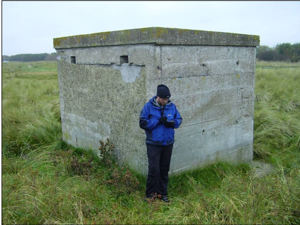
Fig 5.8.10 One of the observation posts. Note the large blocked entrance and aperture at the front, distinguishing it from a pillbox.
