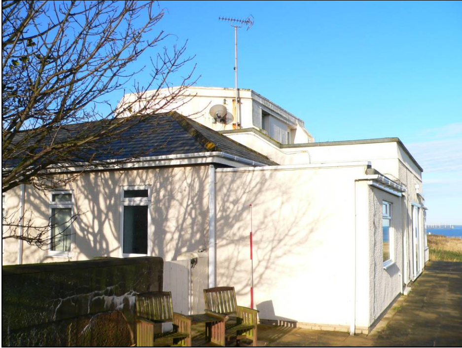
Fig 5.7.8 Exterior of Fort House looking north.
