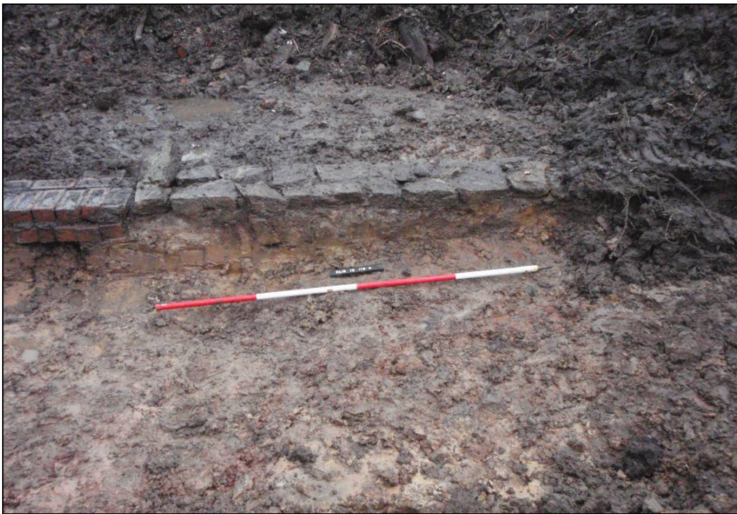
Fig. 11: South-east facing wall (114) and brick wall (113) laid onto natural ground. Facing north-west. Scale 2m
