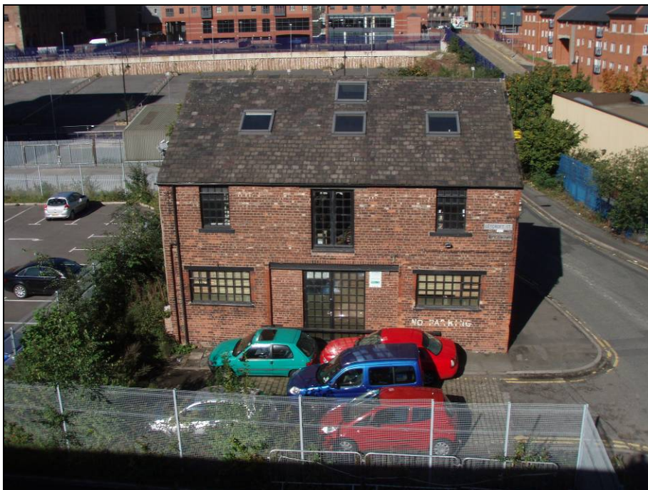
Fig 11 View looking north, showing the only surviving building in proximity to the development that predates the car park, now used as offices.
