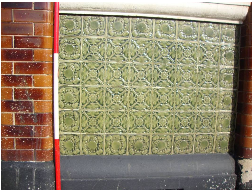
Fig. 60. Glazed bricks and Tiles
