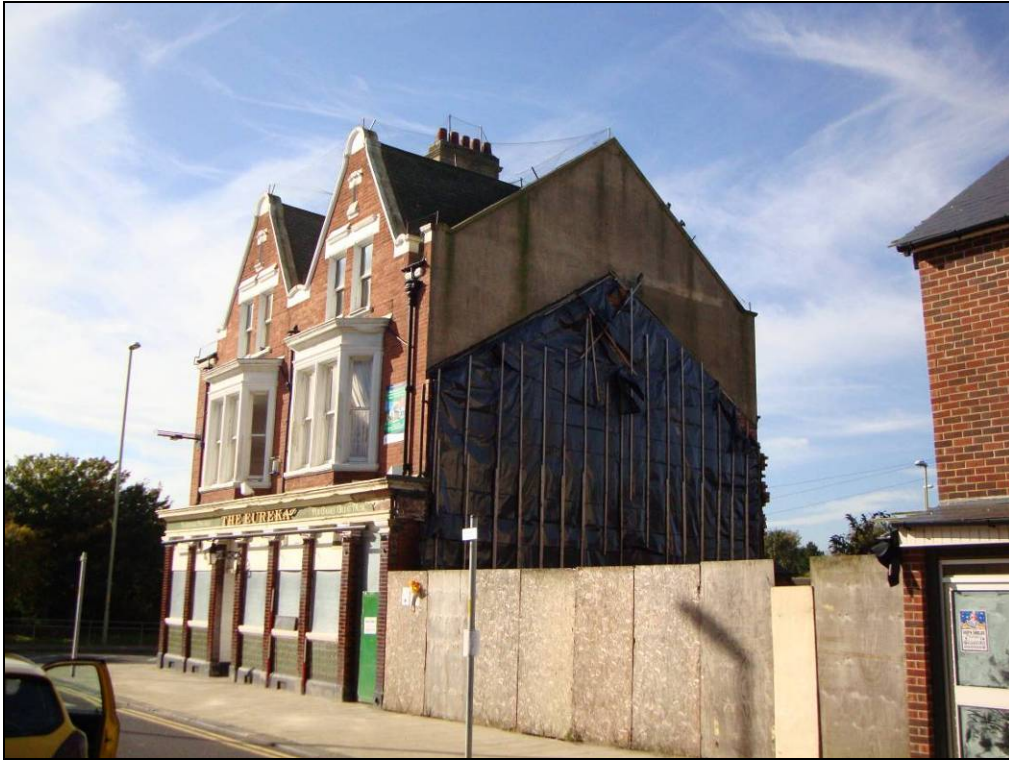
Fig. 55. Northeast facing elevation
