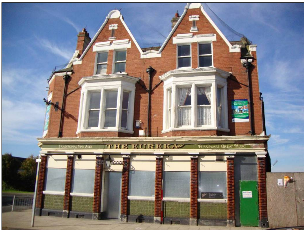
Fig. 54. Southeast facing elevation
