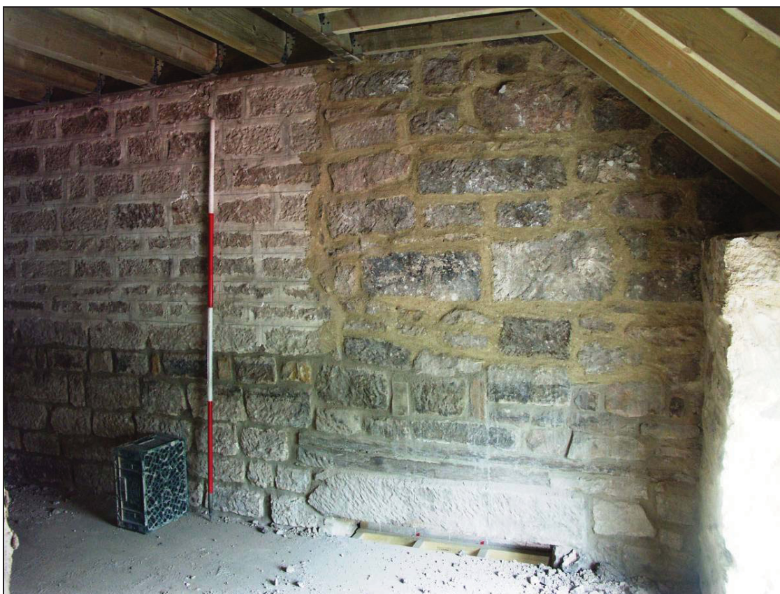
Figure 32: Room S-6, looking east (scale 2m)
