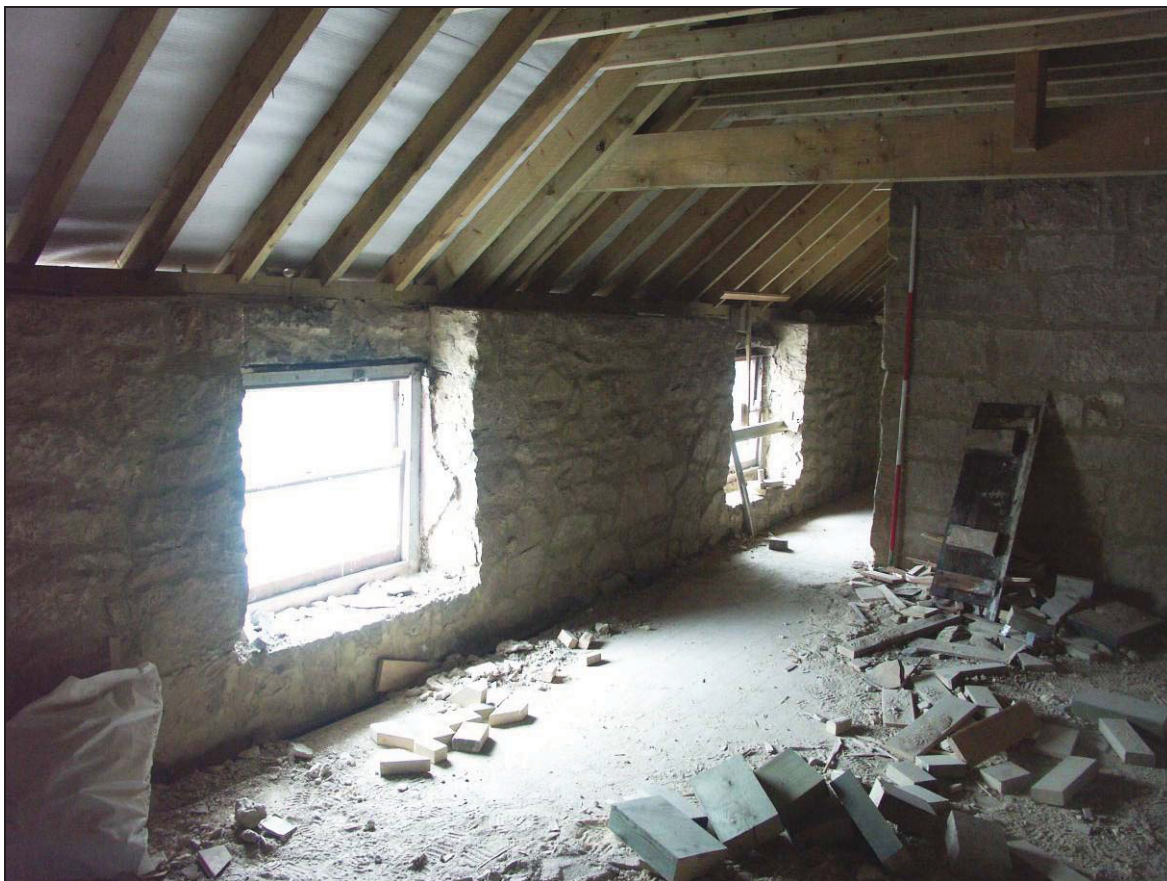
Figure 33: Room S-7, looking east (scale 2m)
