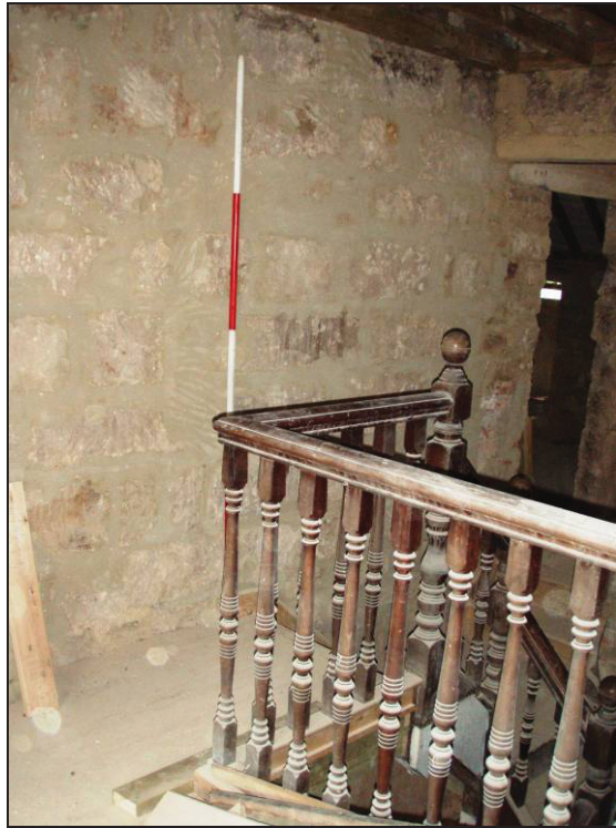
Figure 26: Top of balustrade, looking north
