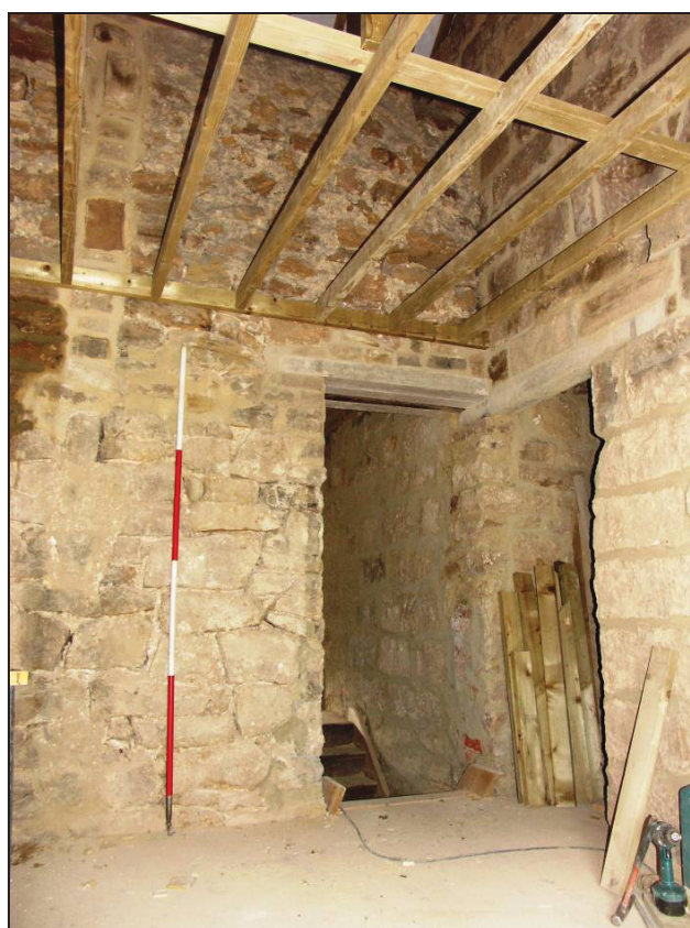
Figure 30: Room S-4, looking south (scale 2m)
