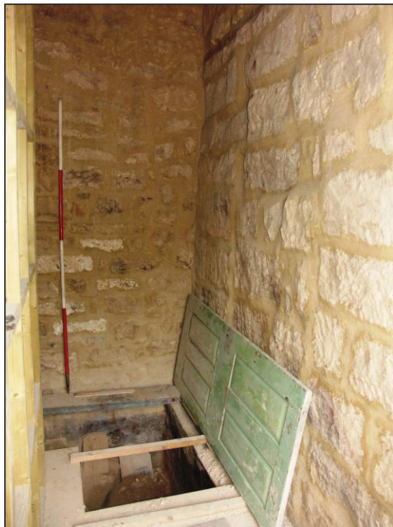
Figure 8: Hallway G-1 with stairs down to the cellar
