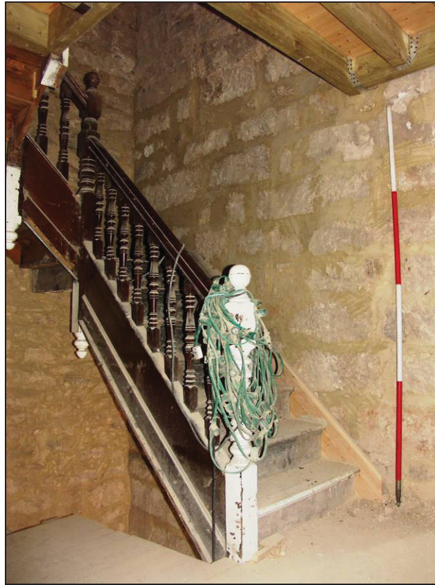
Figure 19: Staircase in hallway F-1, looking north-east (scale 2m)
