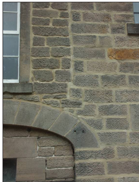
Figure 4: Detail of jagged joint above the arched head of the cart way
