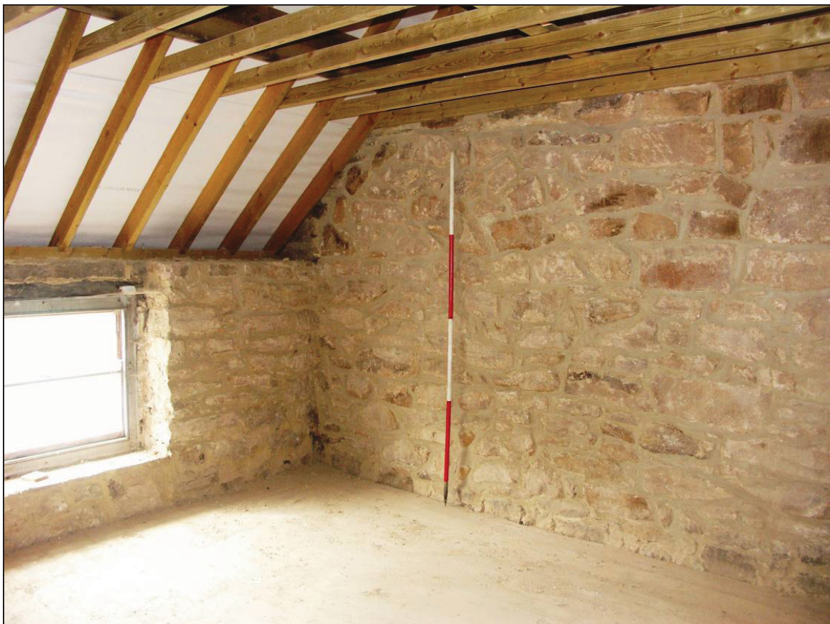
Figure 28: Room S-2, looking west (scale 2m)
