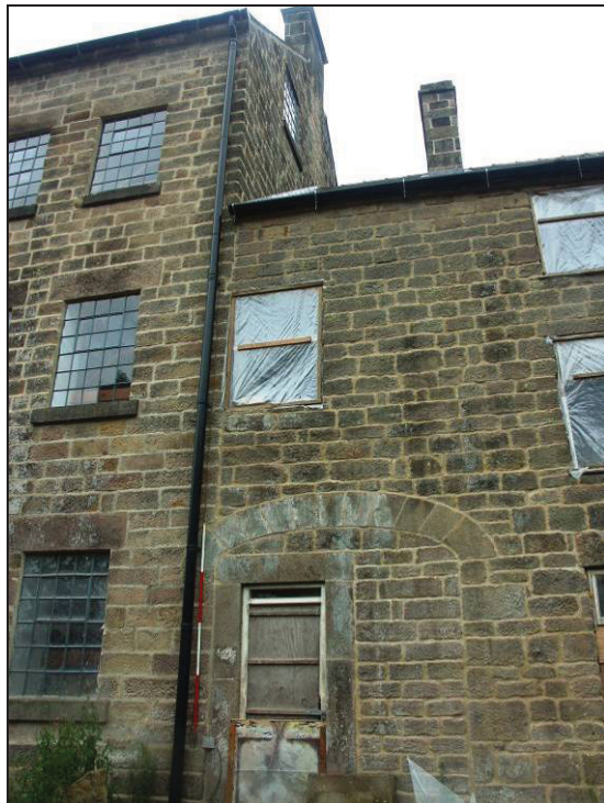
Figure 6: Joint between the house and the mill
