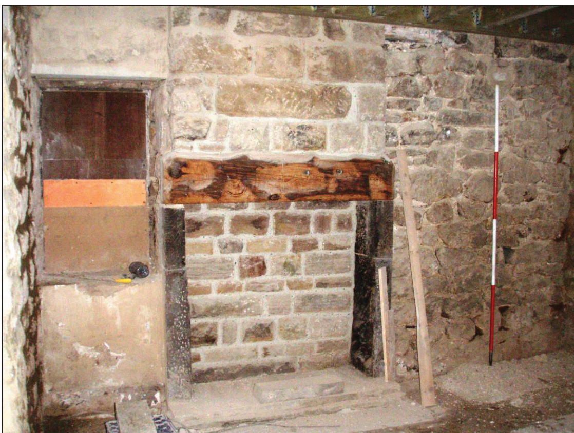
Figure 13: Fire place in room G-3, looking west (scale 2m)
