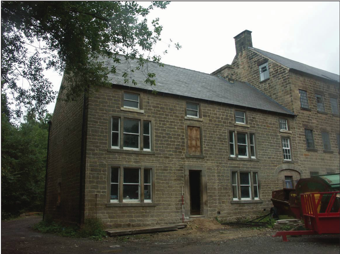
Figure 2: General view of the southern elevation (scale 2m)
