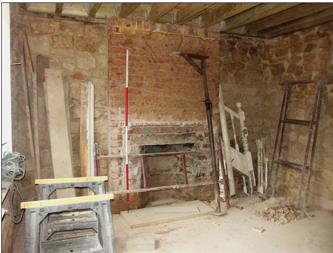
Figure 11: Fire place in room G-2, looking west (scale 2m)
