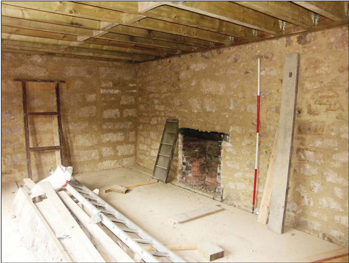
Figure 25: Fire place in room F-7, looking north-west (scale 2m)
