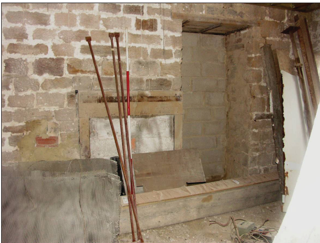
Figure 17: Blocked fire place in room G-6, looking east (scale 2m)
