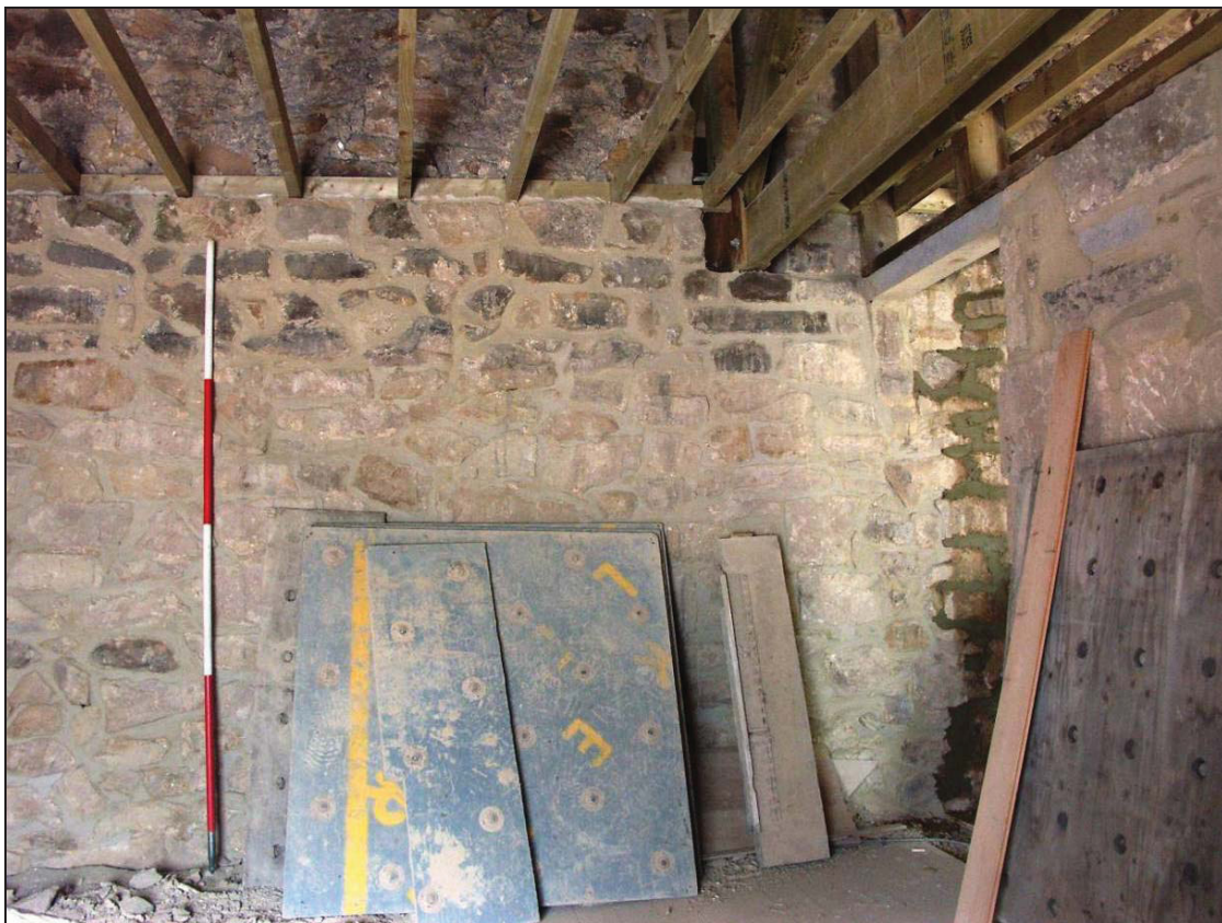
Figure 31: Room S-5, looking south (scale 2m)
