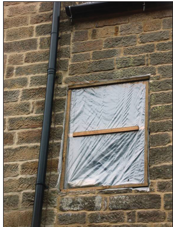
Figure 7: Detail of jagged joint on the second floor
