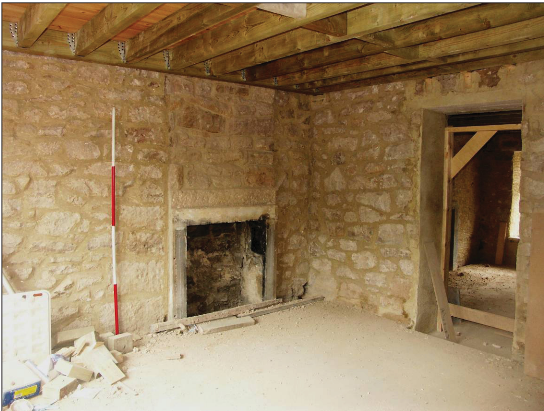
Figure 20: Fire place in room F-2, looking west (scale 2m)
