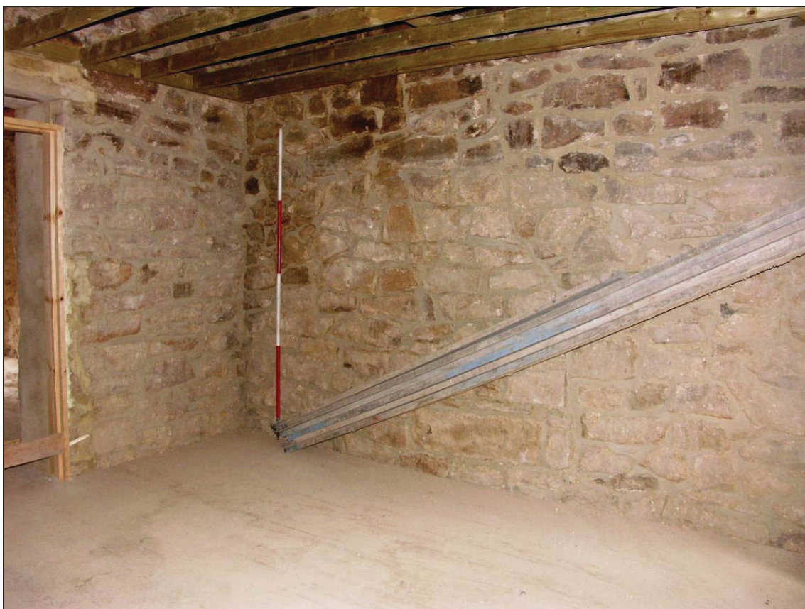
Figure 29: Room S-3, looking west (scale 2m)
