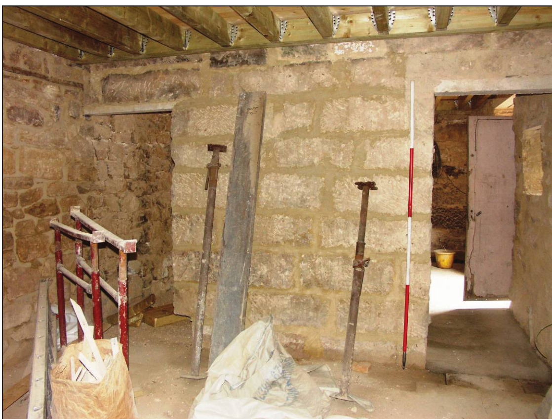
Figure 15: Room G-4, looking east (scale 2m)
