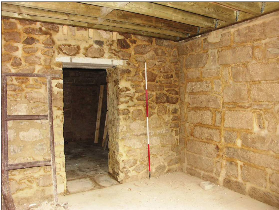
Figure 12: Room G-2, looking north (scale 2m)
