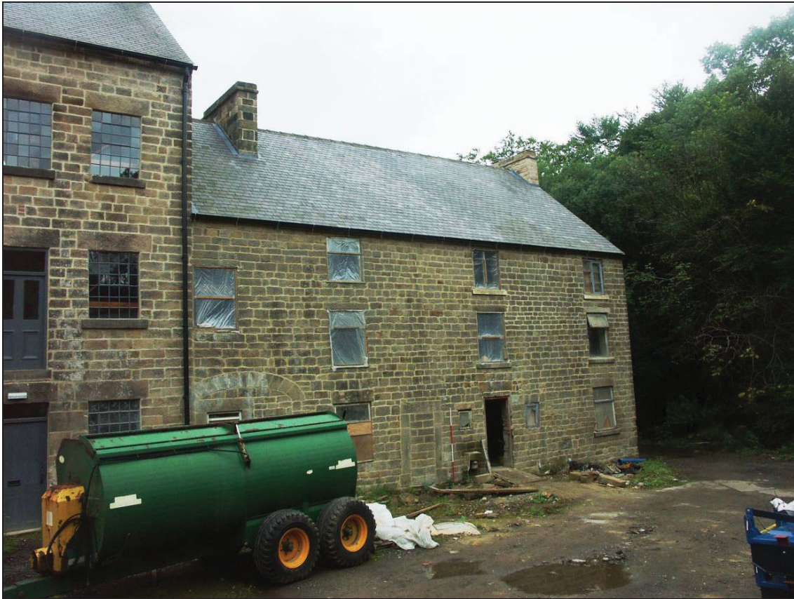
Figure 5: General view of the northern elevation (scale 2m)
