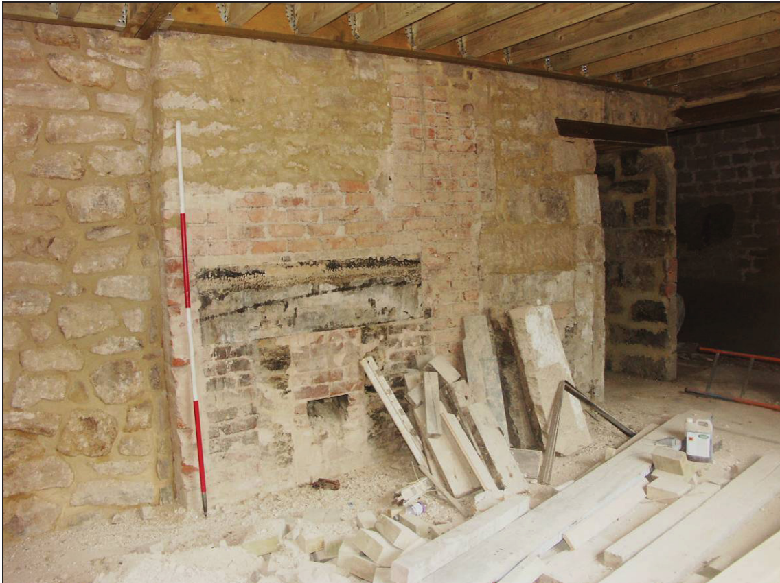
Figure 18: Blocked fire places in room G-7, looking north-east (scale 2m)
