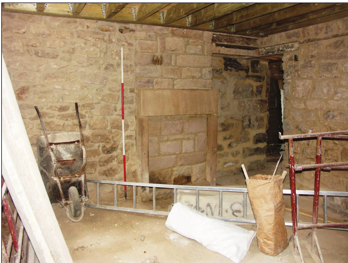
Figure 16: Blocked fire place in room G-5, looking east (scale 2m)
