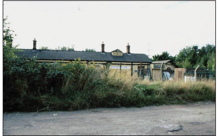
East elevation of the Central Station
