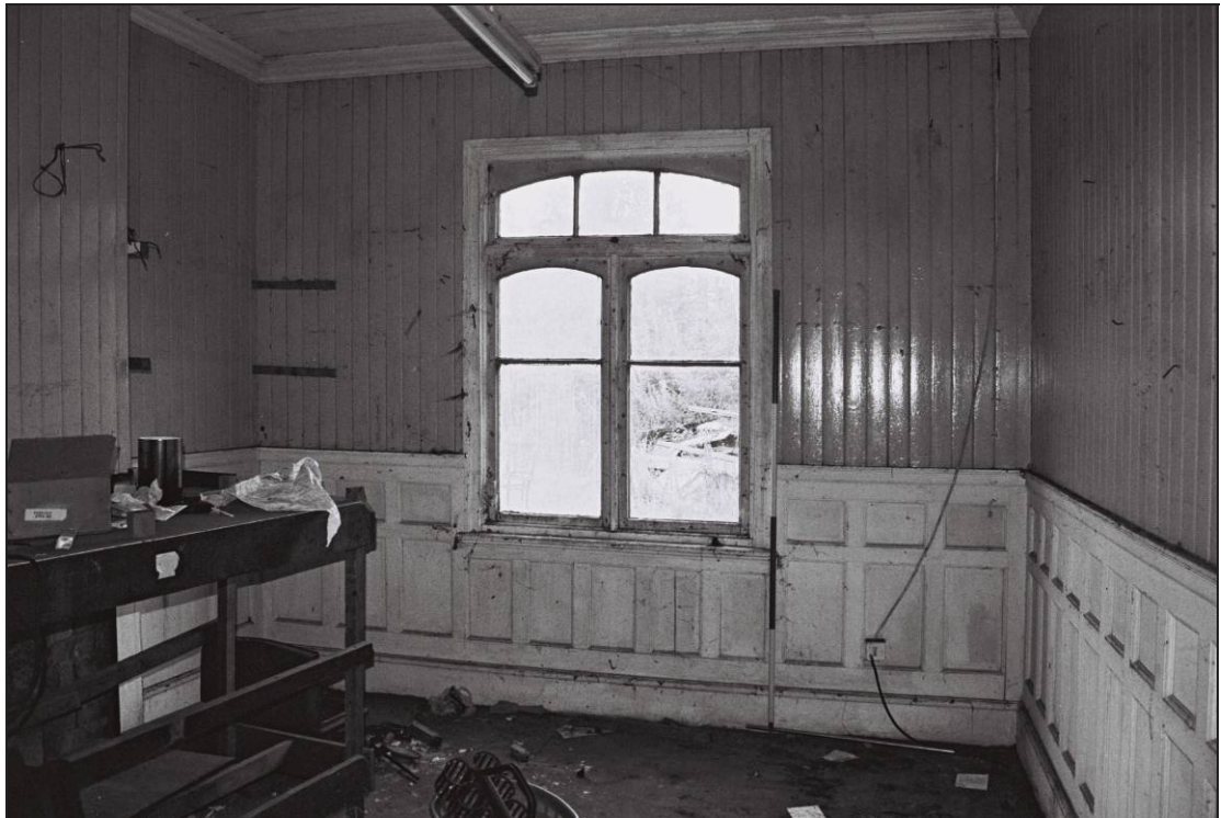
Figure 20: Room 2, looking east
