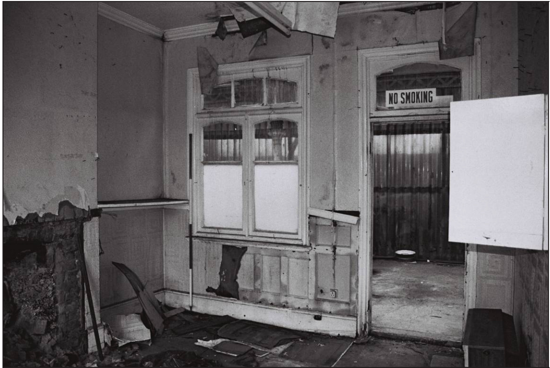
Figure 21: Room 3, looking west towards the platform
