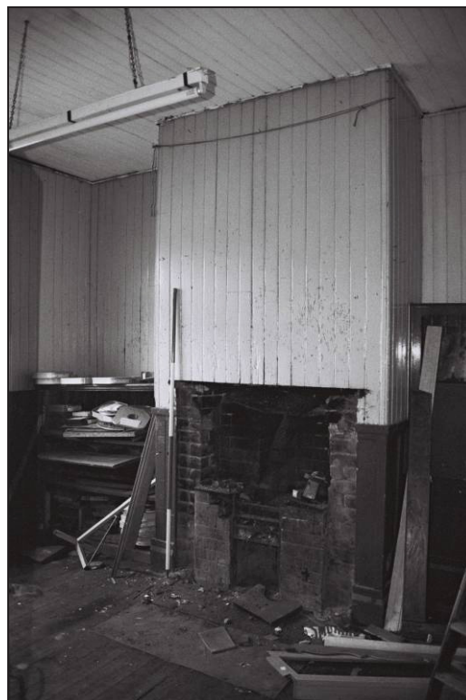
Figure 32: Fire place, looking south
