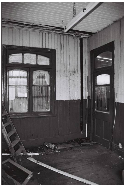
Figure 31: Room 7, looking north-west
