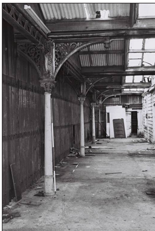
Figure 5: Canopy, looking north
