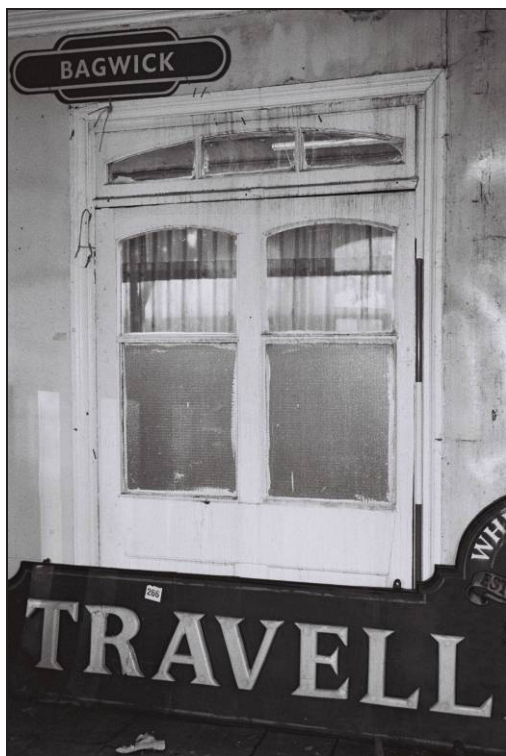
Figure 23: Example of window, looking east
