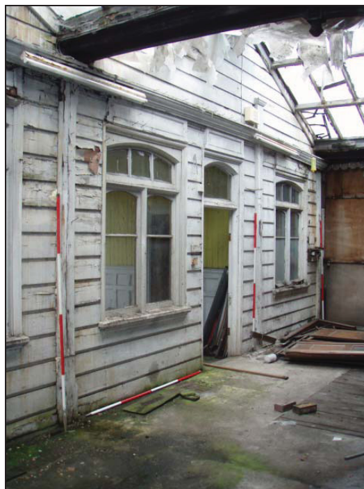
Figure 4: Glazed canopy on the southern end of the west elevation
