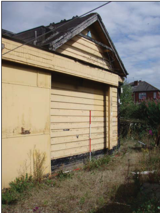
Figure 9: Southern gable wall
