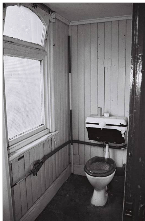
Figure 34: Toilet inside north-east partition
