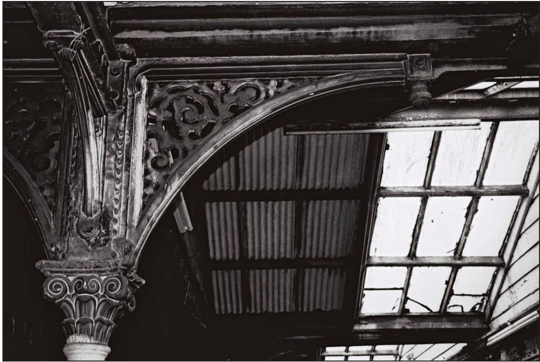
Figure 7: Detail of capital and braces
