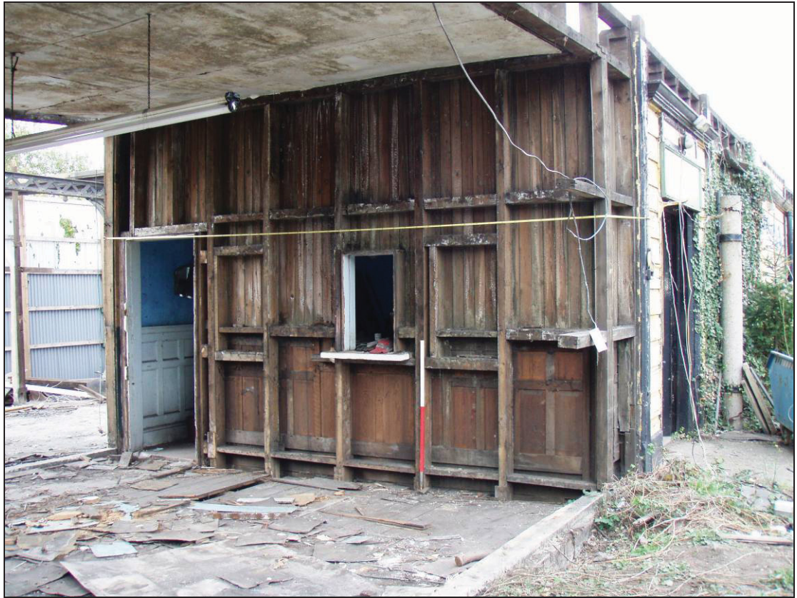
Figure 25: Timber frame of the Tickets Office after wall panel's dismantlement
