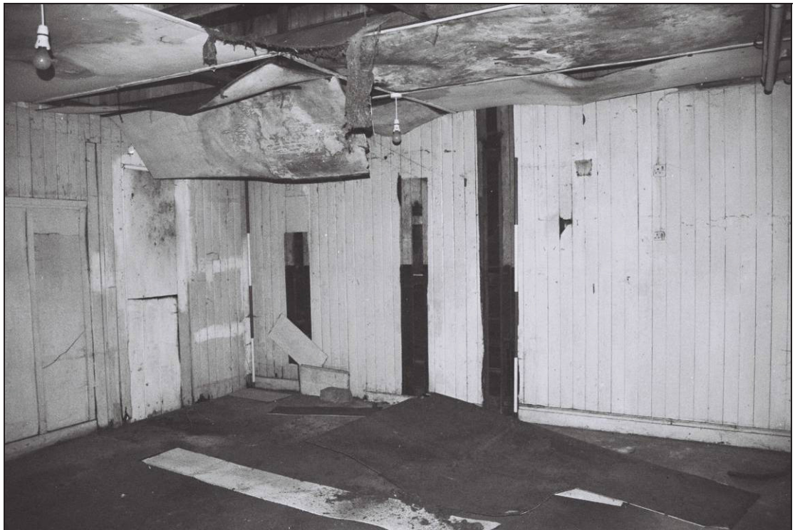
Figure 29: Room 6, looking north-east
