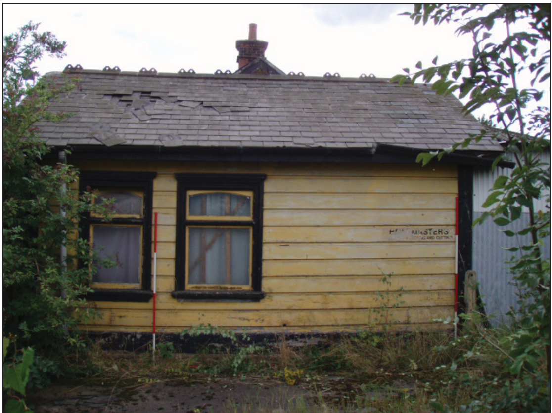
Figure 14: North side wall of the northern wing
