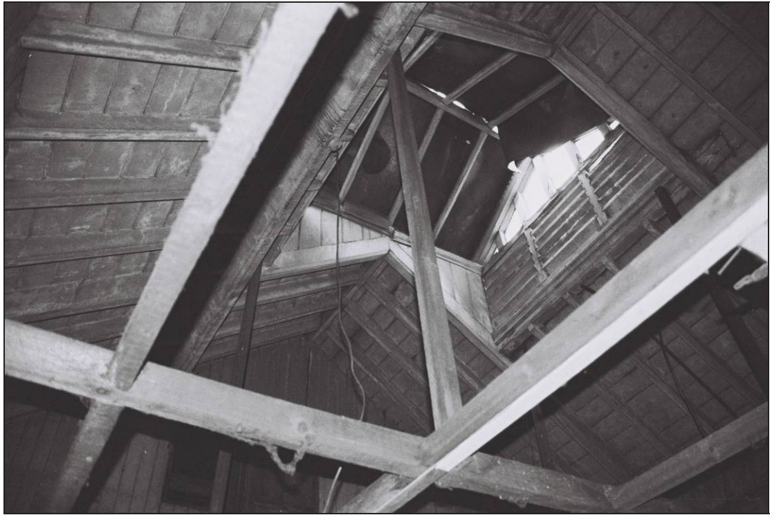
Figure 30: Louvre lantern in Room 6
