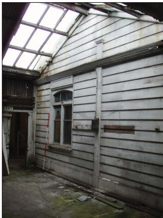
Figure 3: Glazed canopy on the northern end of the west elevation
