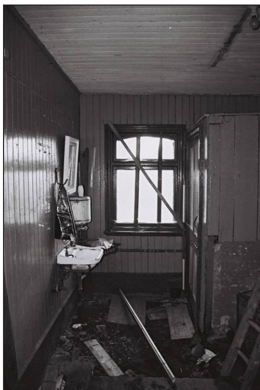
Figure 33: Gents Lavatory, looking north
