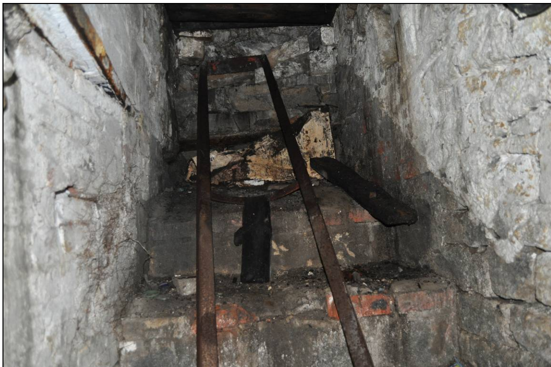
Figure 87. Cellar barrel chute
