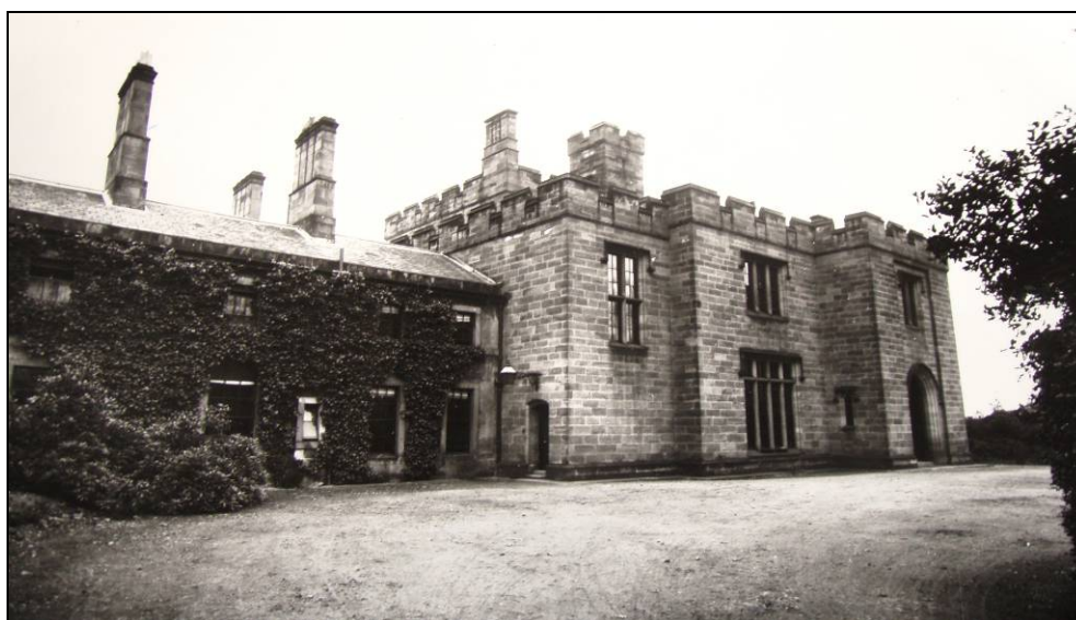
Figure 10. Southwest facing elevation of Benwell Tower dated c1900
