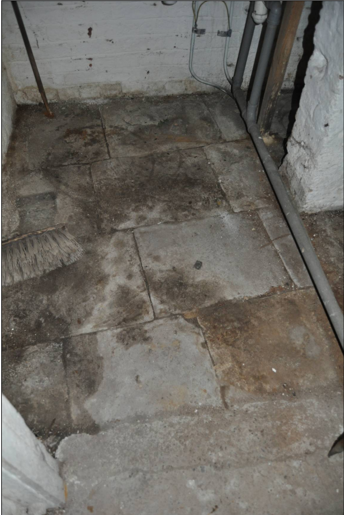
Figure 86. Cellar flag flooring
