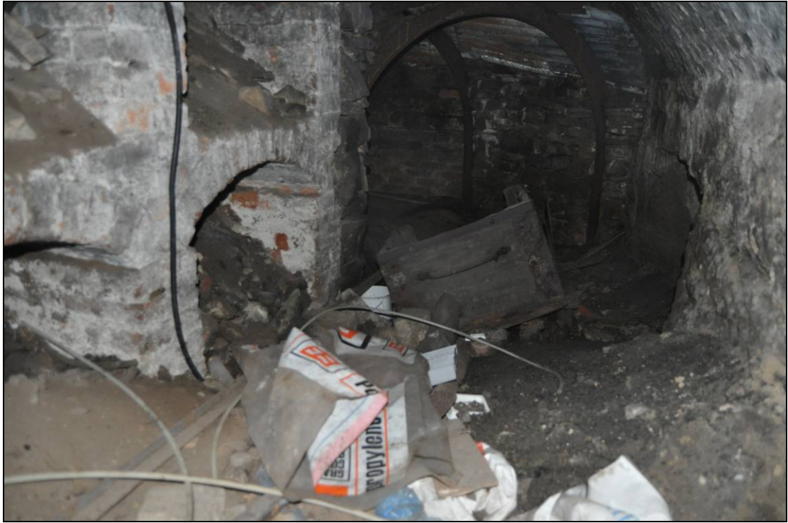
Figure 84. Cellar Tunnel with cart.
