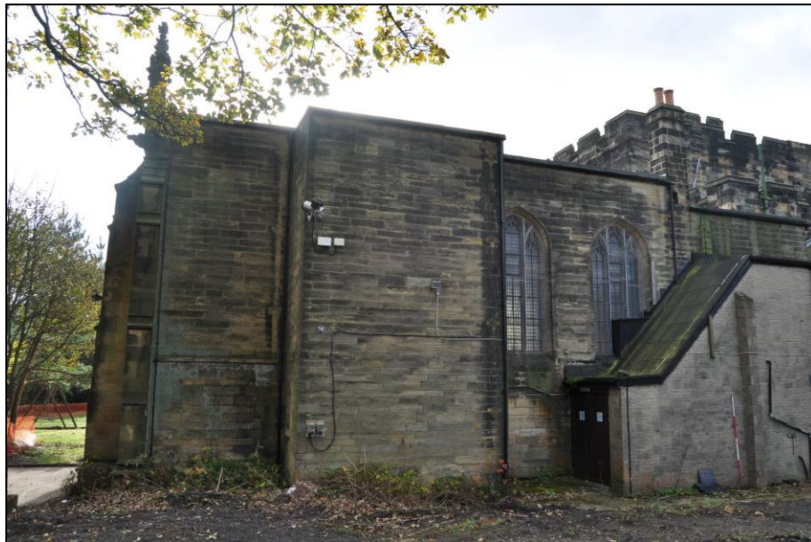
Figure 28. Chapel, north facing elevation
