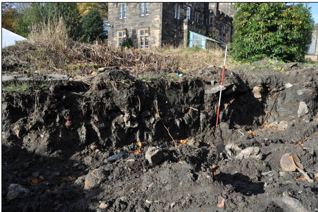
Figure 90. Excavation showing backfill layer
