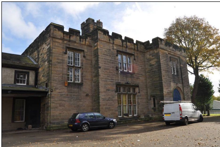
Figure 24. Southwest facing elevation
