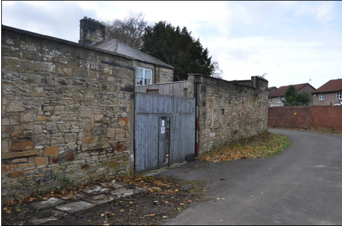
Figure 34. North facing courtyard wall
