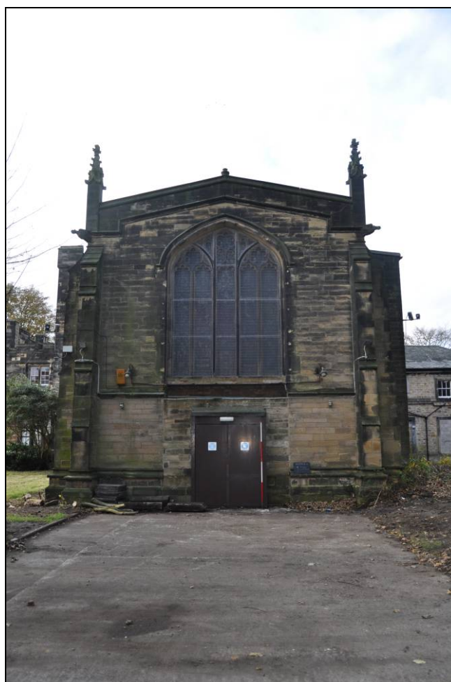
Figure 31. Chapel, northeast facing elevation
