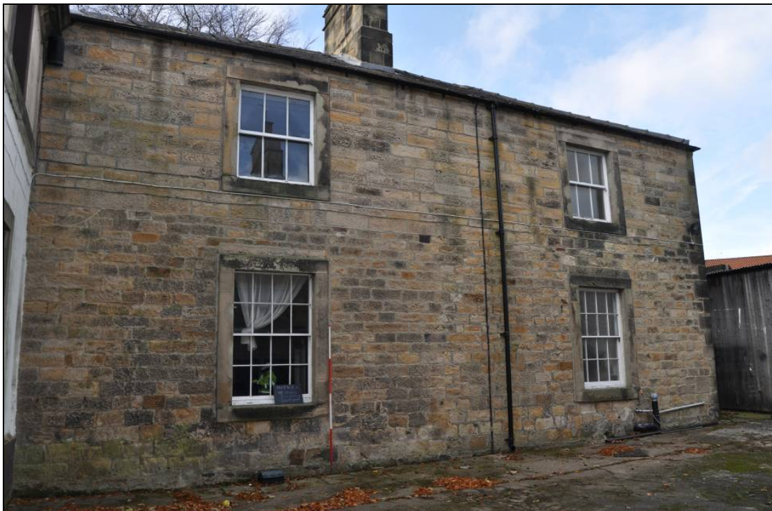
Figure 35. Courtyard, northeast facing elevation
