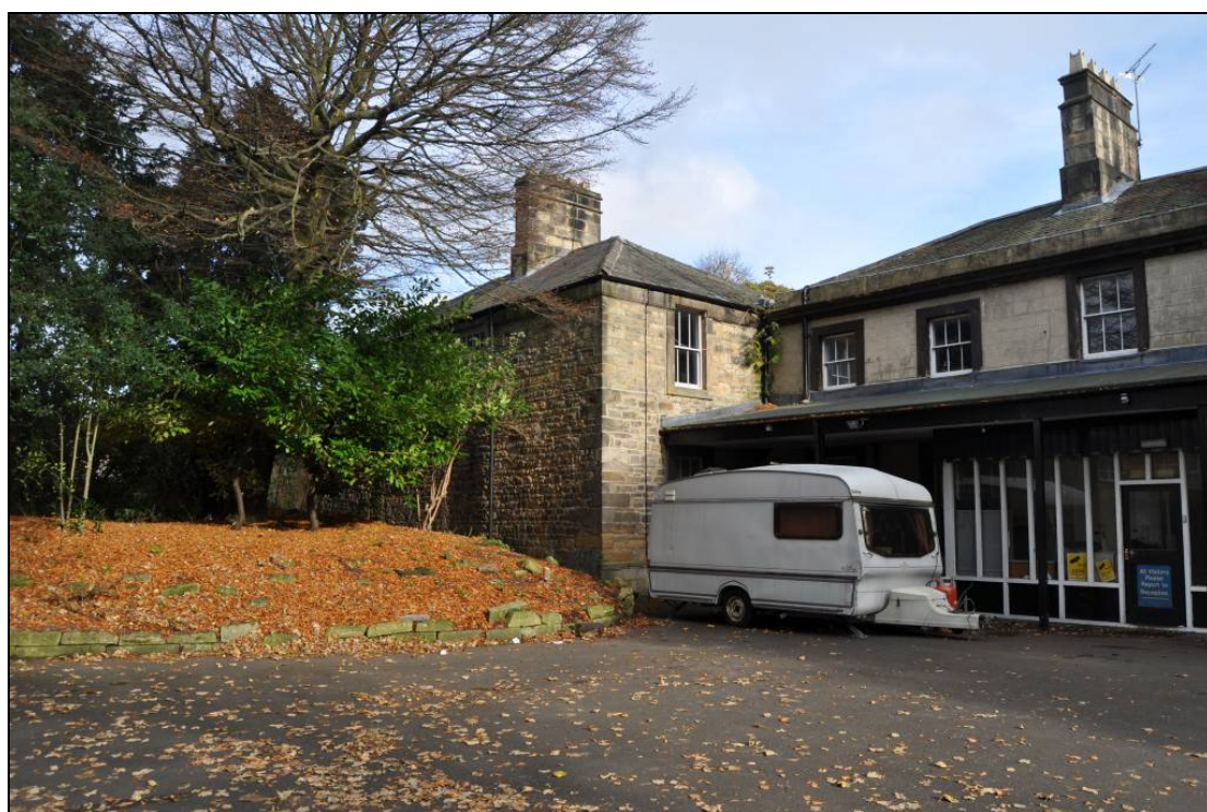
Figure 23. Southwest facing elevation
