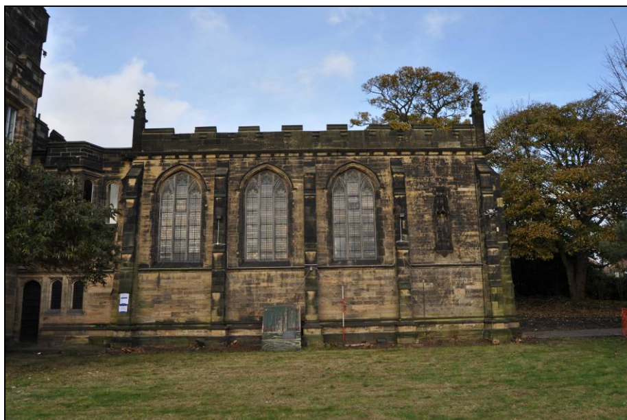
Figure 30. Chapel, south facing elevation
