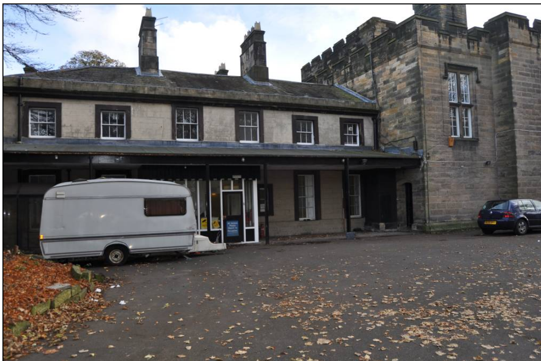
Figure 22. Southwest facing elevation
