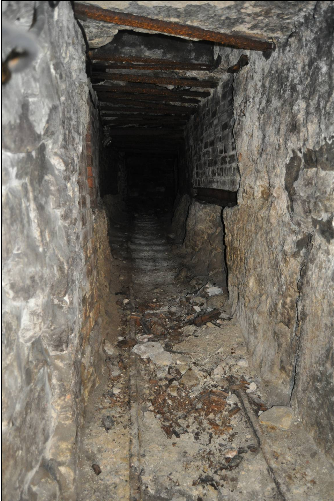
Figure 85. Cellar Tunnel showing tracks
