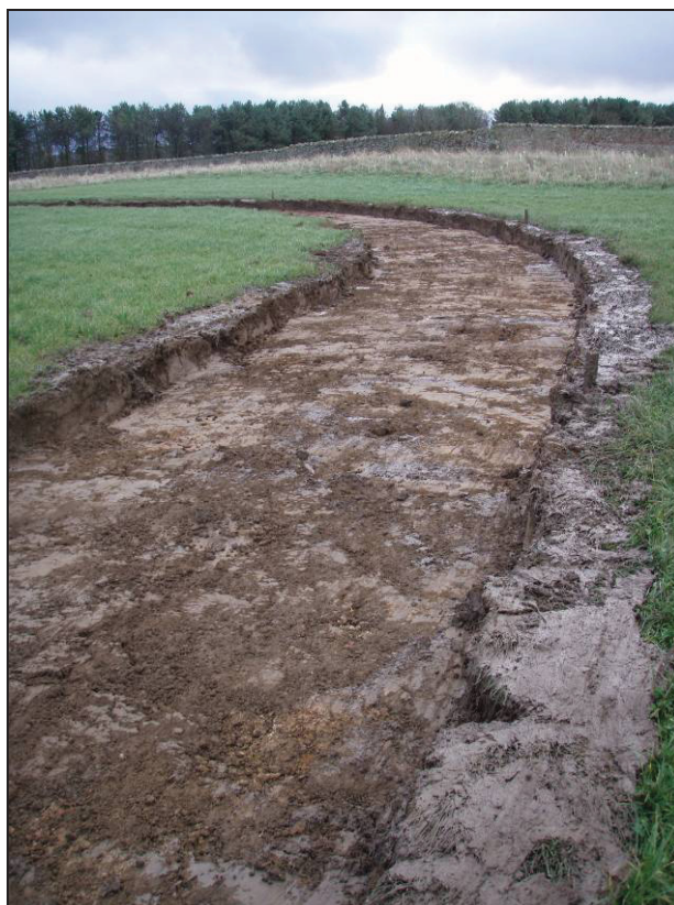
Figure 7. Excavation of new road
