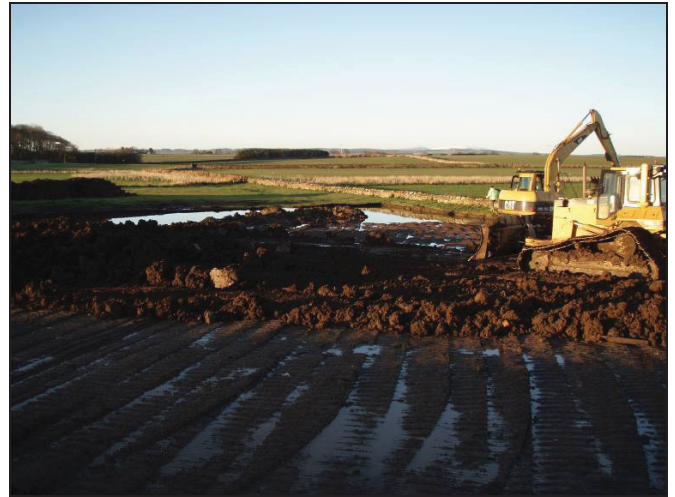
Beadnell campsite excavations
