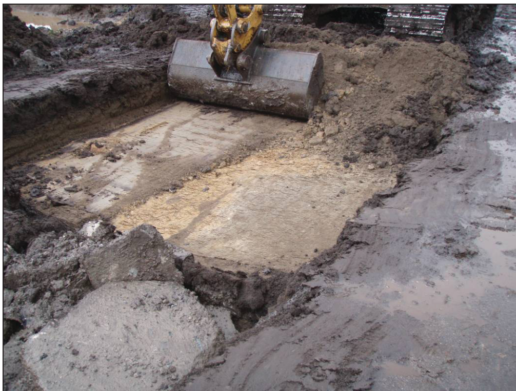
Figure 6. Excavation of hard standings
