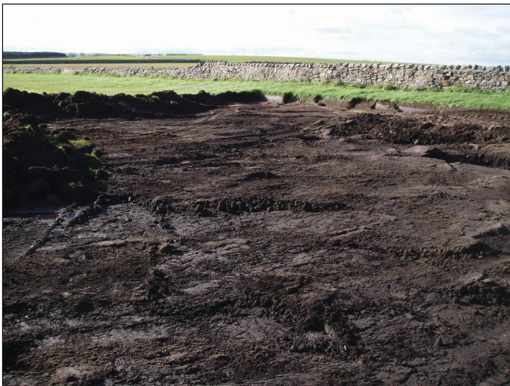
Figure 4. Levelling of site looking southwest
