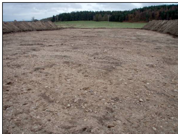
View across the stripped area at Cloddach Quarry
